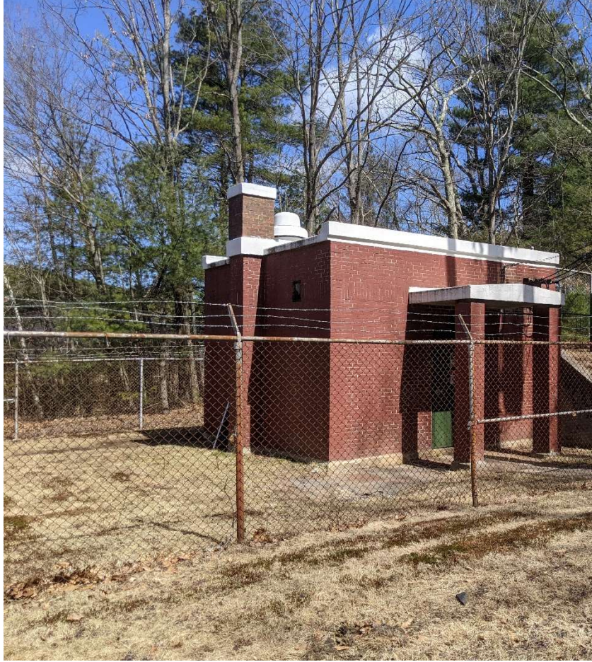
Well Station 3 Exterior – Maximum height 20 feet above ground
