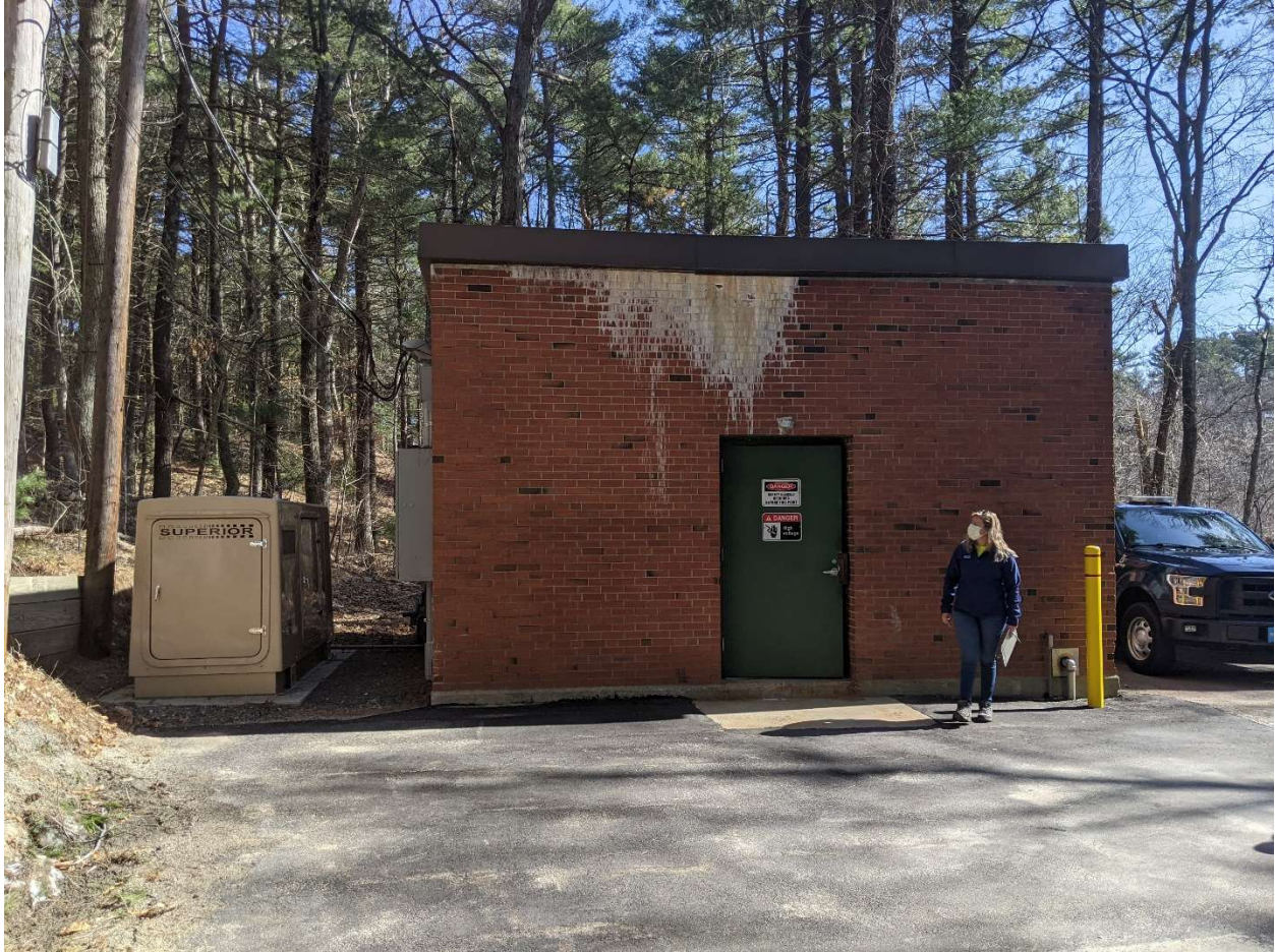
Well Station 4 Exterior (Prior to Installation of Temporary PFAS Treatment) – Maximum height 20 feet above ground
