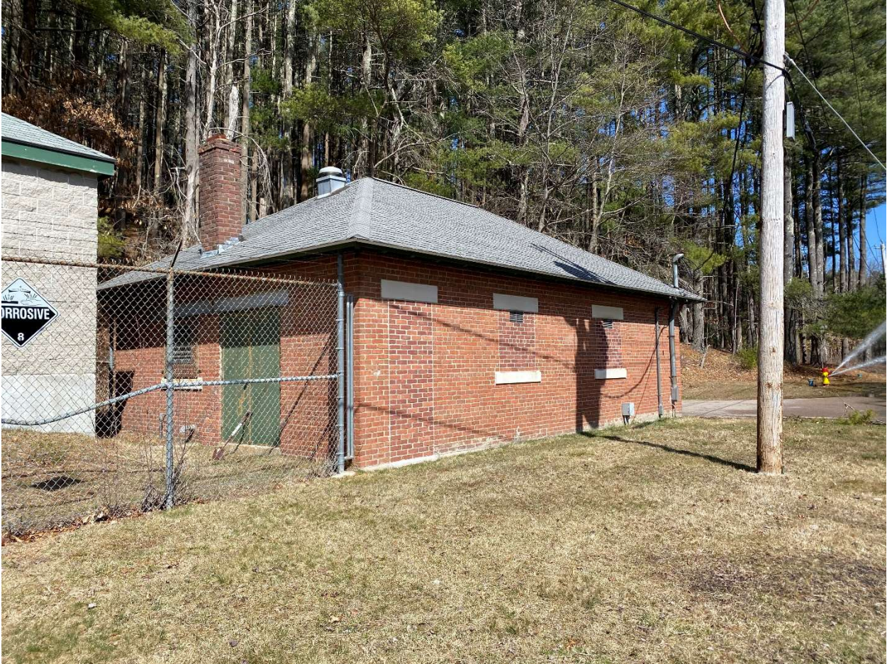
Well Station 2 Exterior – Maximum height 20 feet above ground
