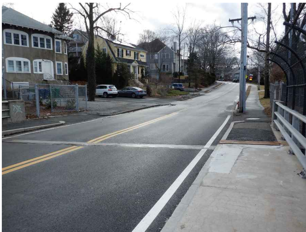
Photo 4: South approach from bridge, looking south.
