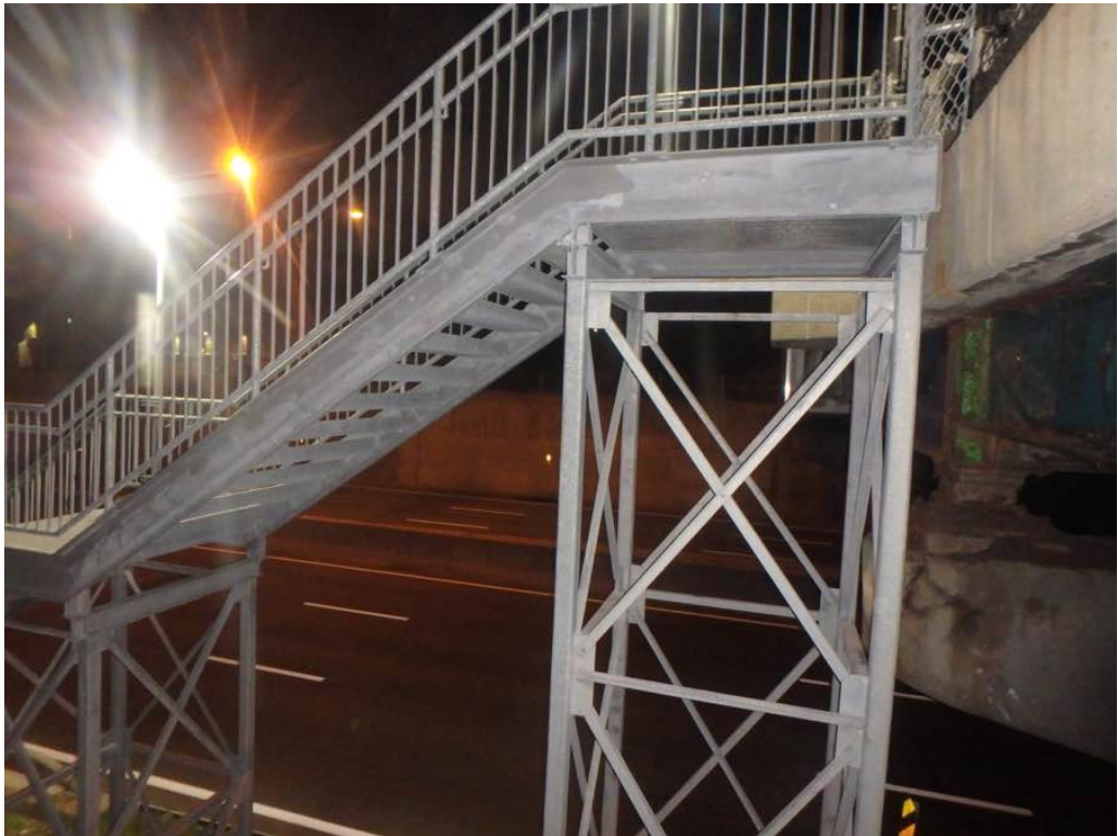
Photo 15: New steel stairway mounted to east fascia in span #3
