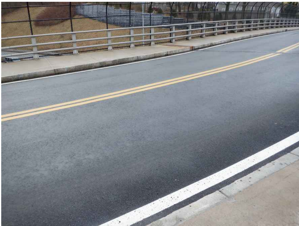
Photo 8: Wearing surface, span 1 shown, looking southeast - repaved since the previous inspection.
