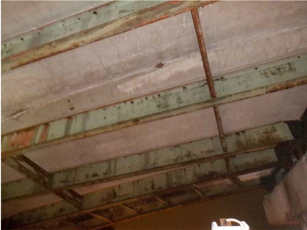
Photo 1: Underside of superstructure, span 1 shown, looking east.
