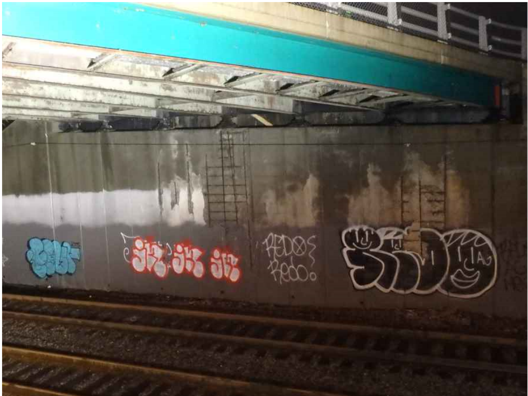
Photo 16: North abutment breastwall - note areas with large spalls with exposed and debonded rebar.
