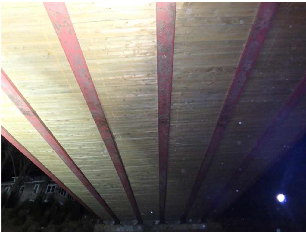
Photo 7: Underside of superstructure and timber shielding, span 3 shown, looking south.
