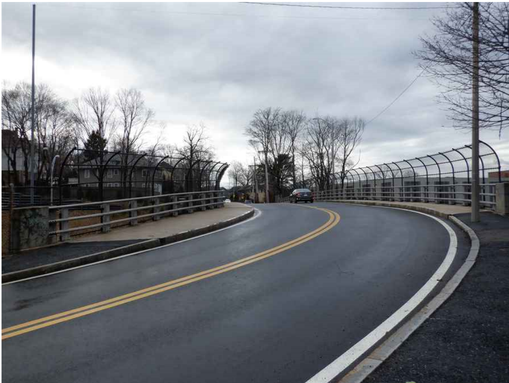
Photo 6: Bridge from north approach, looking south.
