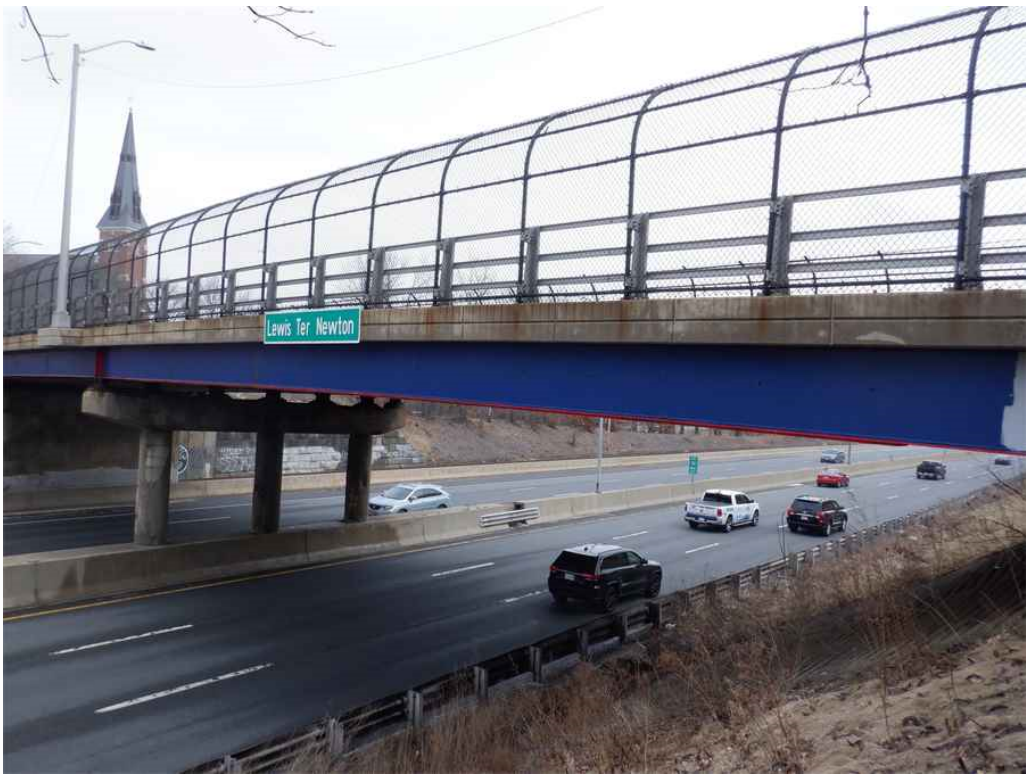
Photo 1: West elevation, looking northeast.
