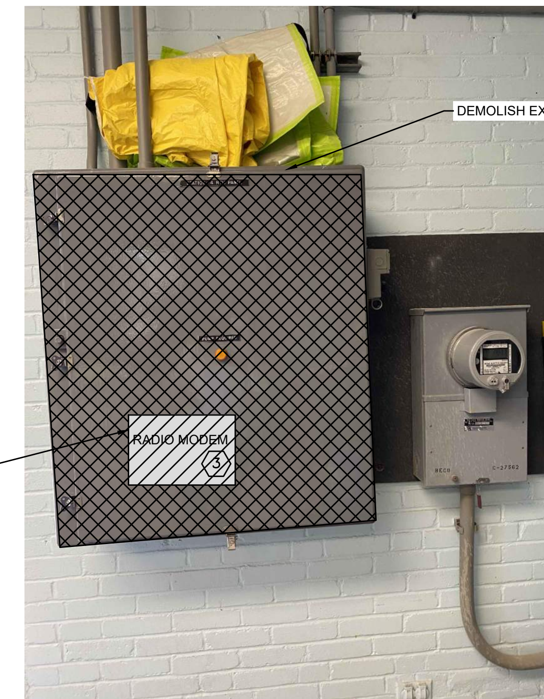
PICTURE 2 (P2) - WELL STATION 4 DEMOLITION
