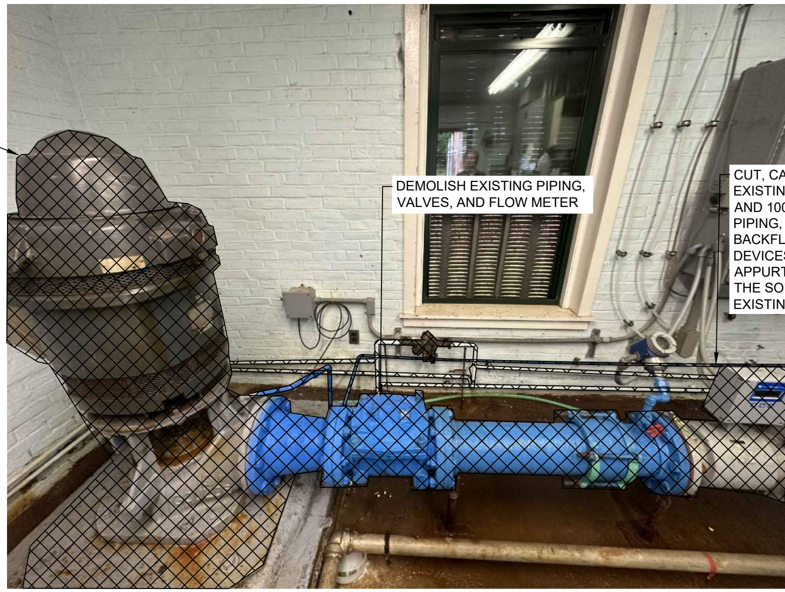
PICTURE 1 (P1) - WELL STATION 3 DEMOLITION SCALE: N.T.S.
