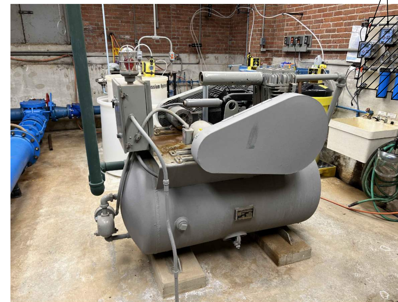
PICTURE 4 (P4) - WELL STATION 2 DEMOLITION
