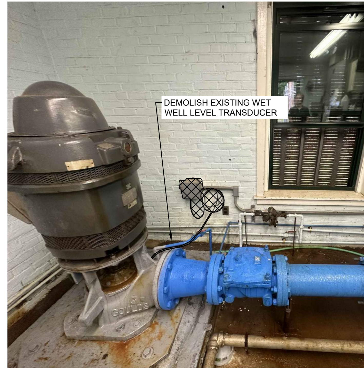
PICTURE 1 (P1) - WELL STATION 3 DEMOLITION
