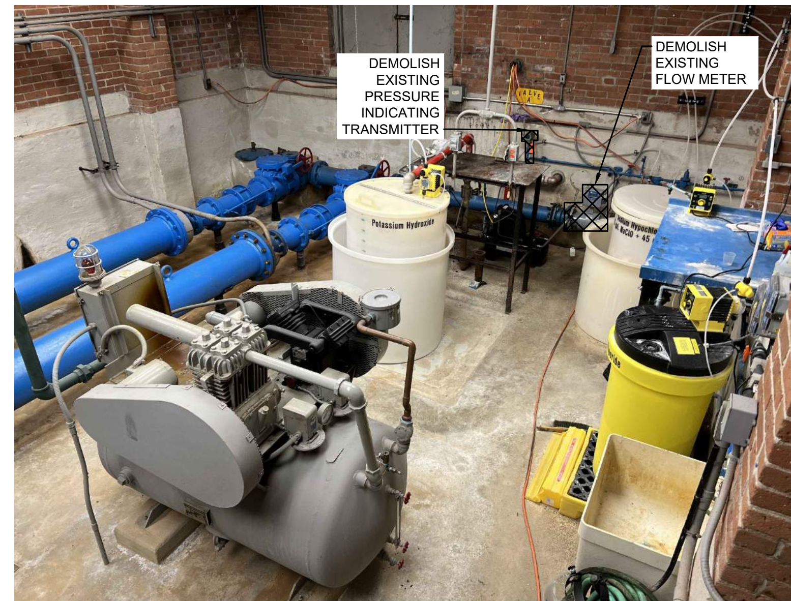
PICTURE 3 (P3) - WELL STATION 2 DEMOLITION
