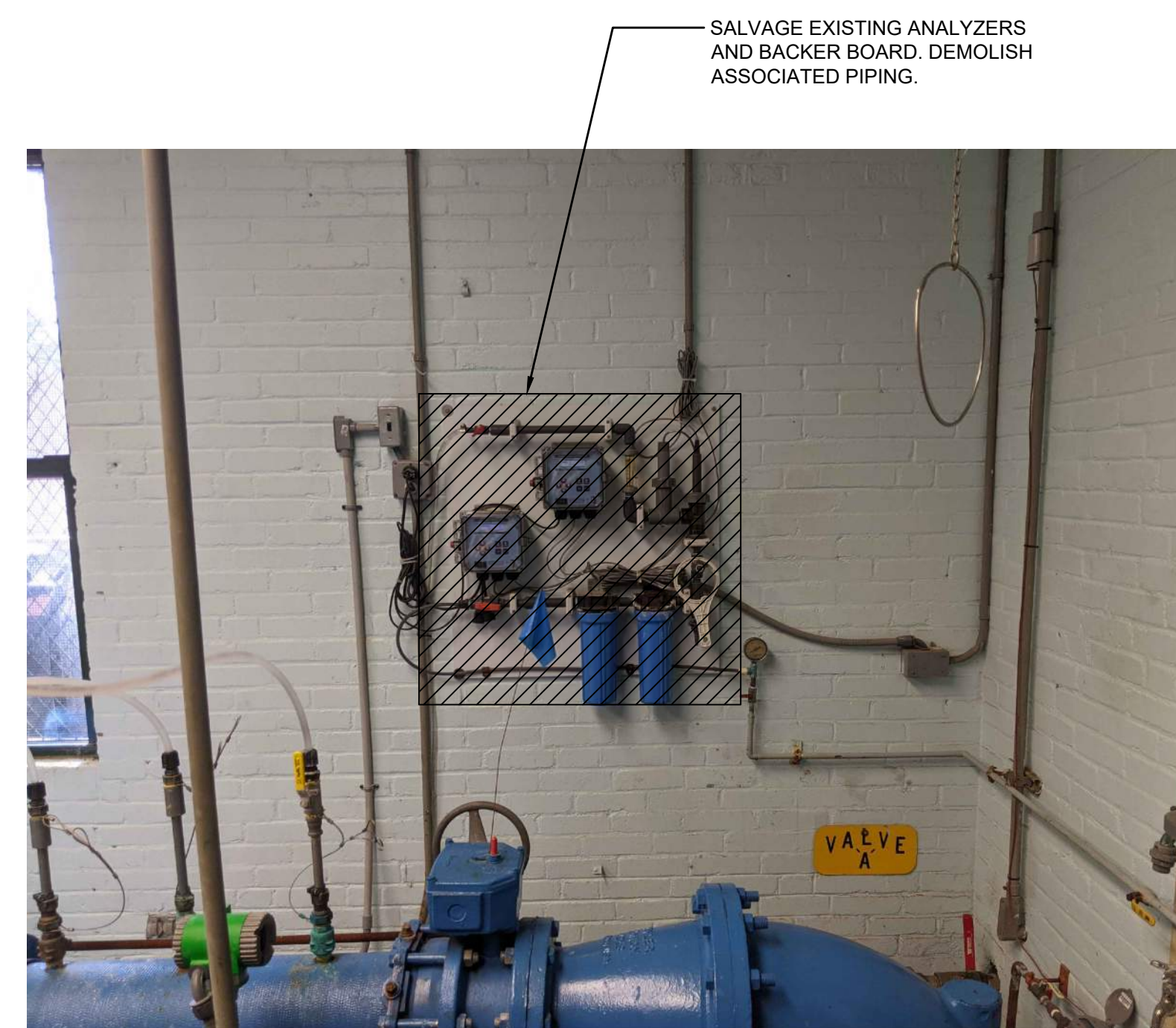
PICTURE 3 (P3) - WELL STATION 4 DEMOLITION
