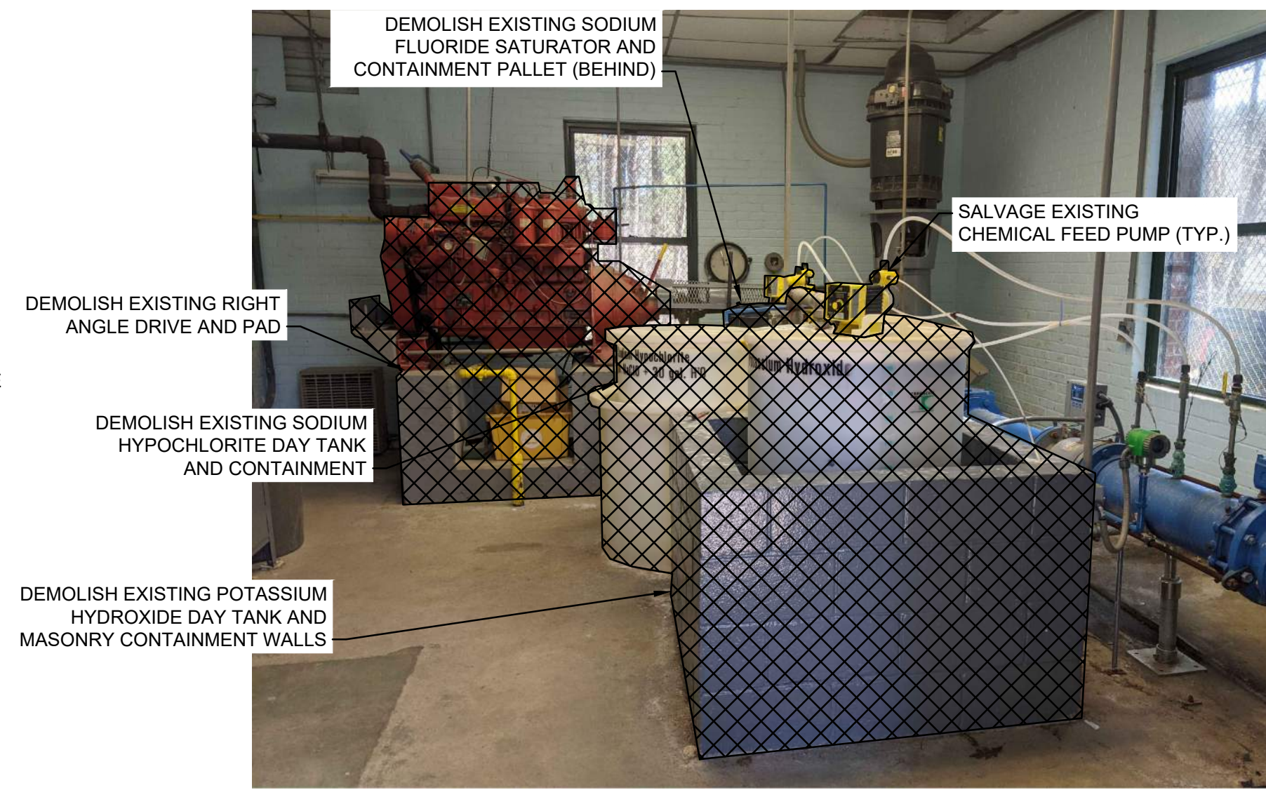
PICTURE 1 (P1) - WELL STATION 4 DEMOLITION
