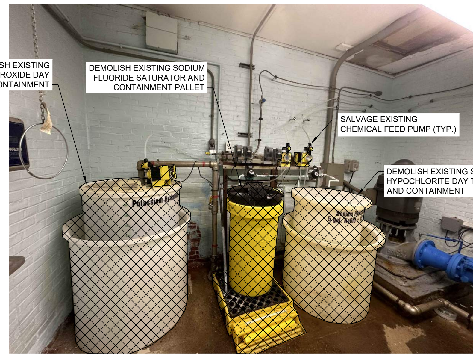
PICTURE 3 (P3) - WELL STATION 3 DEMOLITION SCALE: N.T.S.
