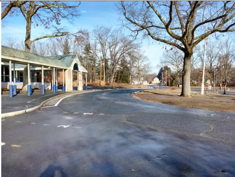
Photo #3: Entrance at the northeast corner of the school
