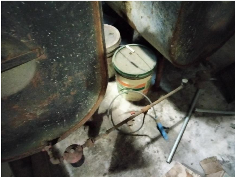
Photo #33: Two 275-gallon ASTs with fuel oil feed line
