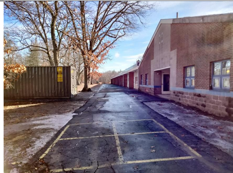
Photo #4: North side of the school
