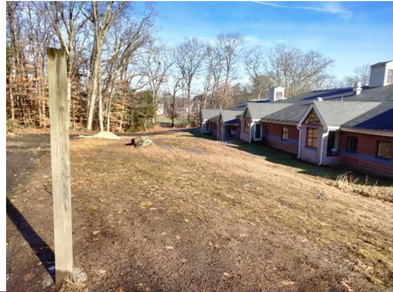
Photo #6: West side of the school
