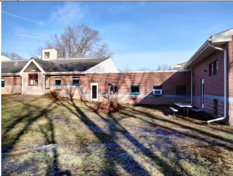
Photo #7: Southeast corner of the school looking north
