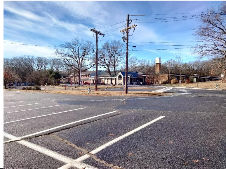
Photo #2: Green Meadow Elementary looking southwest
