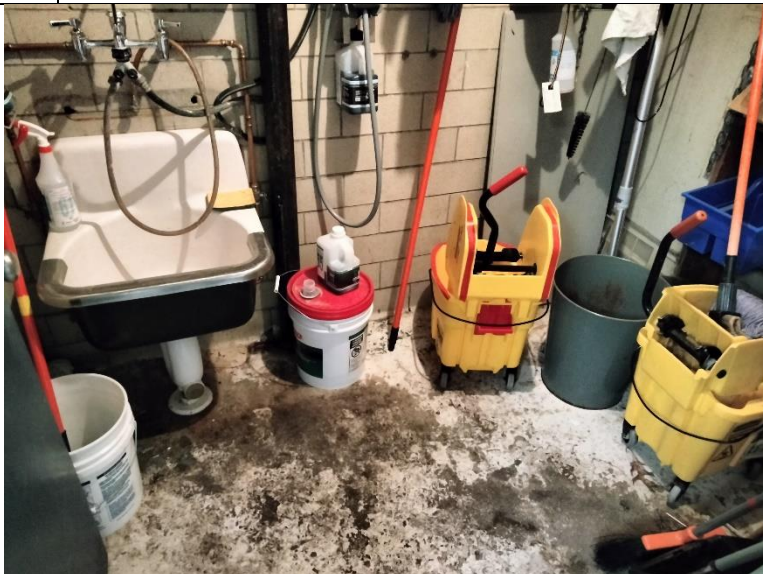
Photo #15: Maintenance closet
