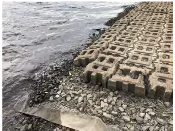
Image of edge of existing boat ramp. Low water reveals crumbling boat ramp and missing fill. Ramp presents hazard for boaters. Needs replacement or repair.
