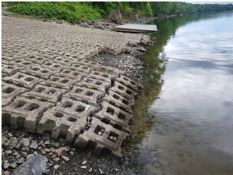
Image of edge of existing boat ramp. Low water reveals crumbling boat ramp and missing fill. Ramp presents hazard for boaters. Needs replacement or repair.
