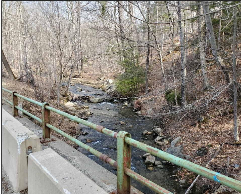
Photo 1. Potter Brook upstream from bridge View north
