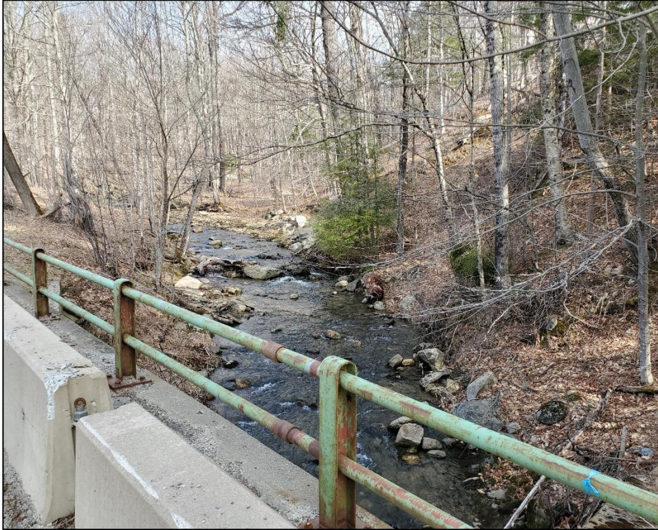
Photo 1. Potter Brook upstream from bridge View north
