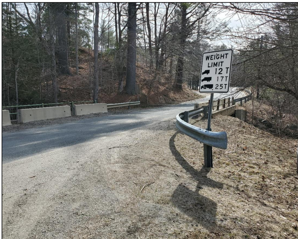
Photo 6. Bridge No. R-10-008 View northeast
