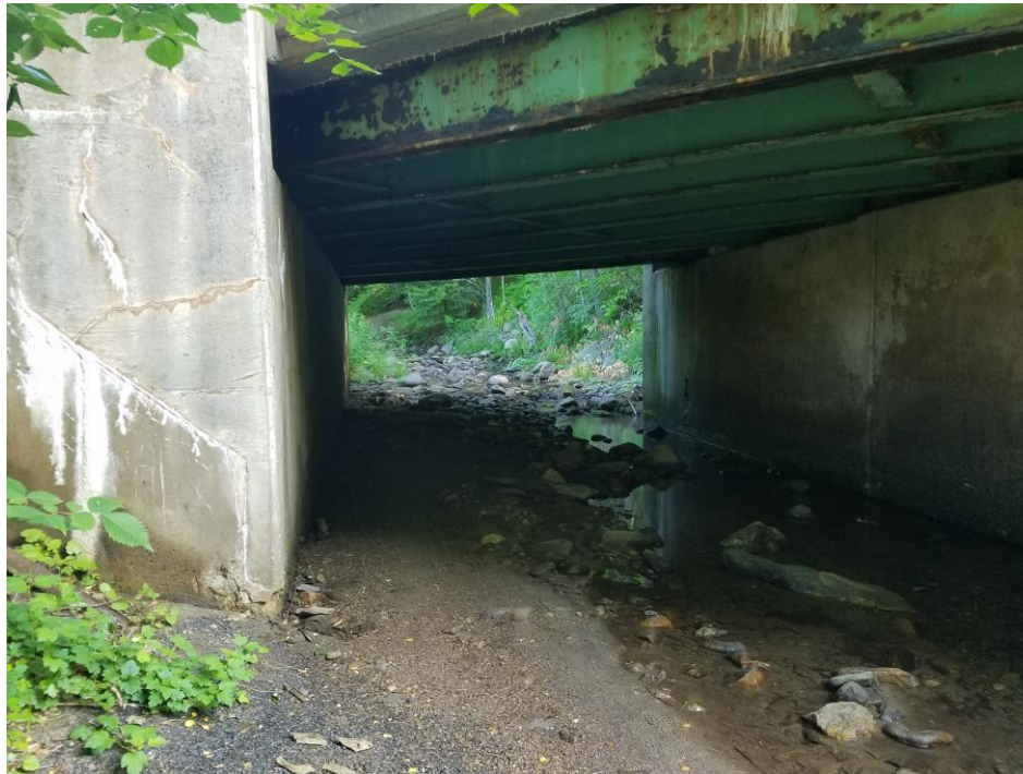
Looking north at Potter Brook beneath the Cyrus Stage Road bridge.
