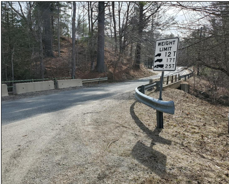
Photo 6. Bridge No. R-10-008 View northeast
