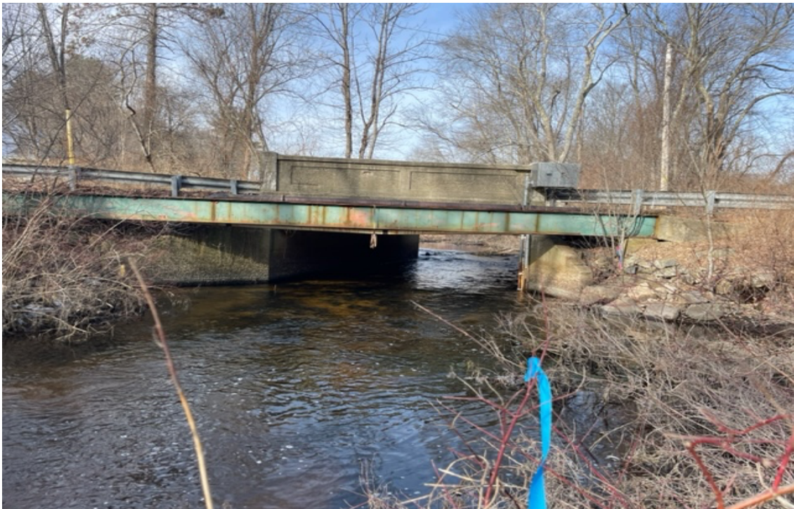
Figure 1. View of Park Road Crossing of Martin Brook.
