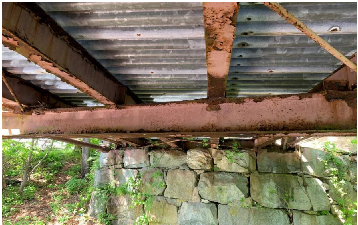
Photo 18: FB2 End Side Looking West
