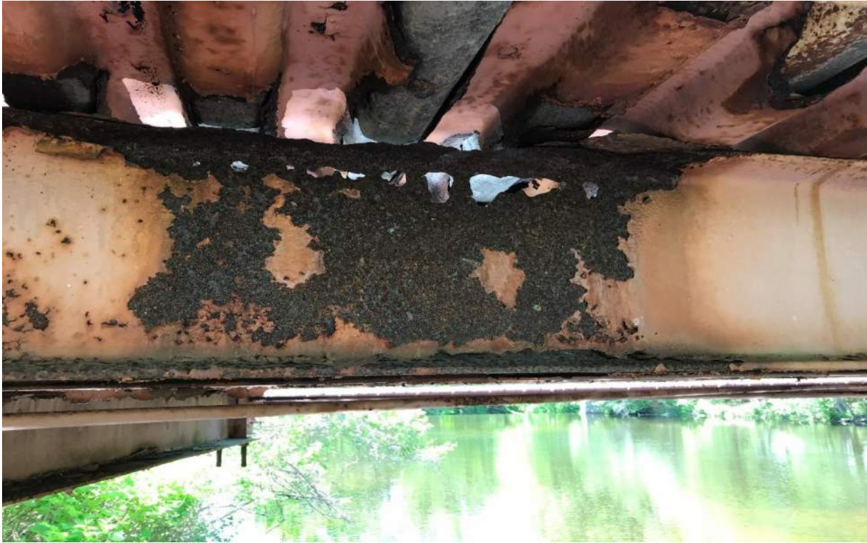
Photo 9: Panel 8 Stringer S1 Left Side Near FB8 Looking South
