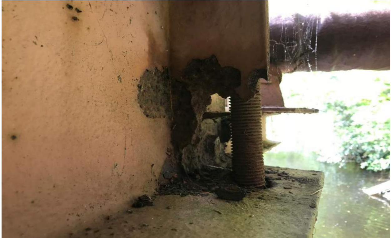
Photo 17: FB1 Right End Begin Bearing Stiffener Looking South
