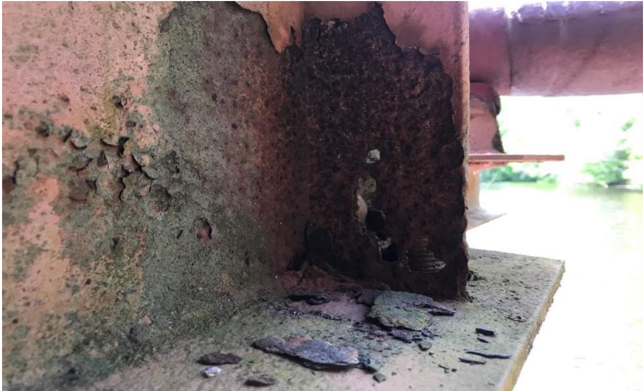
Photo 20: FB4 Right End, Begin Side Bearing Stiffener Looking South
