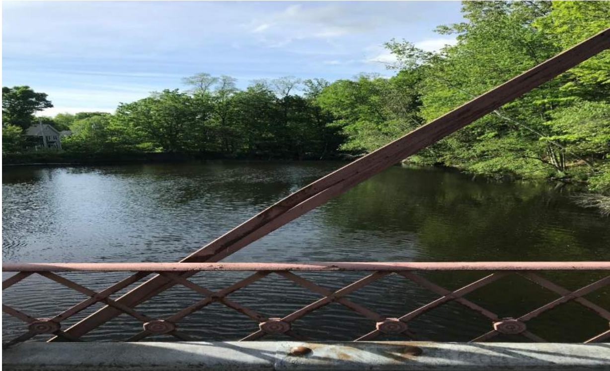
Photo 15: Right Truss Diagonal L3U2 Looking South
