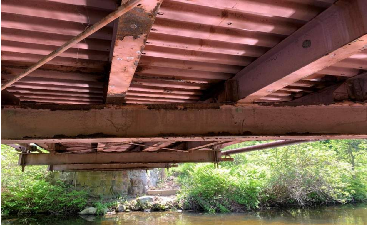
Photo 21: FB5 Begin Side Between Stringer S1 & S4 Looking East
