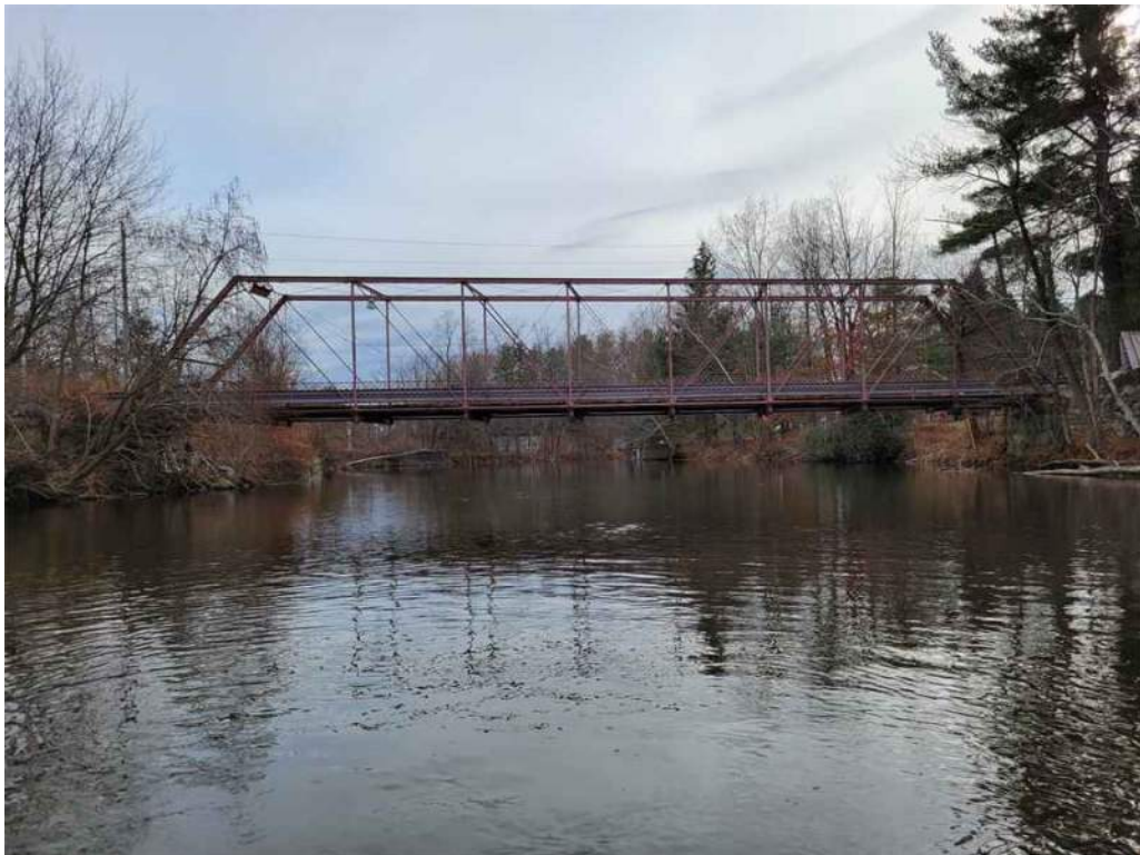
Photo 2: North elevation, looking south.
