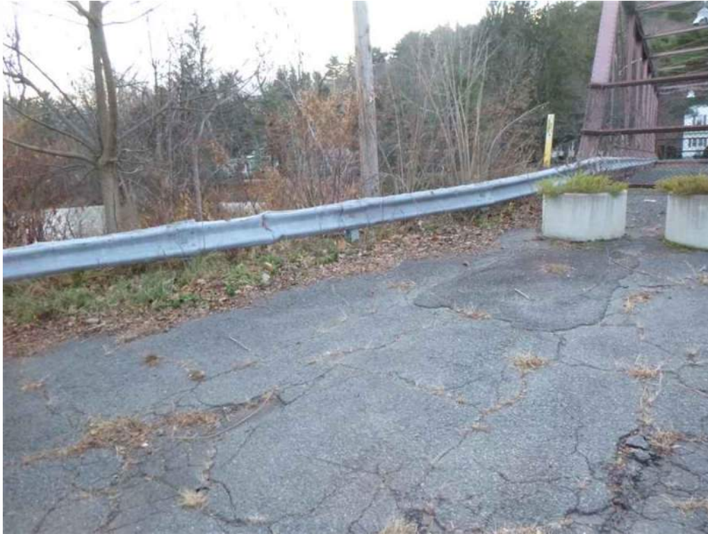
Photo 15: Typical approach guardrail, looking south.
