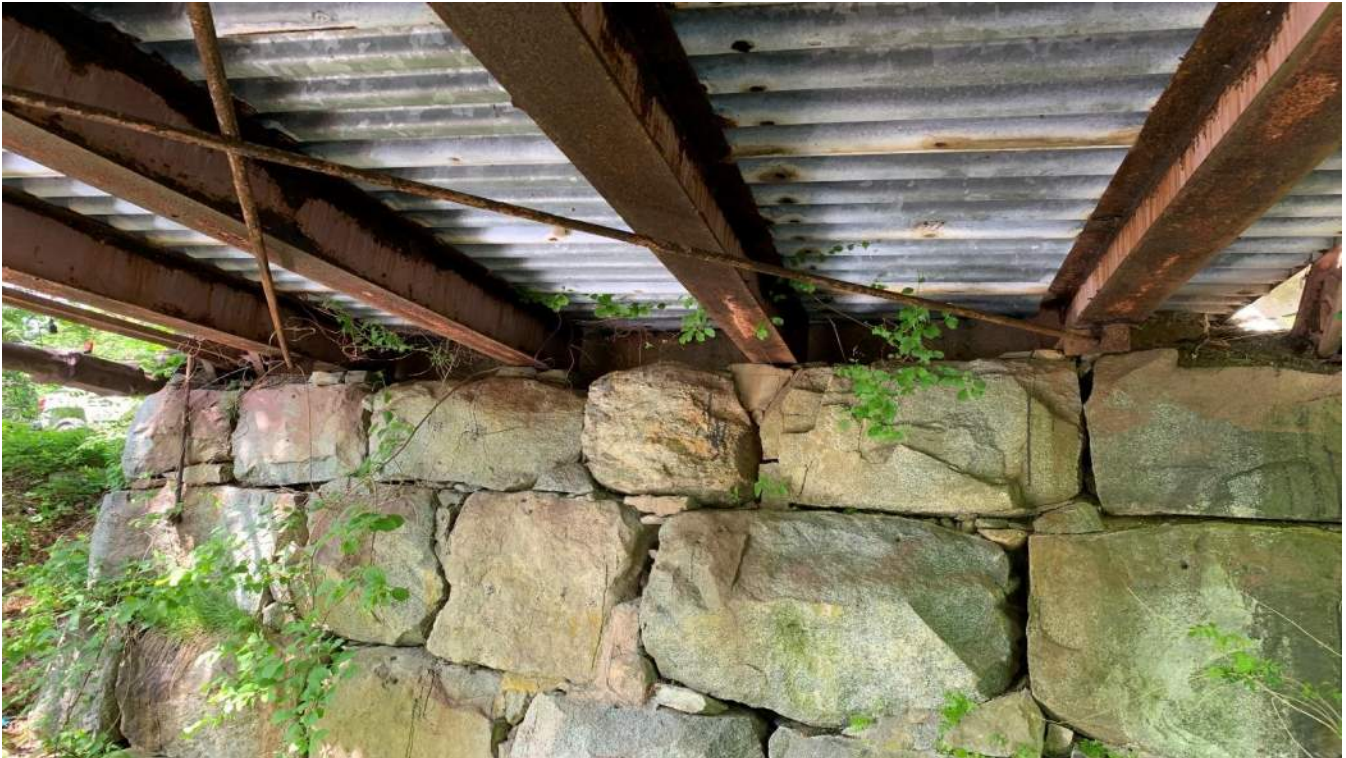
Photo 28: Begin Abutment Looking Southwest
