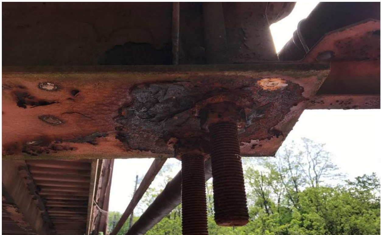
Photo 22: FB5 Right End Bottom Flange at U-Bolt Connection Looking East
