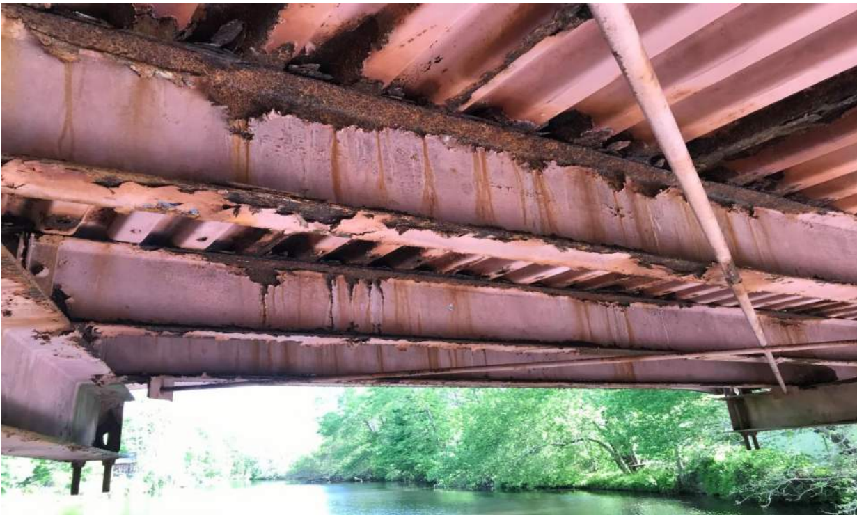
Photo 4: Panel 5 Stringers S1 – S3 Looking North
