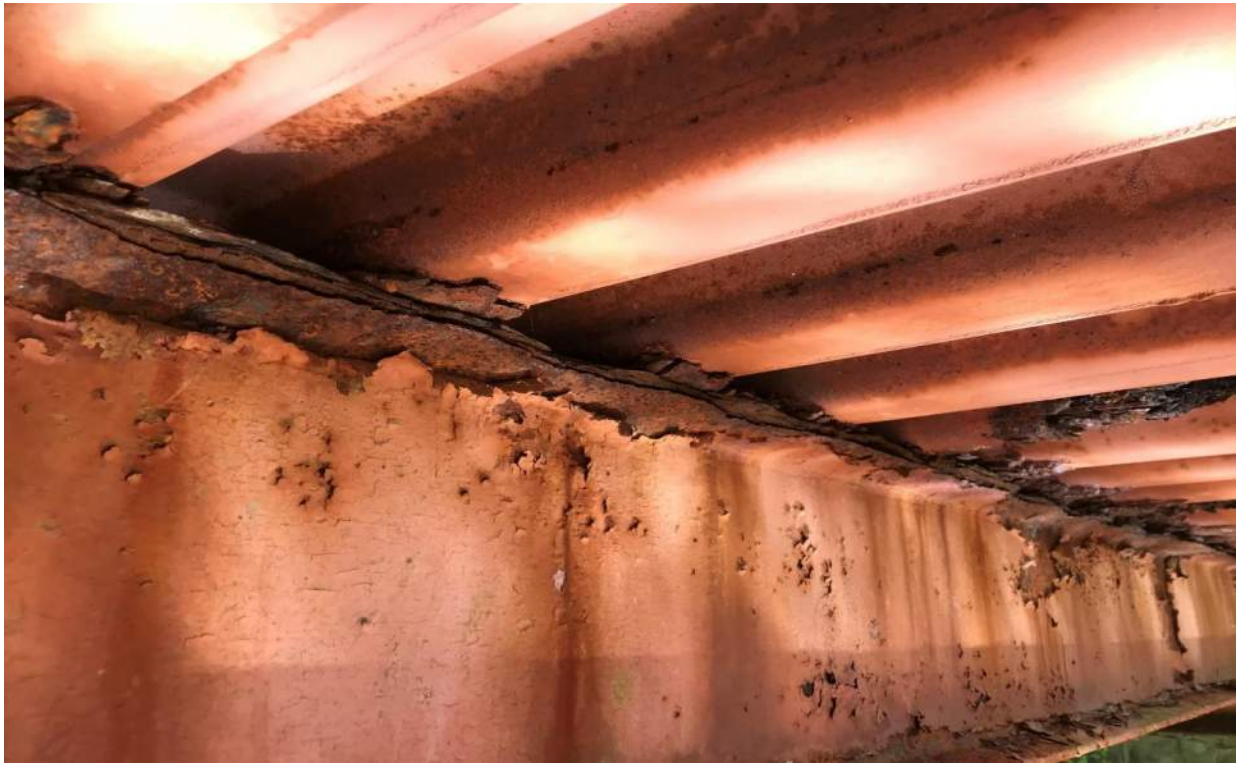
Photo 7: Panel 7 Stringer S4 Right Side Looking Northeast
