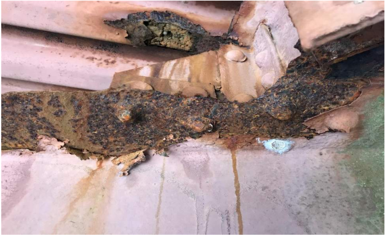
Photo 19: FB3 at Stringer S1 Looking West
