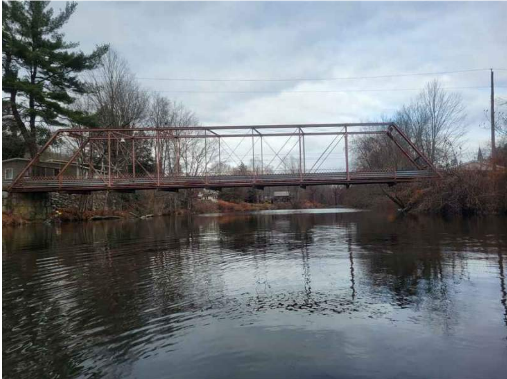
Photo 1: South elevation, looking north.
