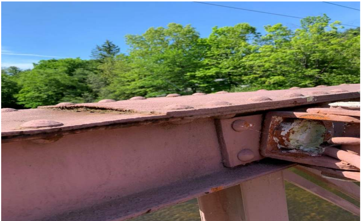
Photo 10: Right Truss, Panel Point U7 Looking Southwest
