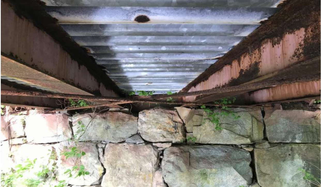
Photo 1: Panel 1 Stringers Looking West
