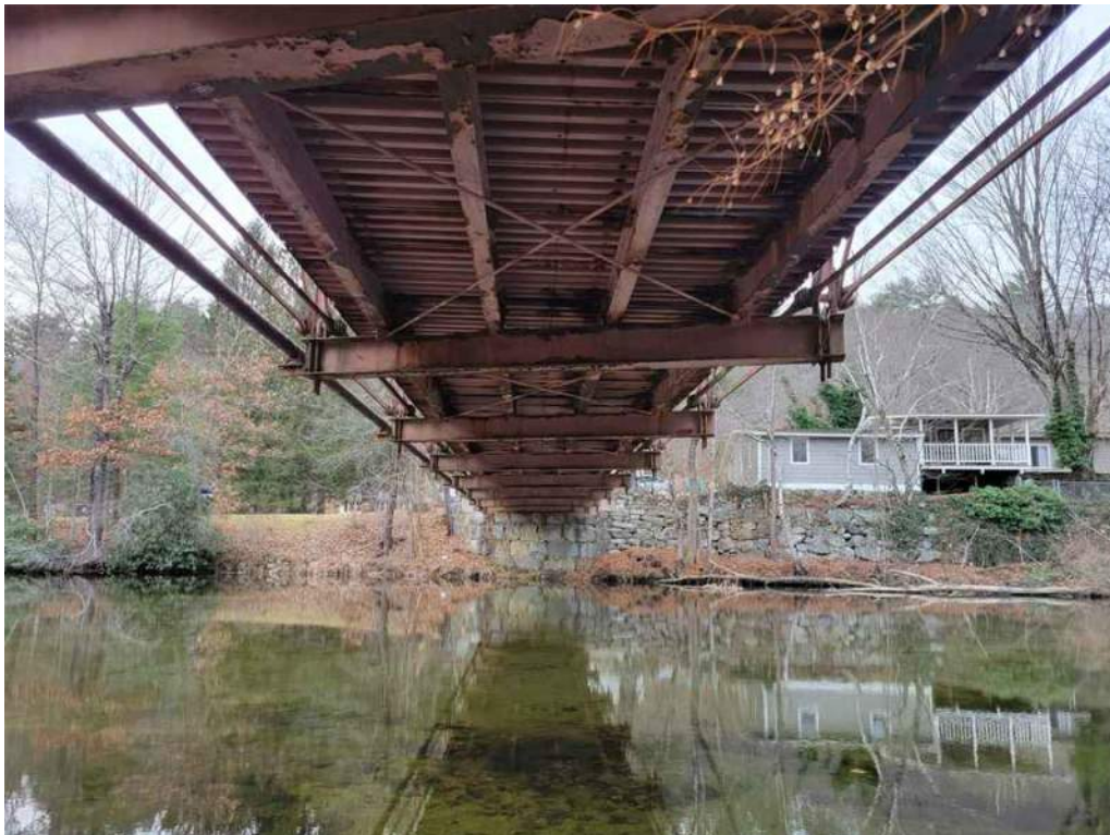
Photo 8: General view of underside of the bridge.
