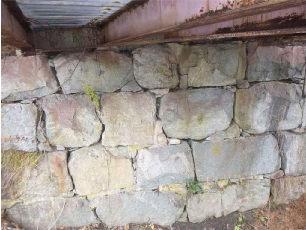
Photo 9: West abutment (Abutment 1).
