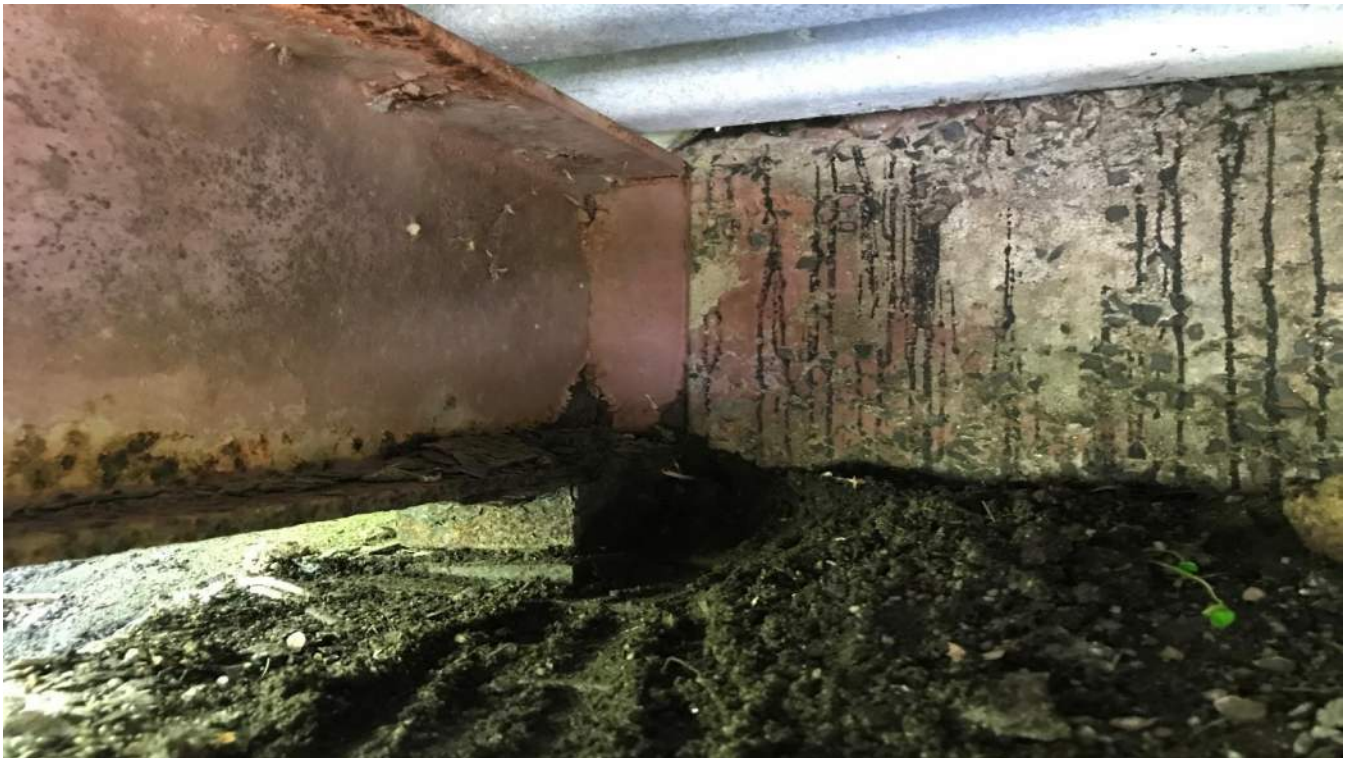
Photo 32: Stringer S1 Bearing at End Abutment Looking Northeast
