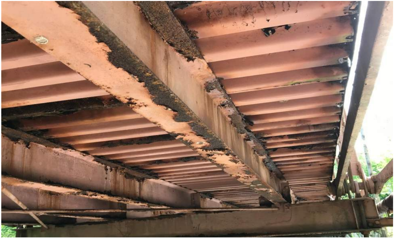
Photo 5: Panel 5 Stringer S4 Looking Northeast
