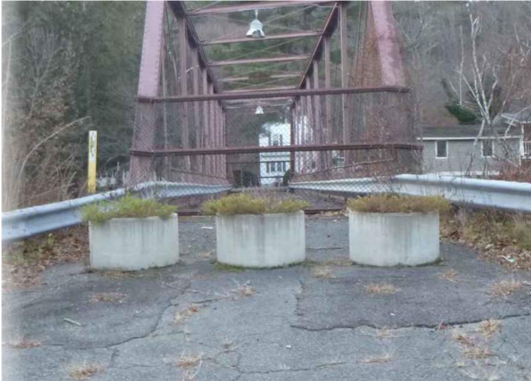
Photo 13: East approach barriers, looking west.
