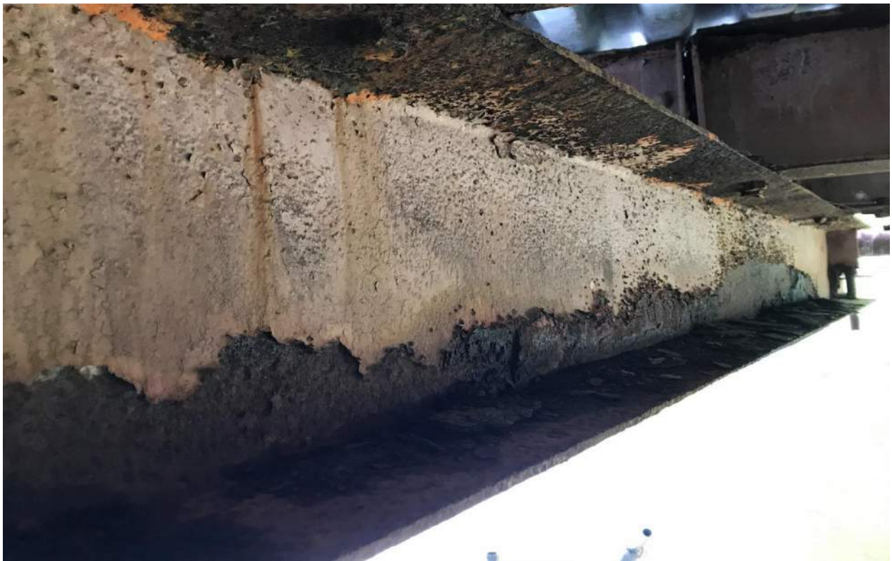
Photo 16: FB1 Begin Side Looking Southeast
