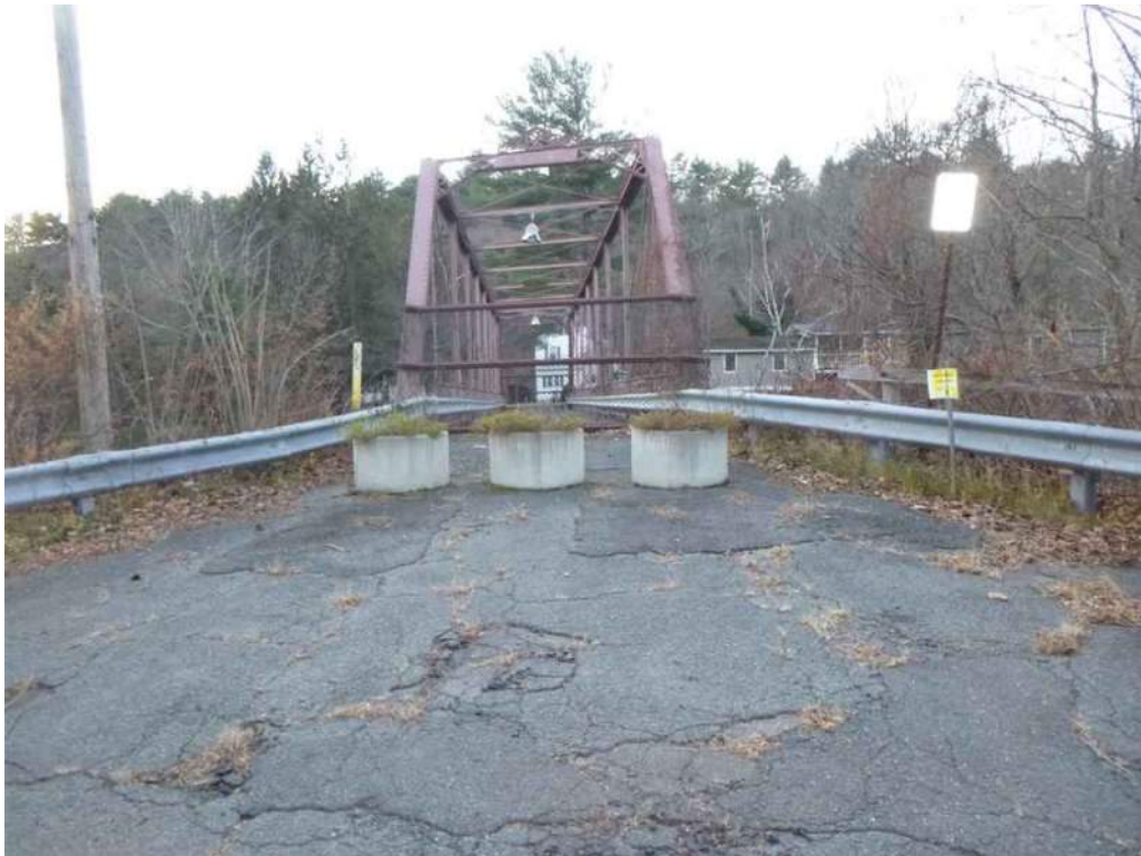
Photo 4: East approach, looking west.
