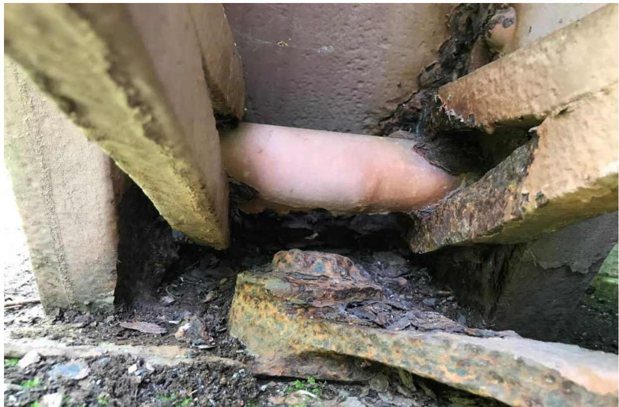
Photo 14: Left Truss Bearing at End Abutment Looking East
