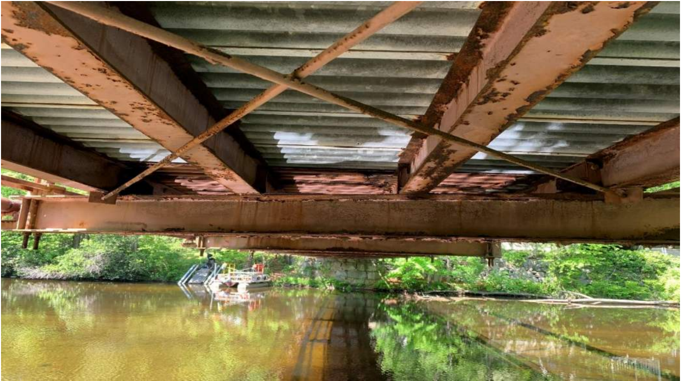
Photo 27: FB8 End Side Looking West
