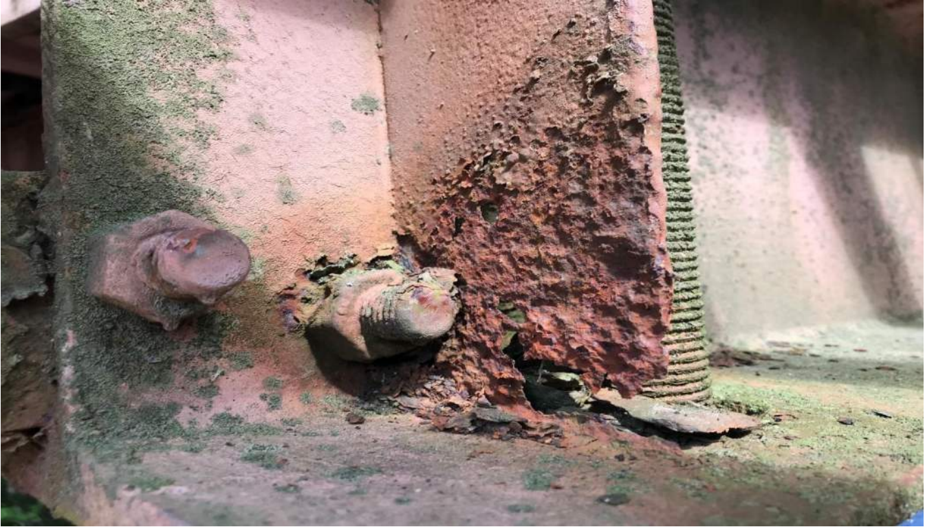
Photo 23: FB5 Right End, End Side Bearing Stiffener Looking Northwest
