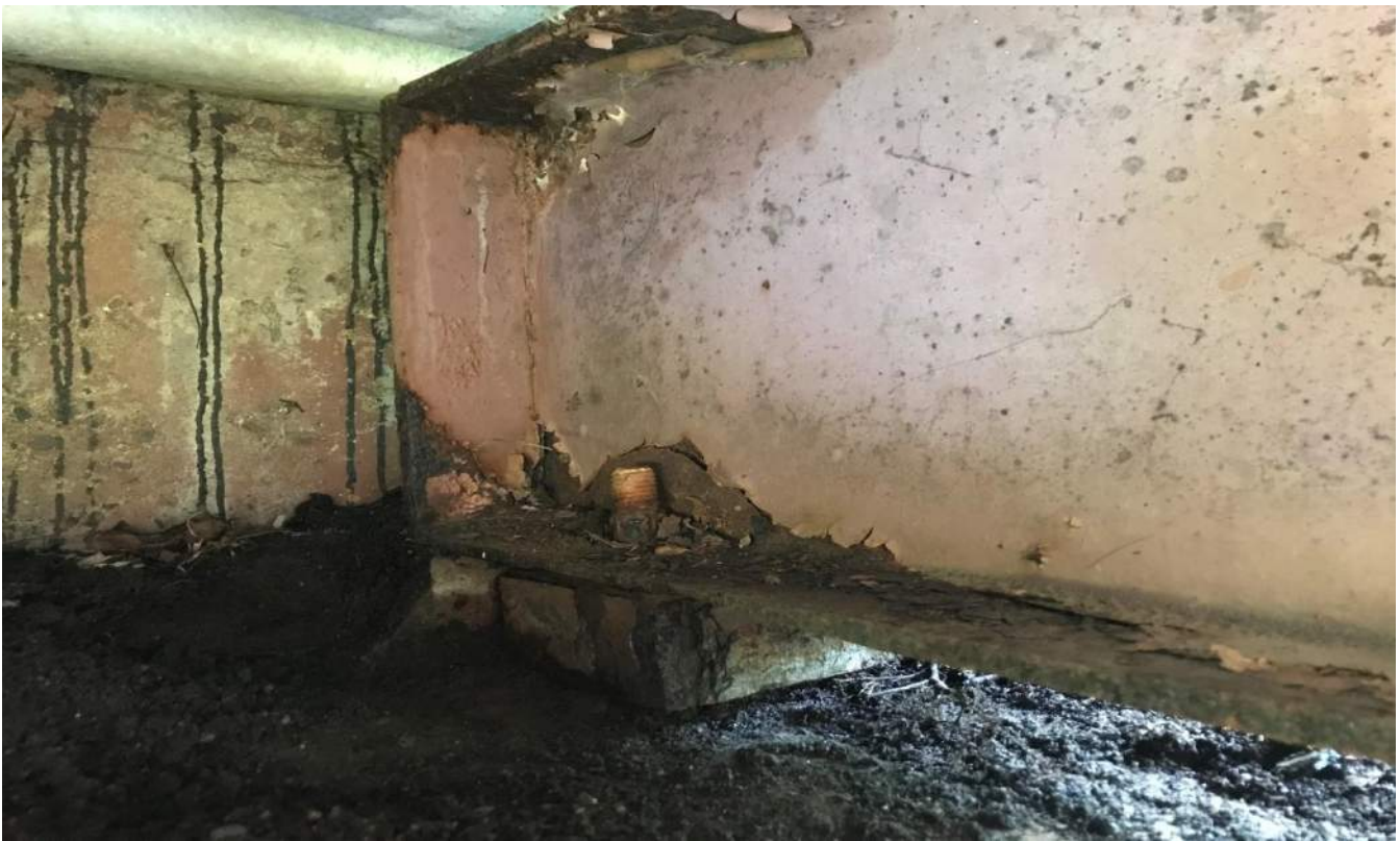
Photo 34: Stringer S4 Bearing at End Abutment Looking Southeast
