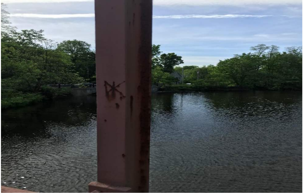
Photo 11: Right Truss Vertical L4U4 Looking Southeast
