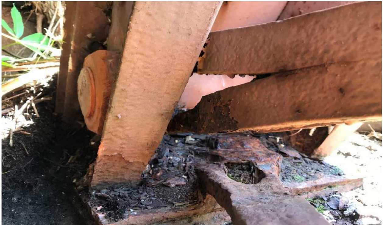
Photo 12: Right Truss Bearing at End Abutment Looking Southeast
