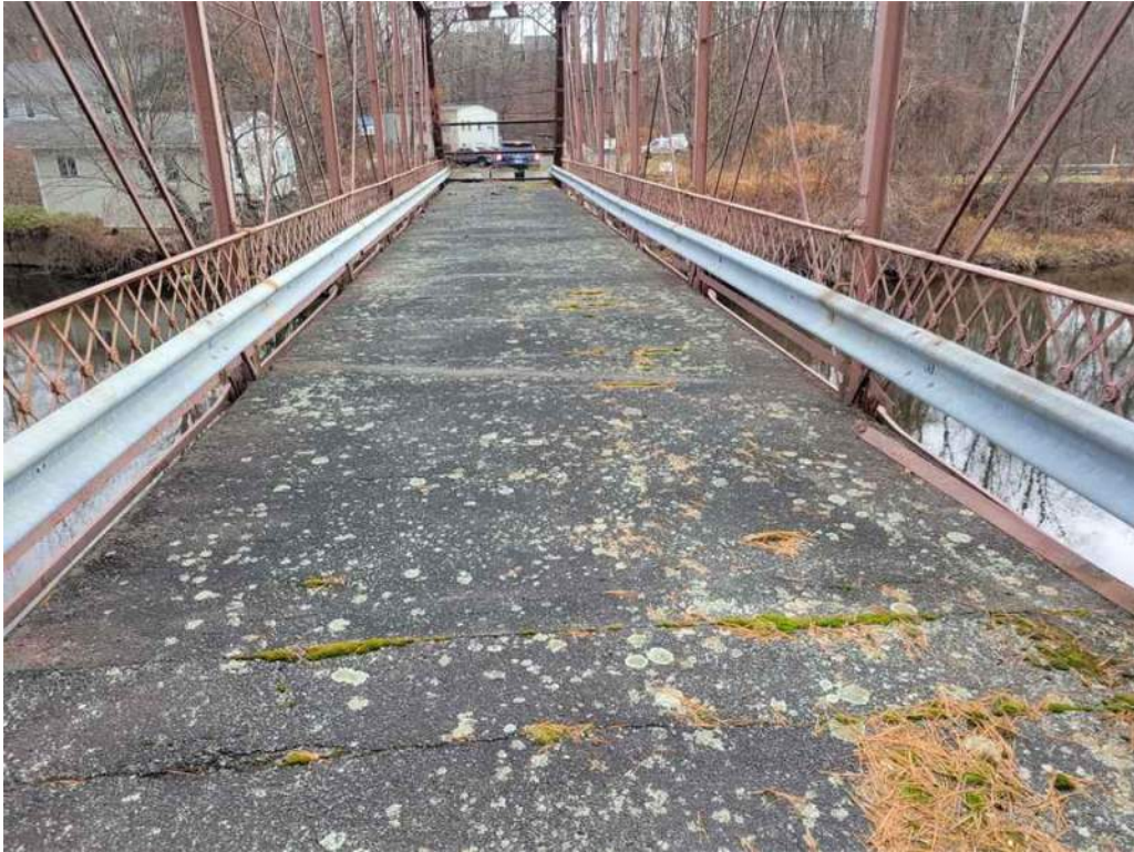
Photo 5: Typical top of deck.
