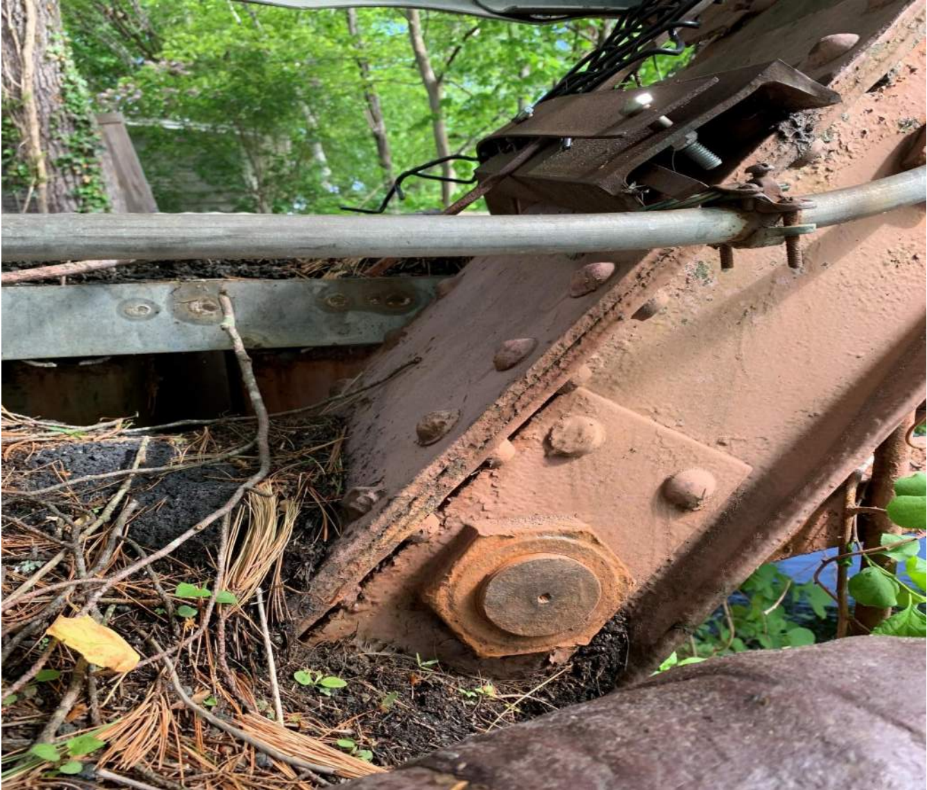
Photo 35: Right Truss Bearing at Begin Abutment Looking North
