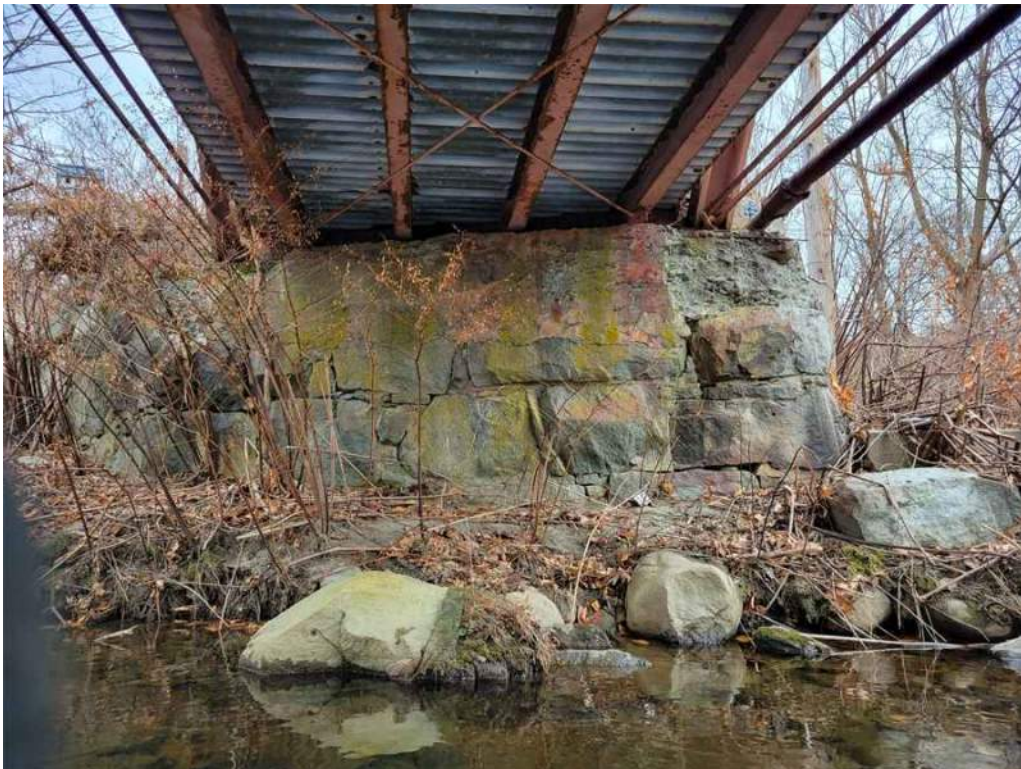
Photo 10: East abutment (Abutment 2).
