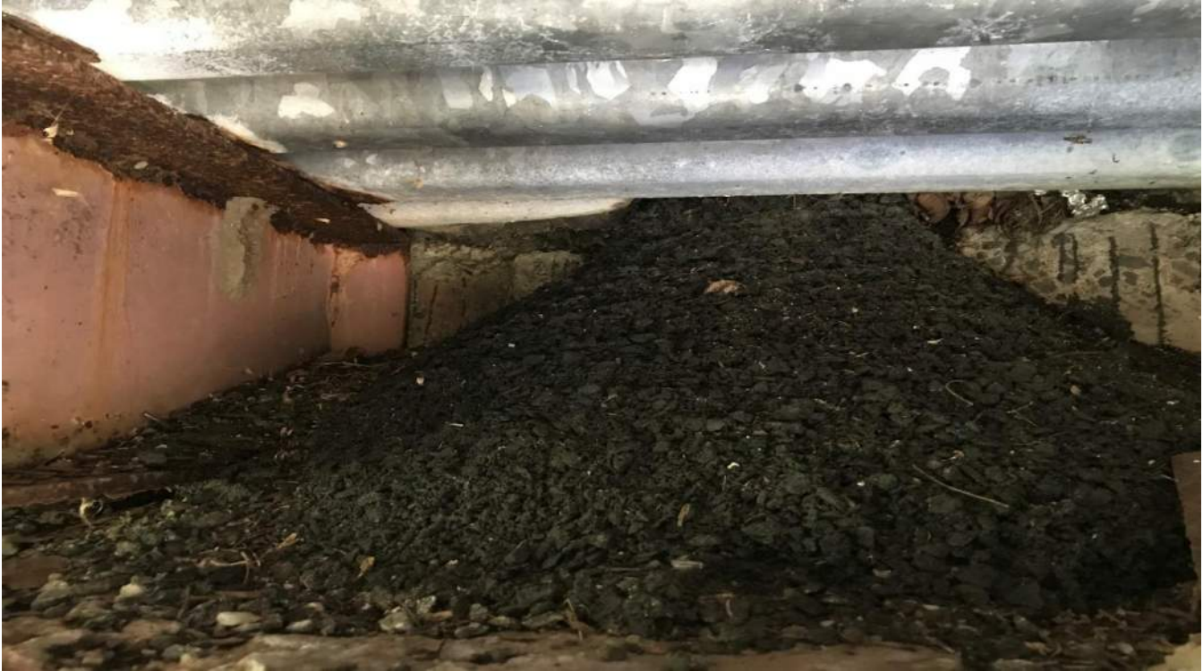
Photo 33: End Abutment Seat Between Stringer S2 & S3 Looking East
