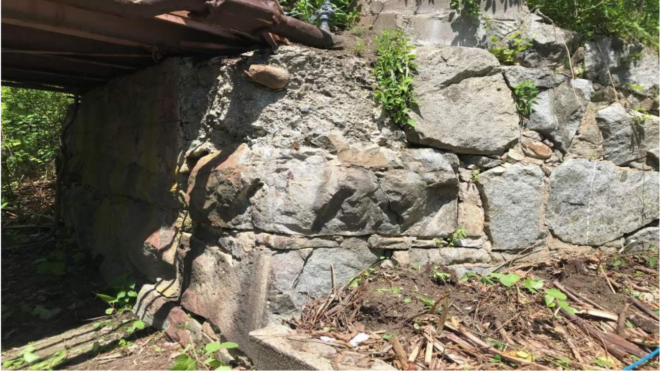
Photo 31: End Abutment Right Corner Looking Northeast
