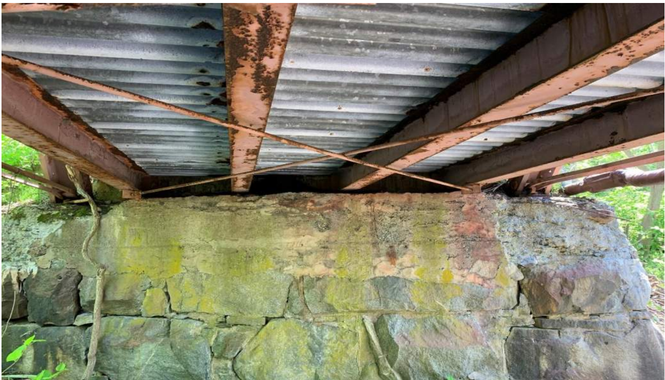
Photo: 30: End Abutment Looking East
