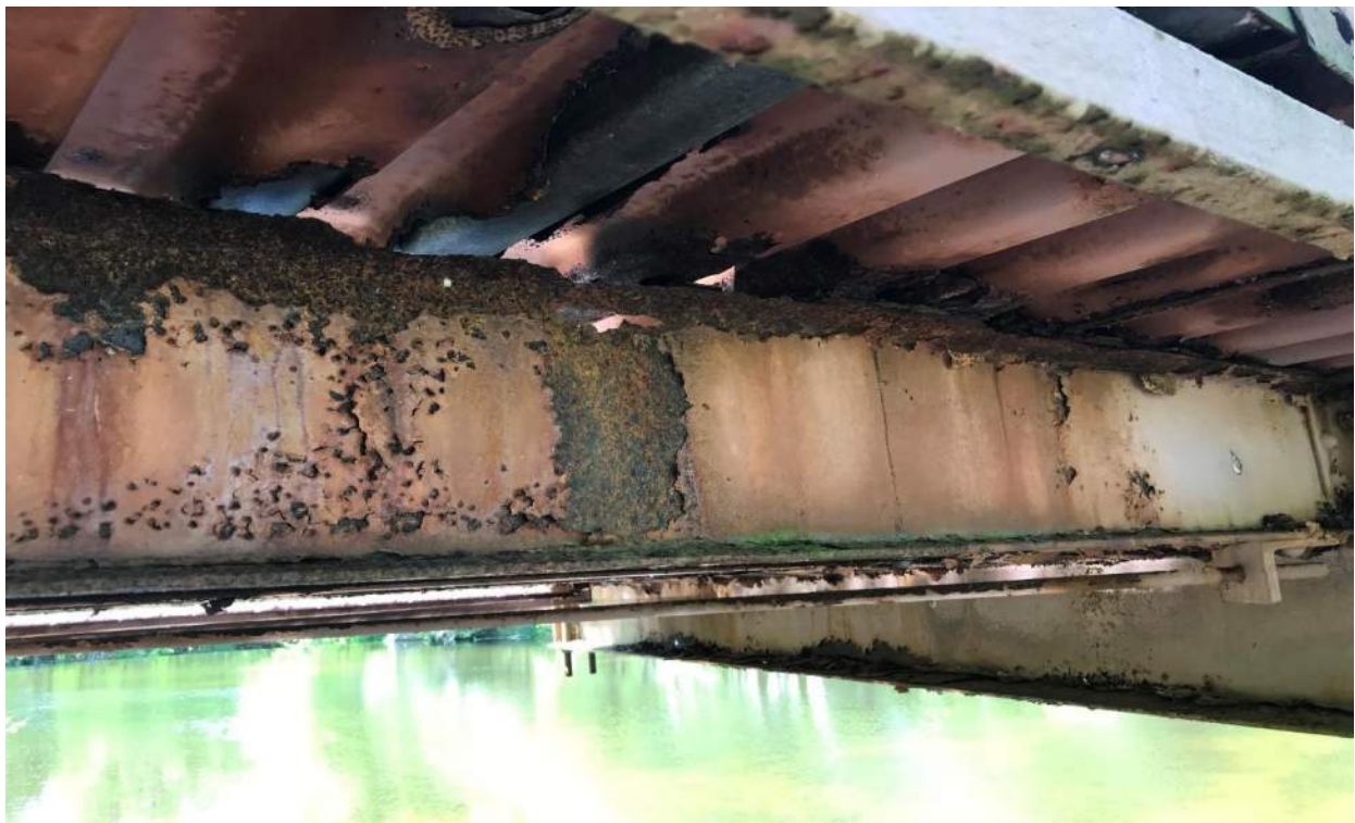
Photo 8: Panel 8 Stringer S1 Left Side Near FB7 Looking Southwest
