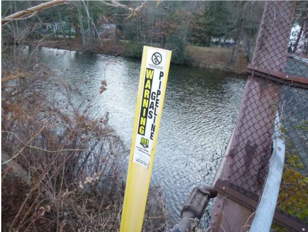
Photo 39: At the southeast approach there is a sign detailing the gas line attached to the bridge.
