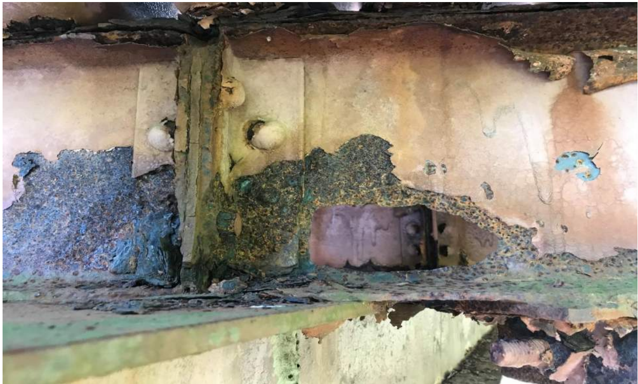
Photo 2: Panel 3, Stringer S1 at FB3 Looking South
