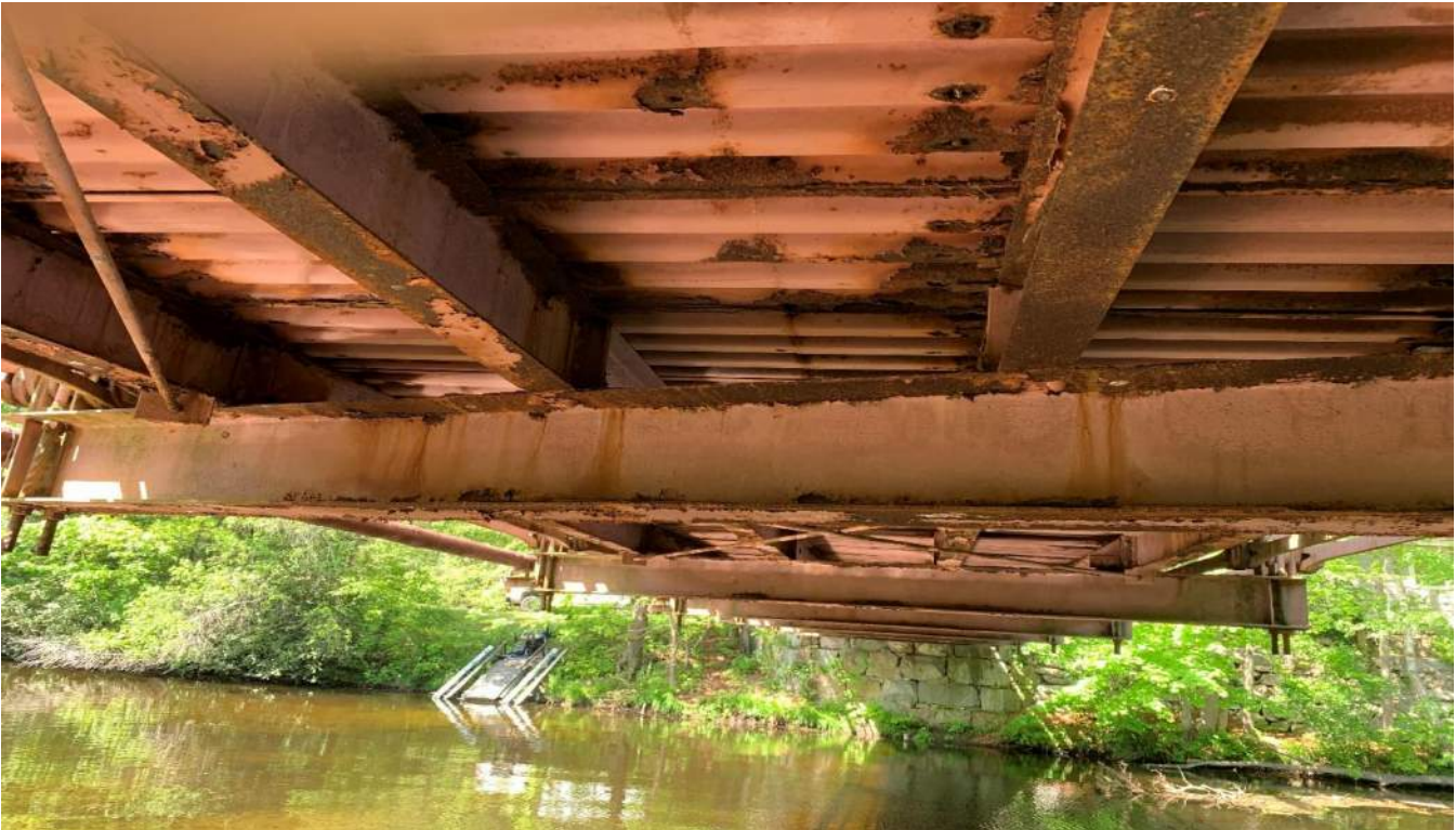
Photo 24: FB6 End Side Between Stringer S1 & S4 Looking West
