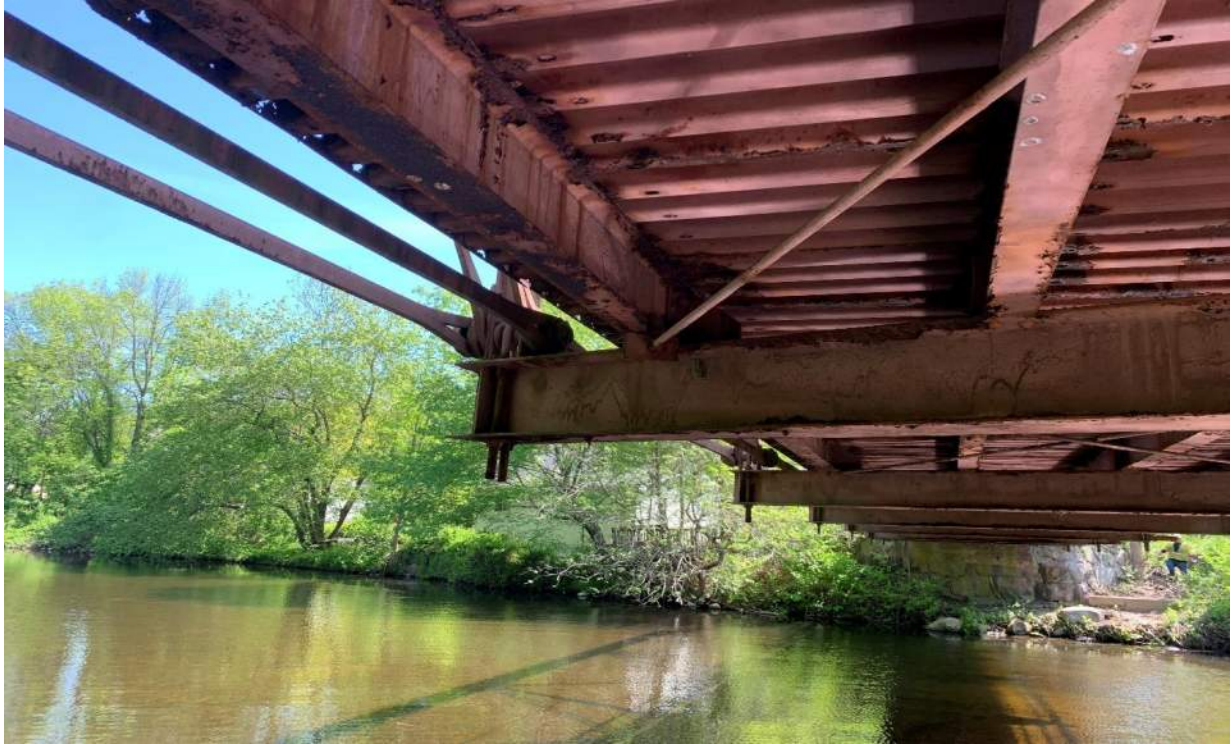
Photo 3: FB3 Left End, Begin Side Looking East
