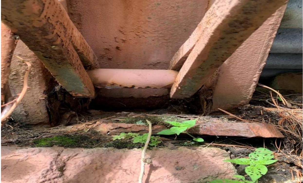
Photo 13: Right Truss Bearing at Begin Abutment Looking West
