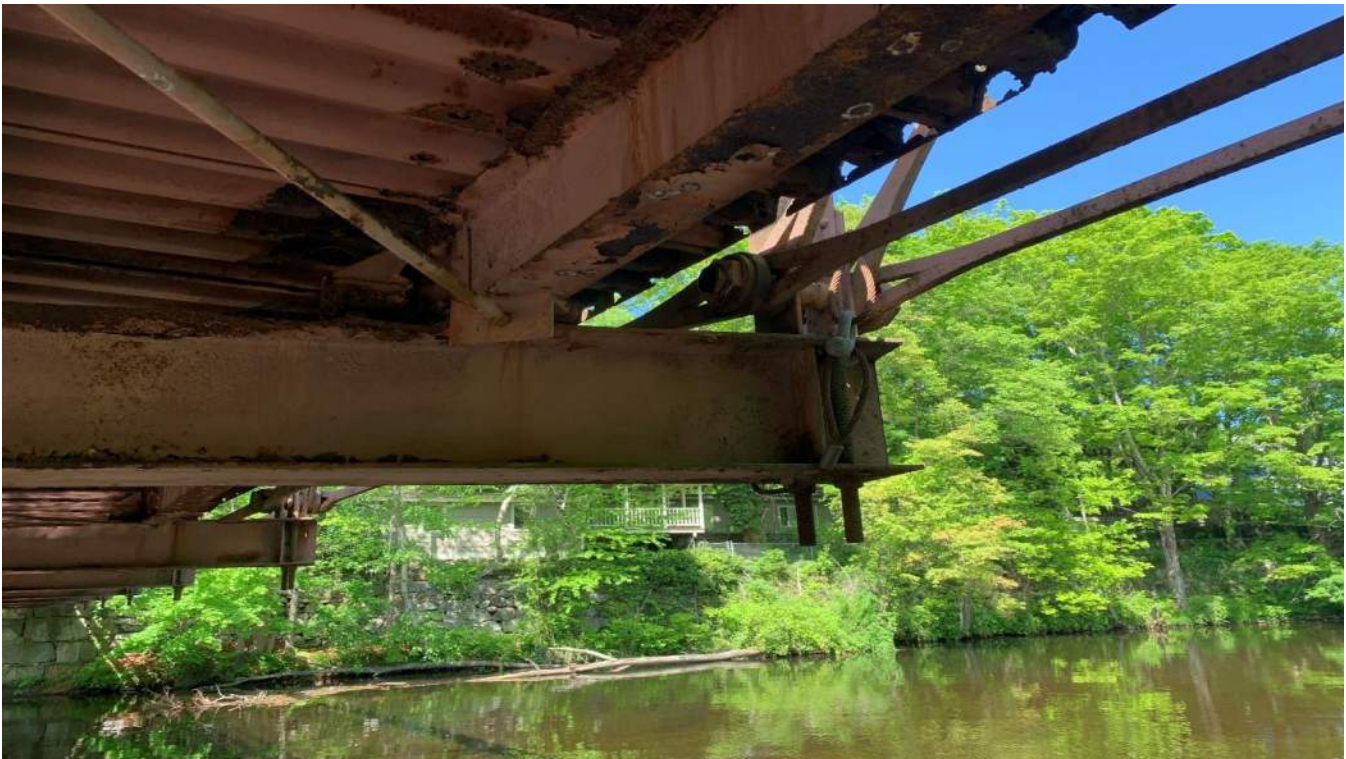
Photo 26: FB7 Left End , End Side Looking Northwest
