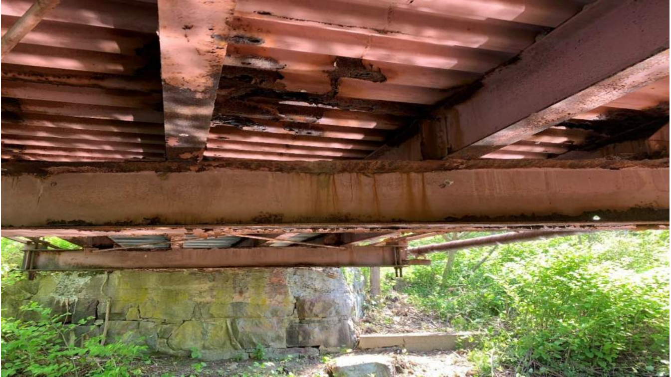
Photo 25: FB7 Begin Side Between Stringer S1 & S4 Looking East
