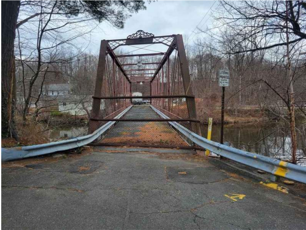
Photo 3: West approach, looking east.
