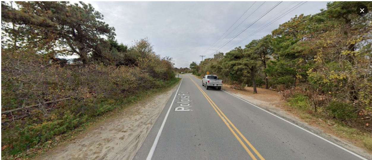
Limit of work on Polpis Road, facing Southwest towards the the intersection between Milestone Road and Polpis Road
