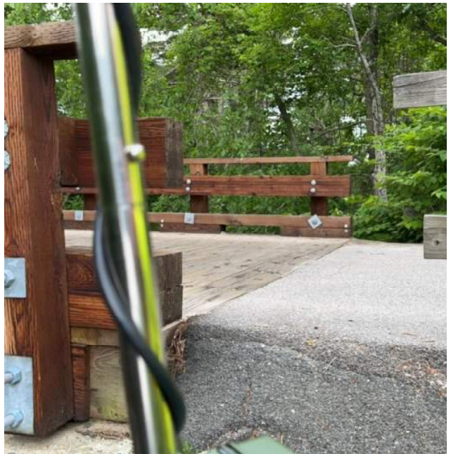
Photo #4: Location 1. Facing west.
