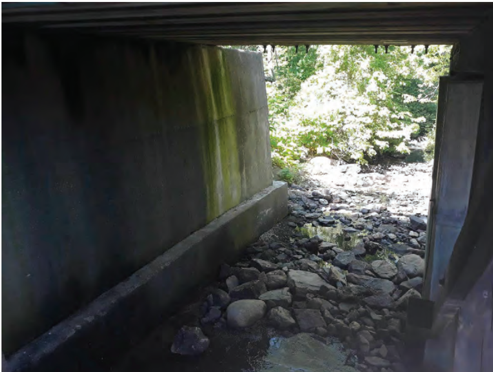
Figure A: Downstream of Bridge:
