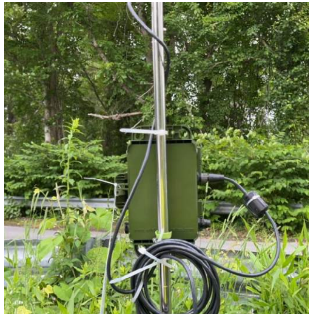
Photo #4: Location 2. Facing west.
