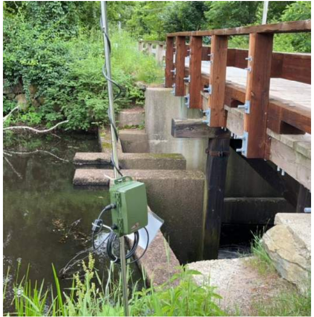
Photo #2: Location 1. Facing south.
