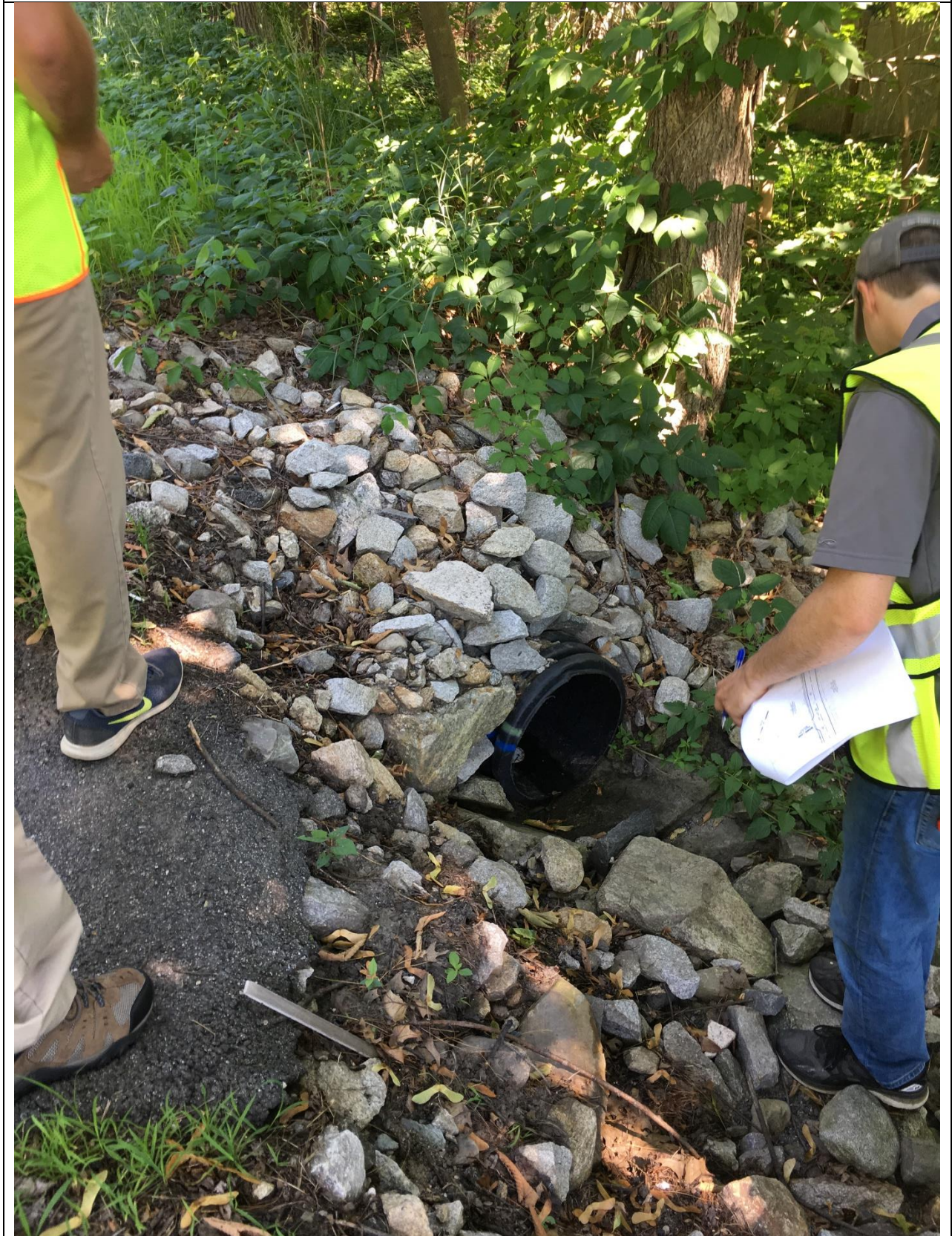
Photo 4 – View looking North at Proposed Outlet Sediment Trap – Existing Outlet Shown
