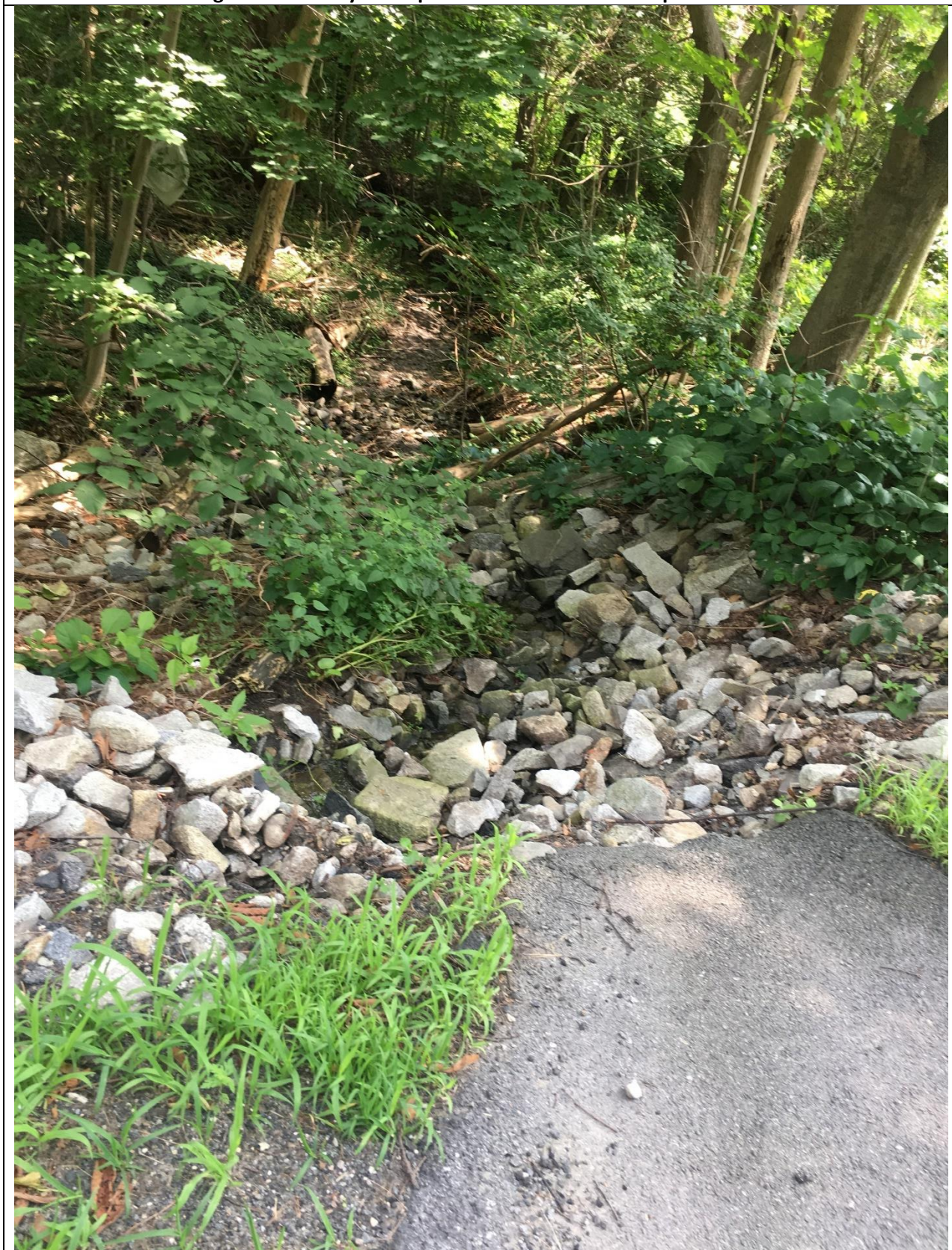
Photo 3 – View looking from roadway at Proposed Outlet Sediment Trap
