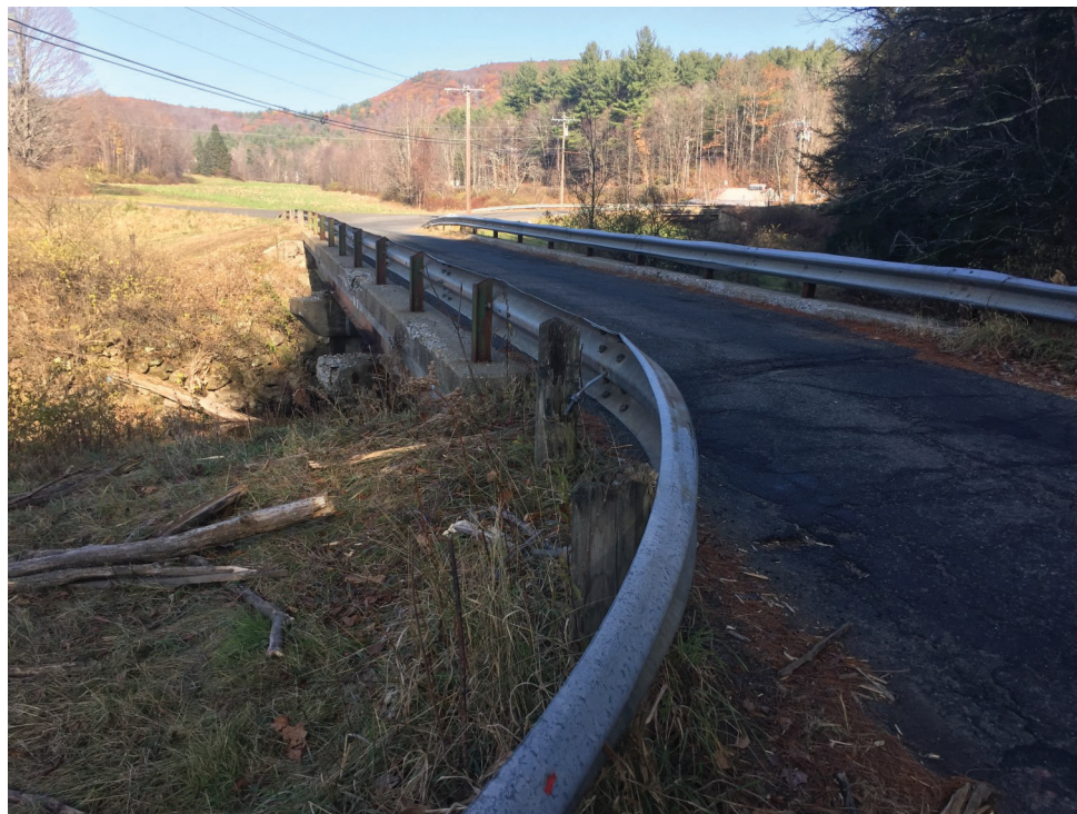
View of the bridge taken from North Poland Road—facing north.
