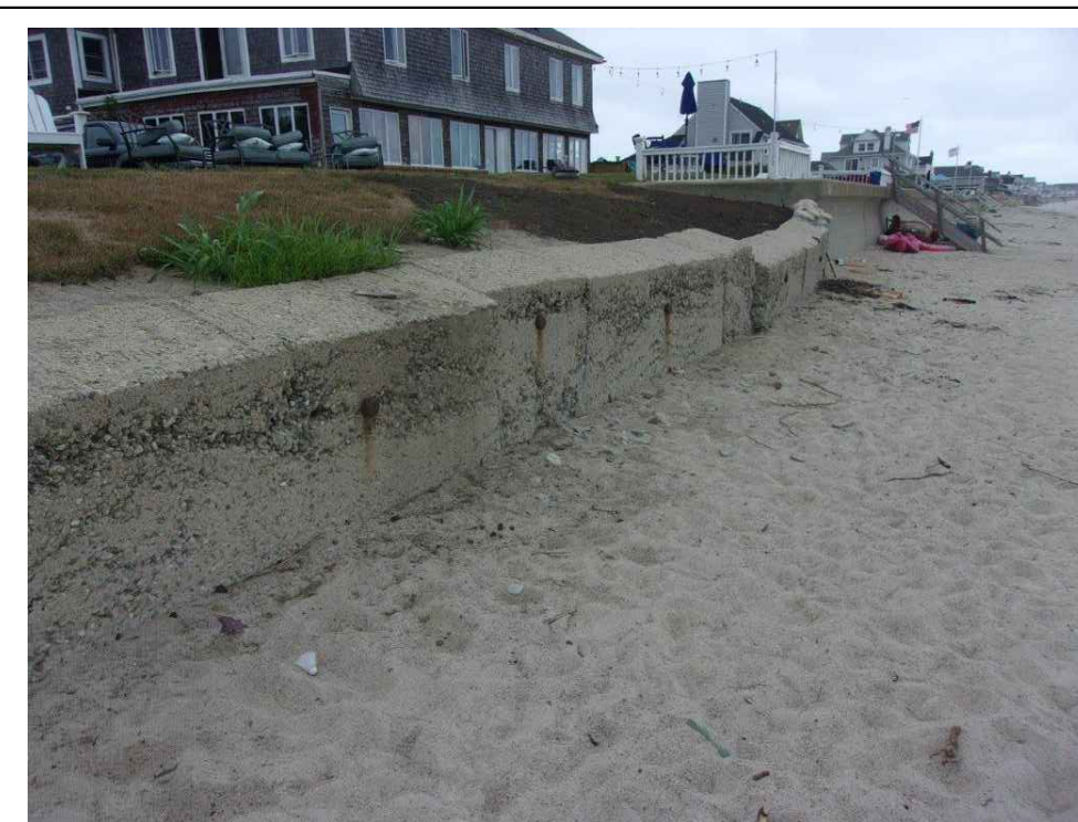
SEAWALL AT STA. 32+96 TO 33+53 WITH STEEL & TIEBACKS (ALSO IN 3 PHOTOS DIRECTLY ABOVE)
