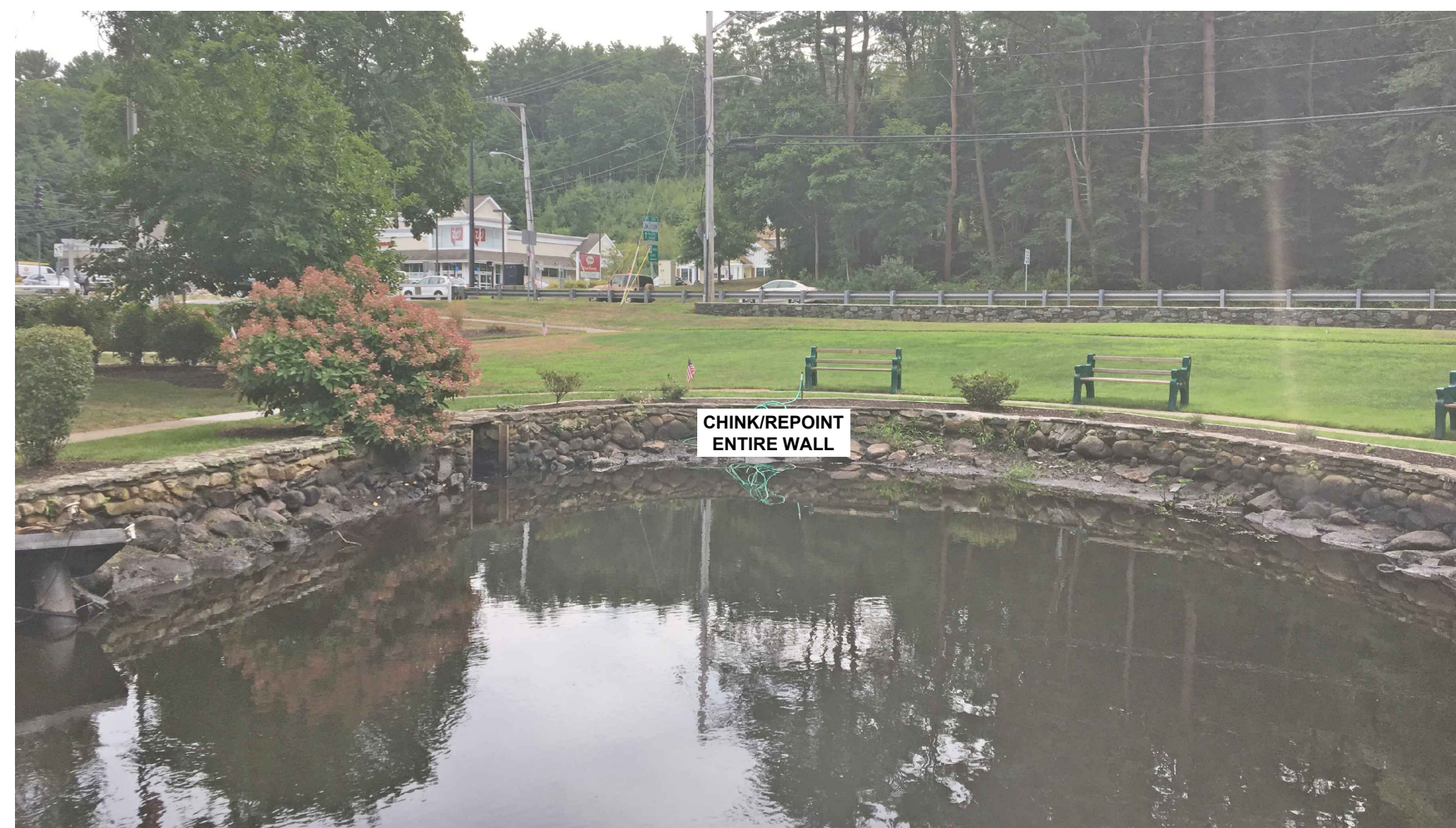
8 LAGOON WALL REPAIR NOT TO SCALE
