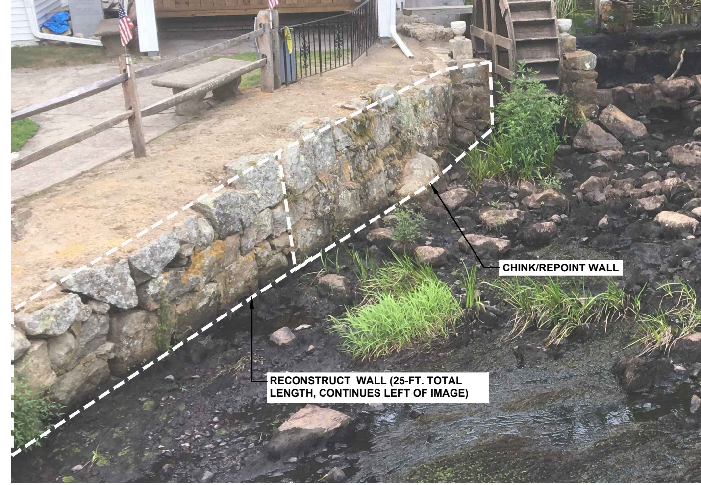
2 DOWNSTREAM CHANNEL WALL REPAIR NOT TO SCALE
