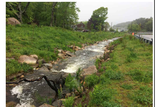
EXAMPLE RIFFLE-POOL CHANNEL NOT TO SCALE
