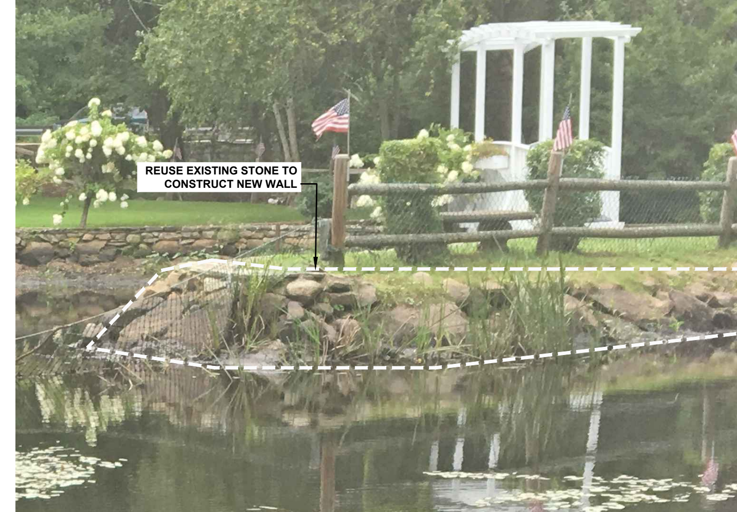
5 RIVER CHANNEL WALL CONSTRUCTION NOT TO SCALE
