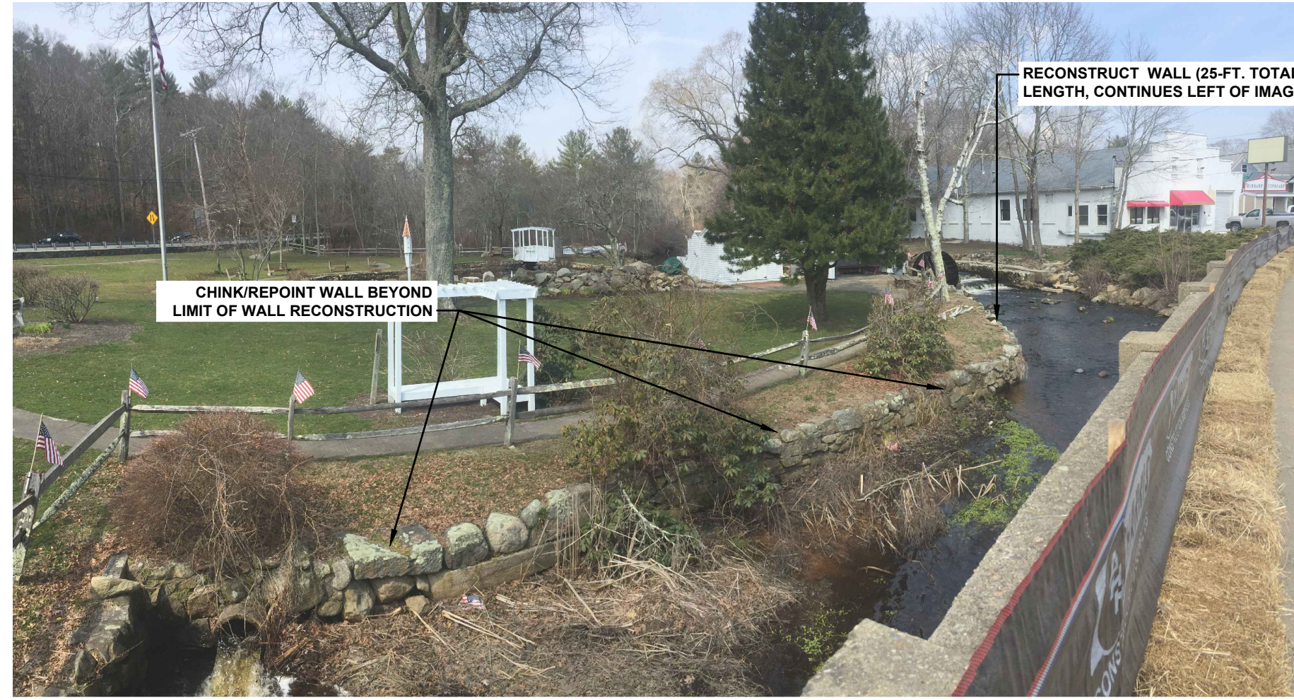
1 DOWNSTREAM CHANNEL WALL REPAIR NOT TO SCALE
