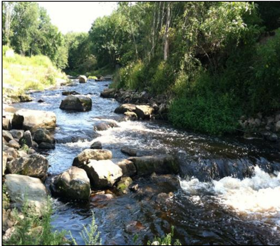
Figure 4. Example constructed riffle-pool nature-like fishway.
