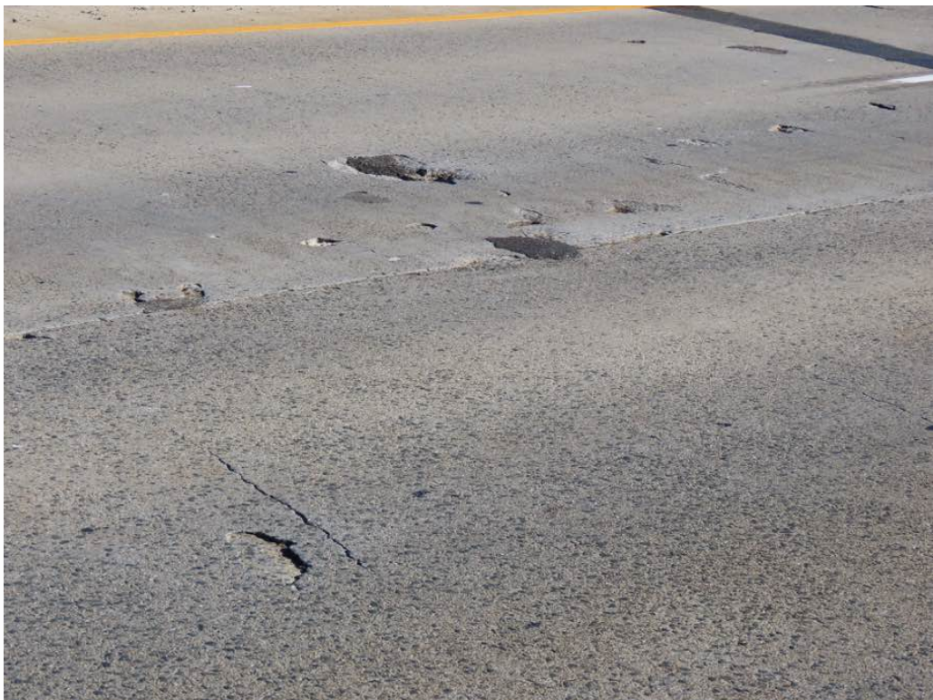
Photo 3: Close up of previous photo - Span 1 concrete deck/wearing surface with transverse cracks and numerous partial filled potholes - Typical.
