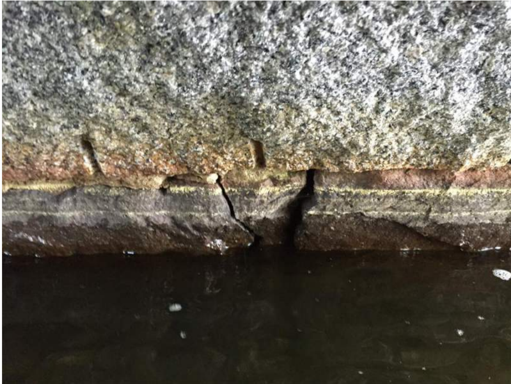
Photo 7: East Arch Ring above Spring Line Approximately 7'-5" from South Fascia
