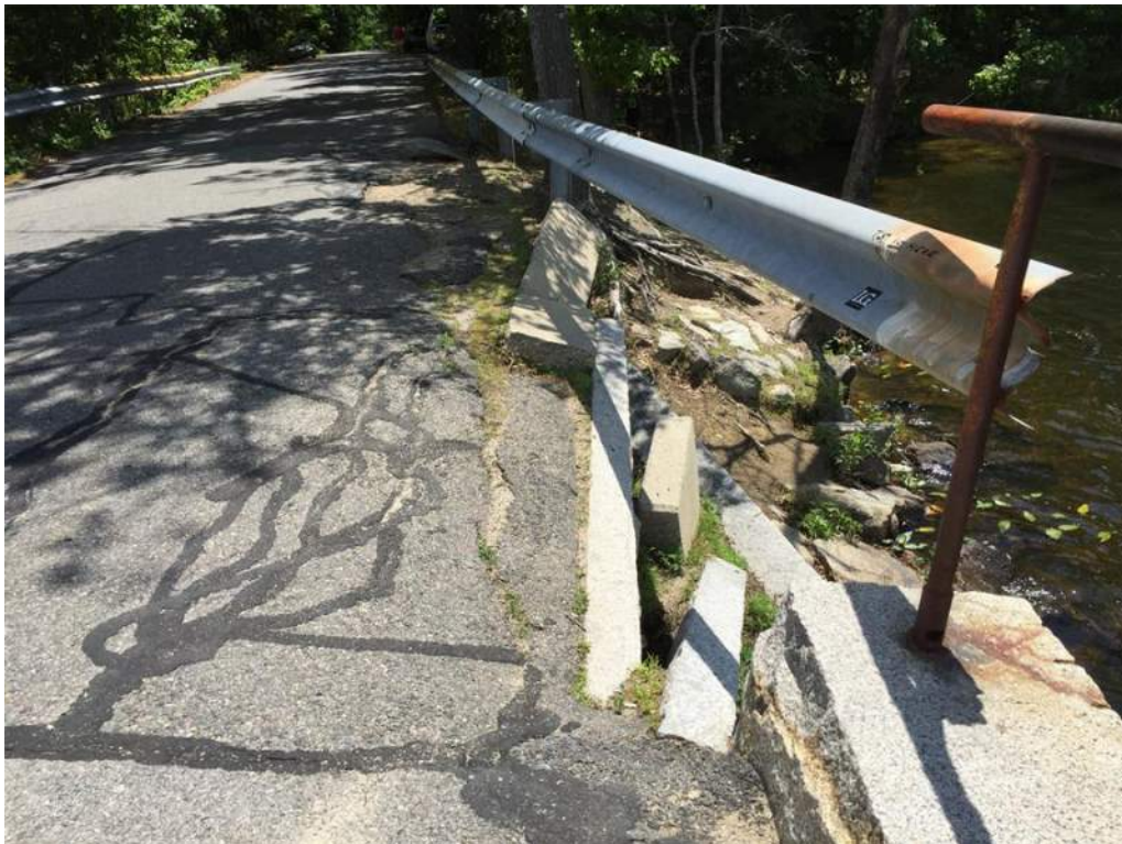
Photo 16: Southeast Bridge Rail and Transition Rail Tack Weld Connection
