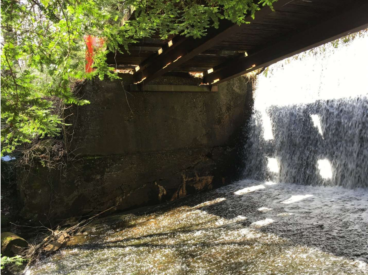
Figure 3. Right concrete training wall and concrete apron
