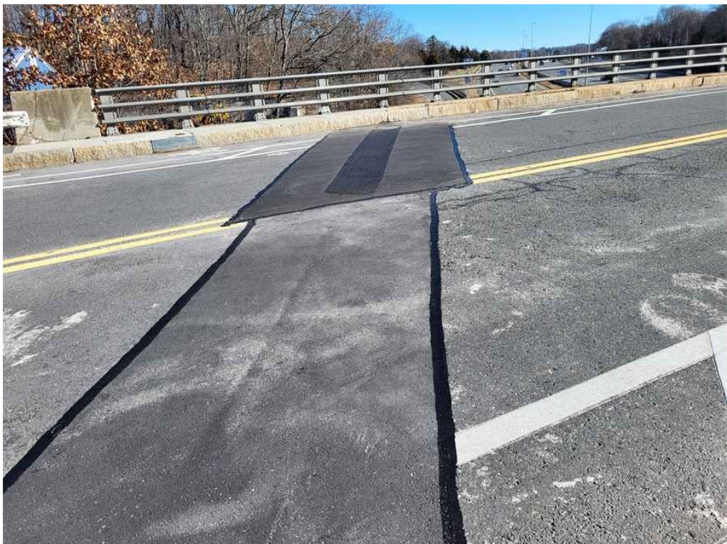
Photo 20: Deck joints at north abutments has been repaired since last inspection.
