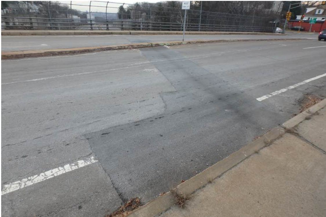
Photo 4: Southbound roadway, Pier joint.
