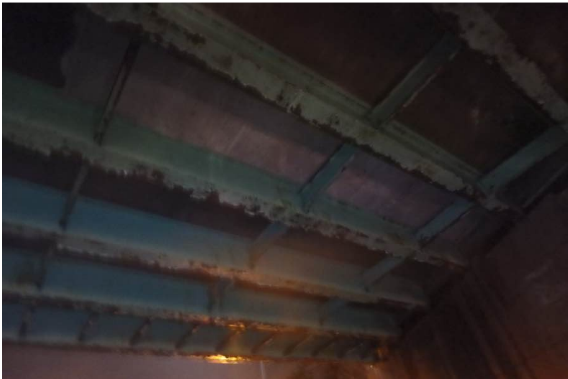
Photo 10: Span 2, Bay 4 repair area.
