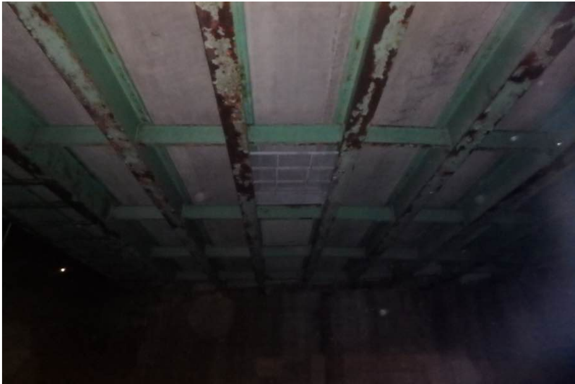
Photo 9: Span 2, Bay 4 screening.
