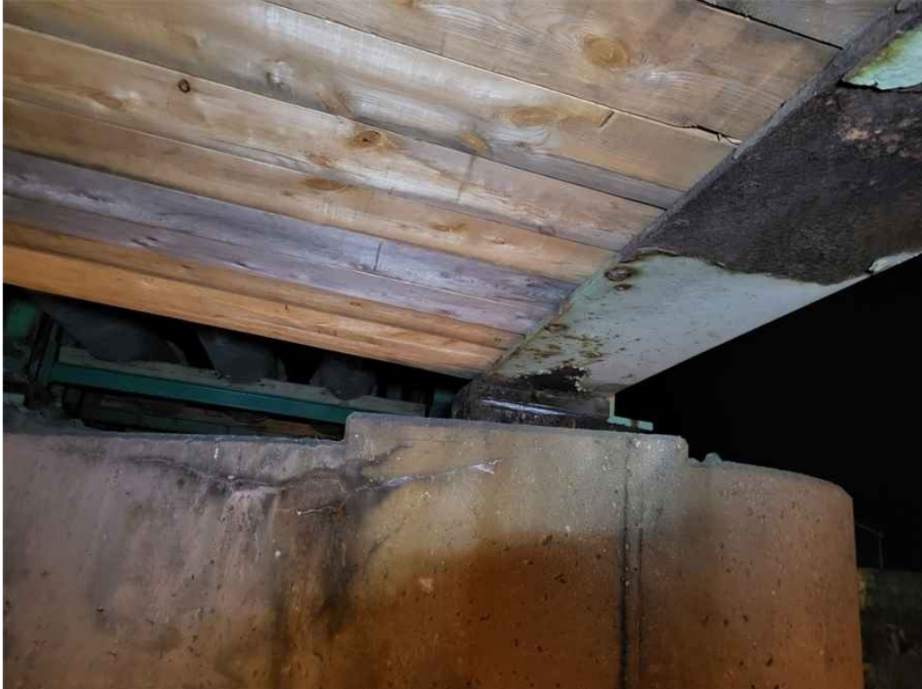
Photo 34: West face of Girder 8, span 2 is hidden by timber shielding.
