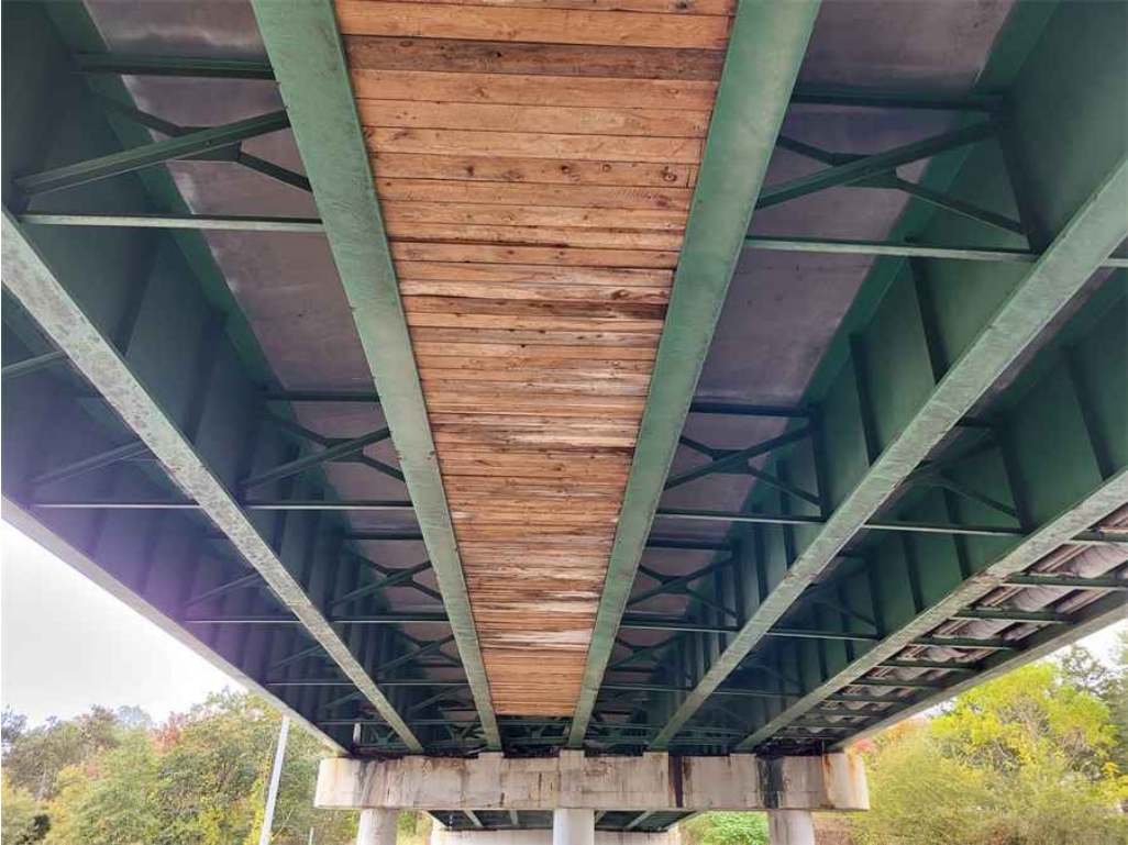
Photo 12: Deck, span 2: Bay 4 shielded over the westbound roadway. (Looking South).
