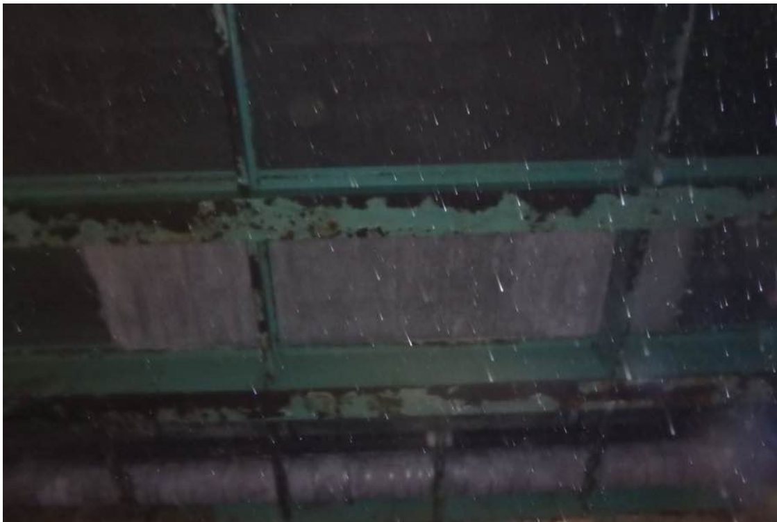
Photo 12: Span 2, Bay 9 repair between diaphragms 4 - 6.
