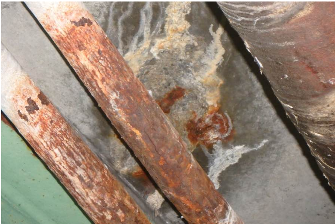
Photo 8: Span 1, Bay 10, spalling at the north end.
