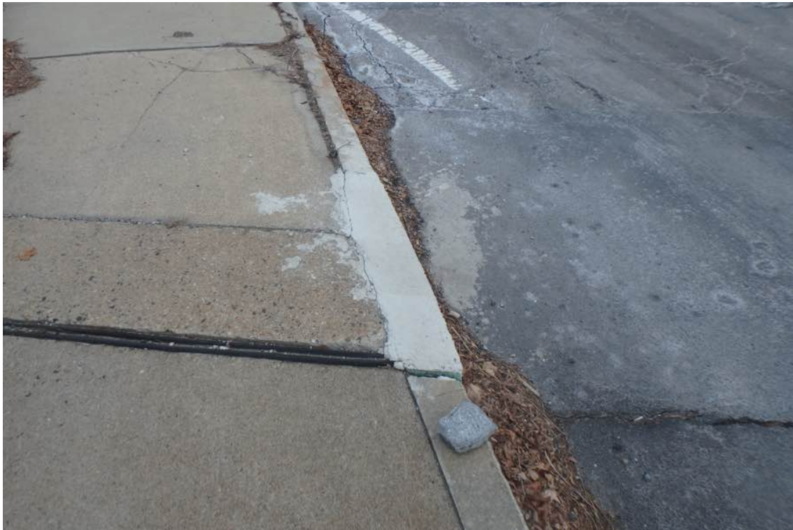
Photo 13: West curb, repaired section in the north approach corner.
