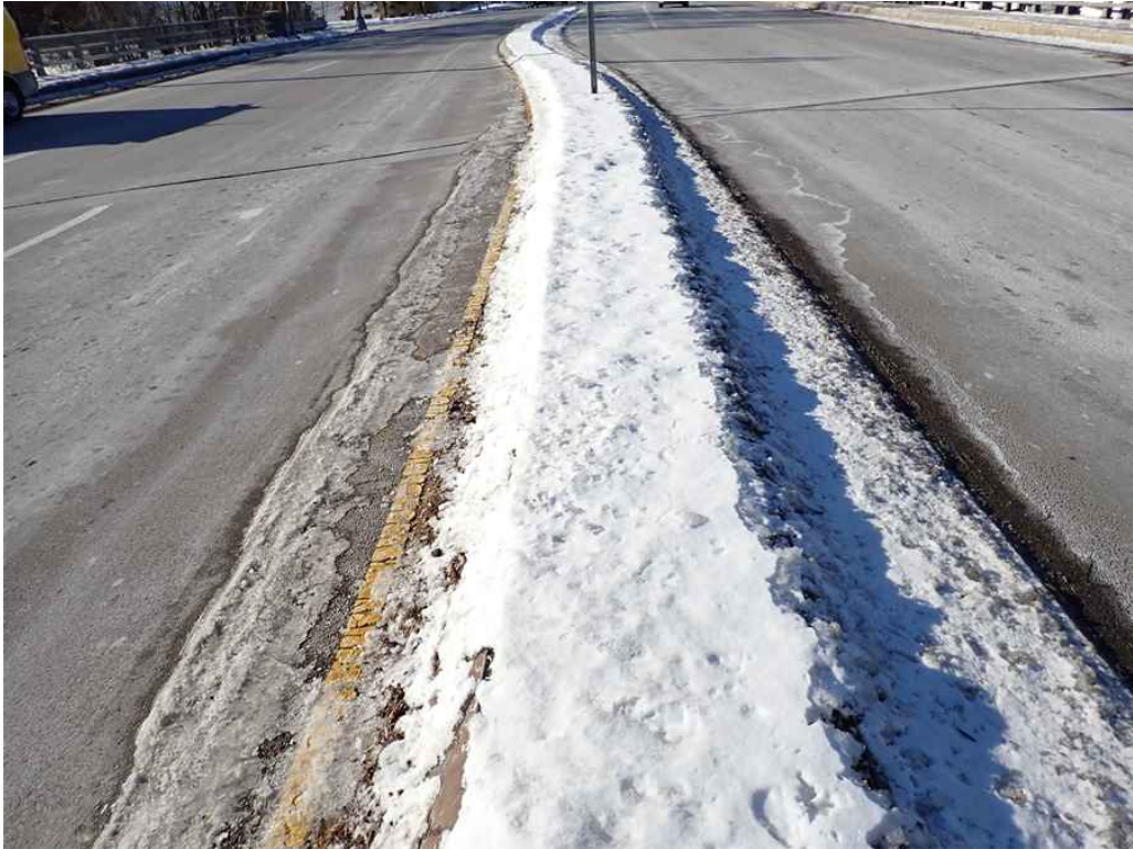
Photo 3: Median covered in snow and ice.
