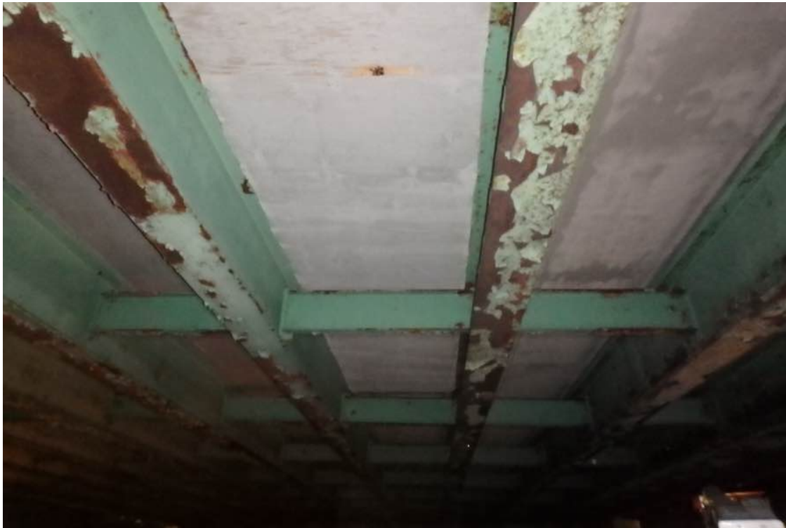
Photo 7: Span 1, Bay 7, repair area.
