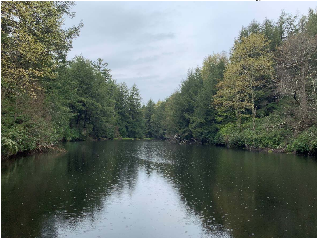
Looking upstream from the dam at the impoundment.
