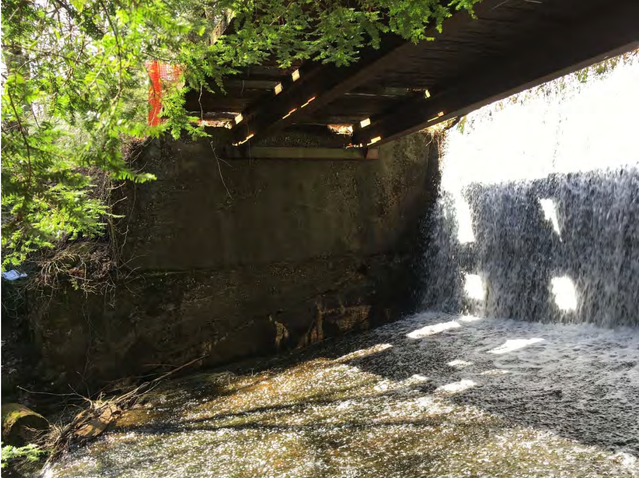
Figure 3. Right concrete training wall and concrete apron
