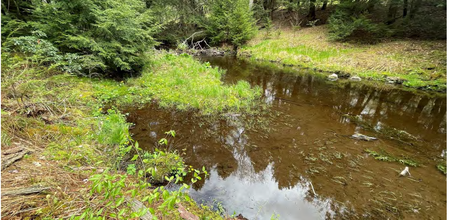
Photo #3: View of slower flowing depositional area, where the stream begins to pond above the Becker Pond Dam.
