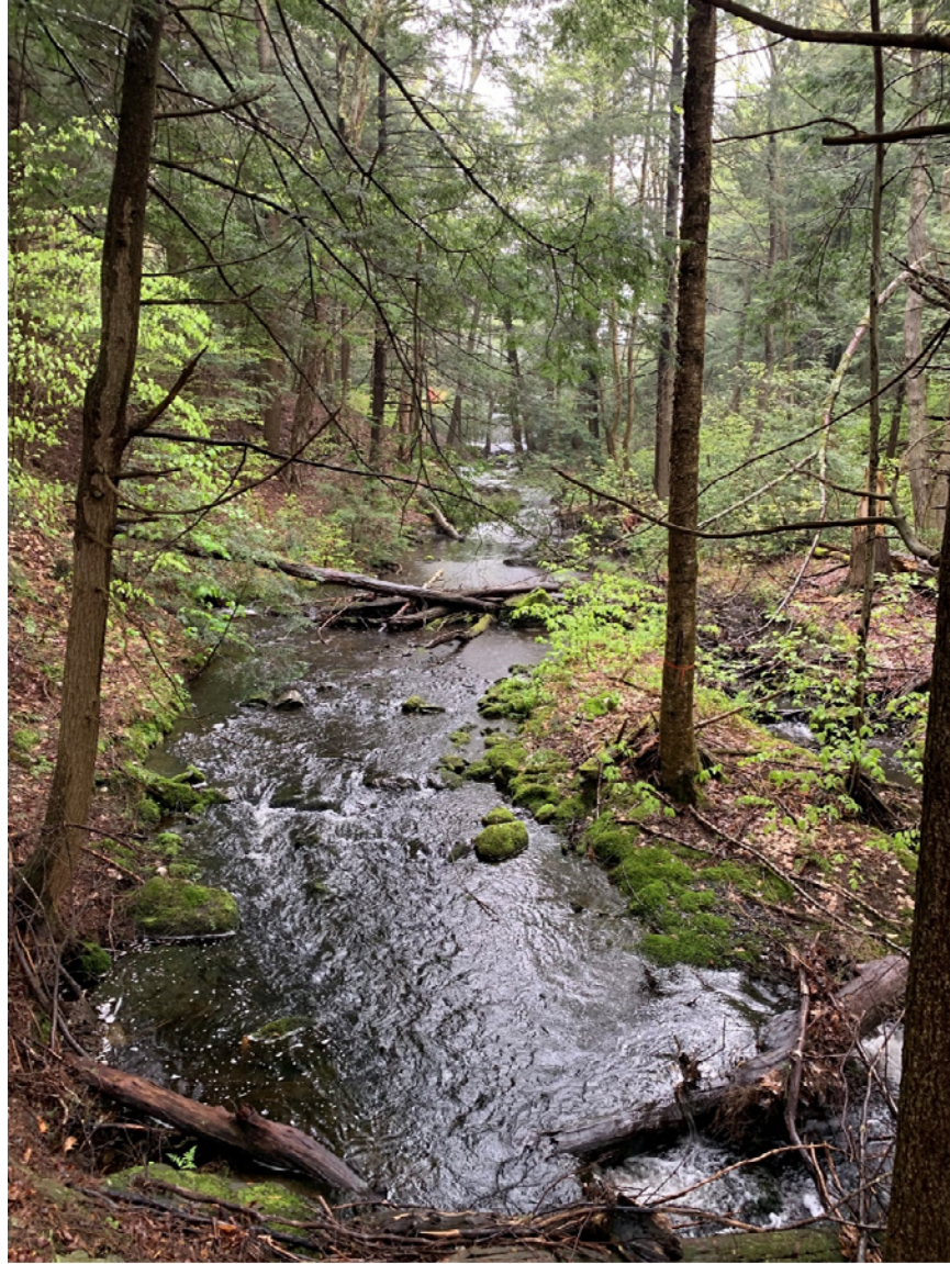
Figure 7. Looking upstream at the reach immediately downstream of the dam
