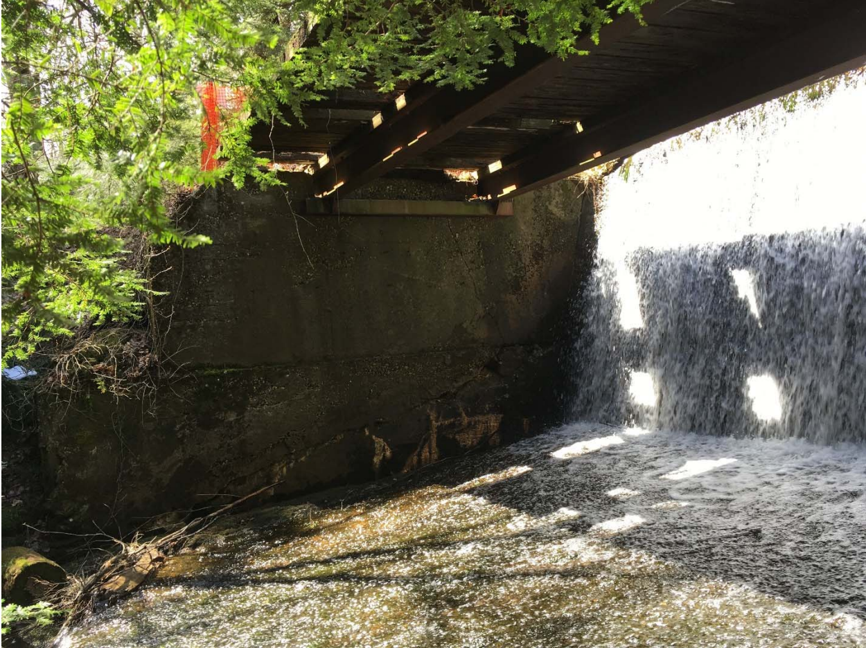
Figure 3. Right concrete training wall and concrete apron
