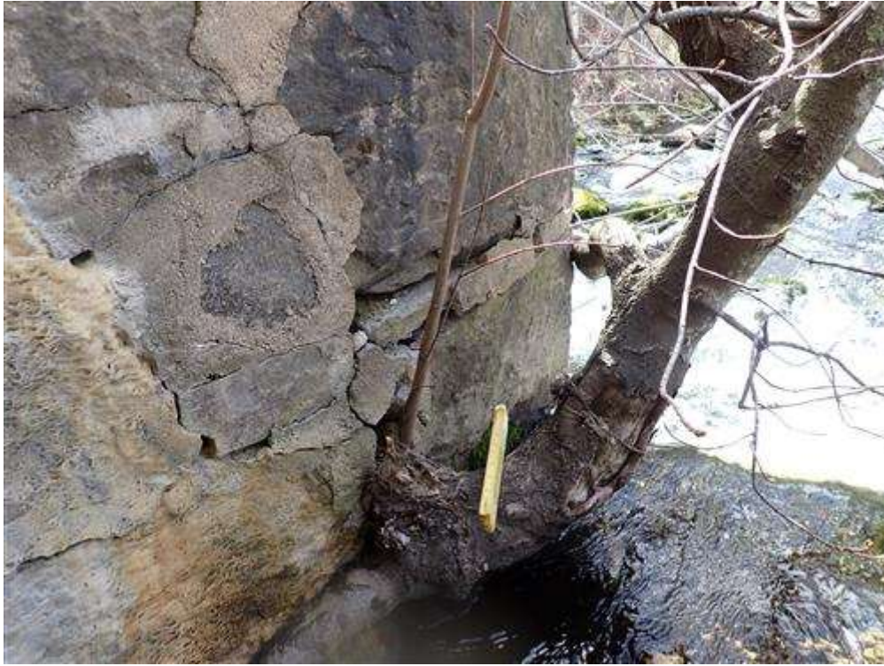
Pier 2 West Downstream Vegetation Growing From Stone
