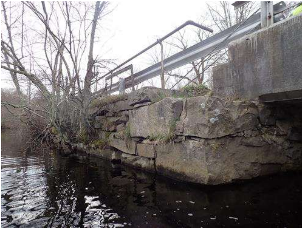
Wingwall 2A and Northeast Retaining Wall
