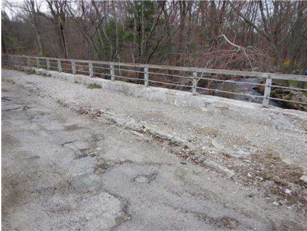
Right (South) Curb, Sidewalk, Parapet and Bridge Rail
