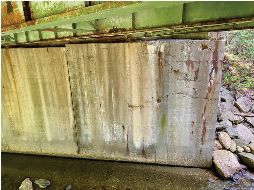
Photo 20: East breastwall at south end.
