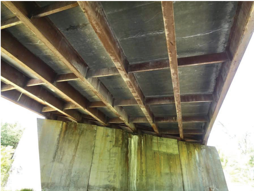
Photo 2: Typical underside, looking west (east span shown).
