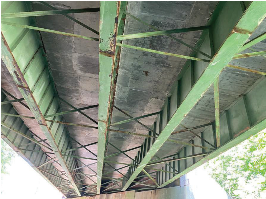
Photo 2: Typical underside, looking west.
