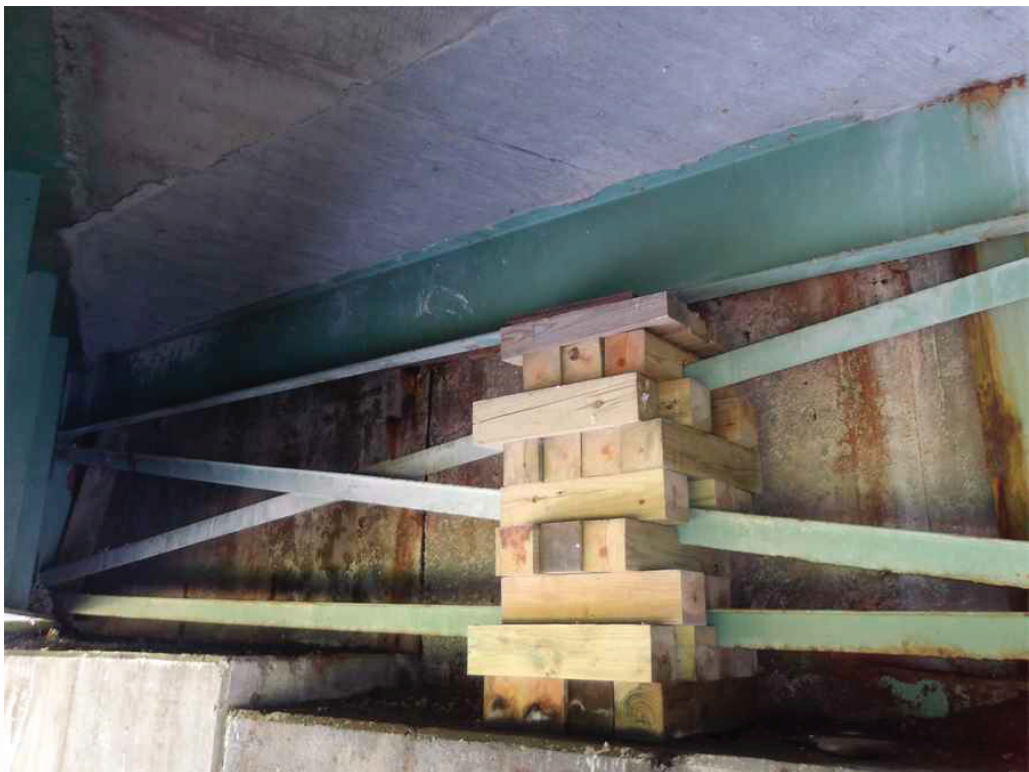
Photo 41: East Abutment below Bay 3, looking northeast. Note the timber cribbing.
