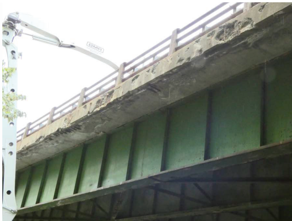
Photo 5: South deck fascia and overhang.
