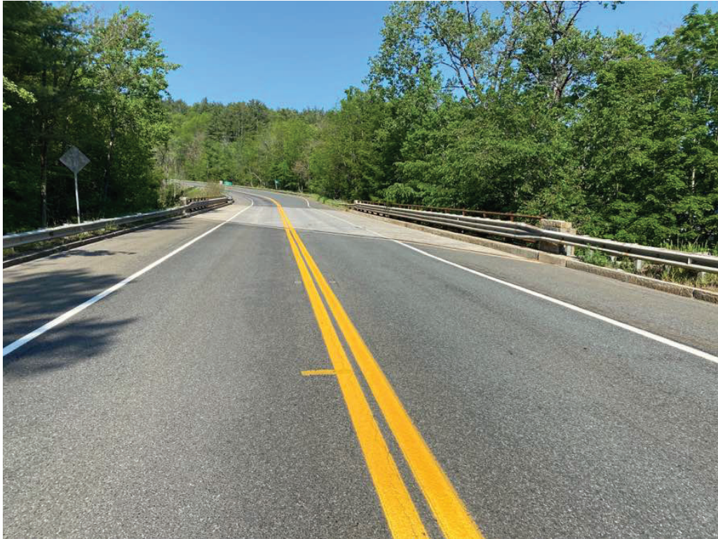
Photo 1: General topside looking west.
