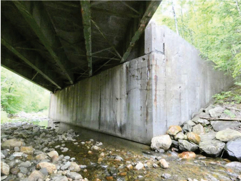
Photo 23: Southeast breastwall, cheekwall and wingwall.
