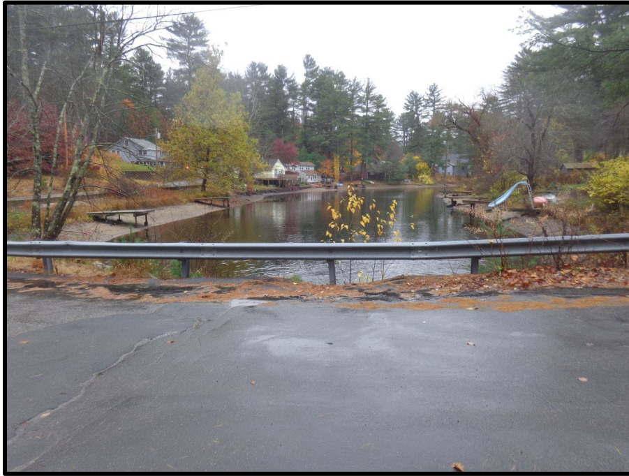
Photograph 7: View downstream of Alden Pond from the bridge.
