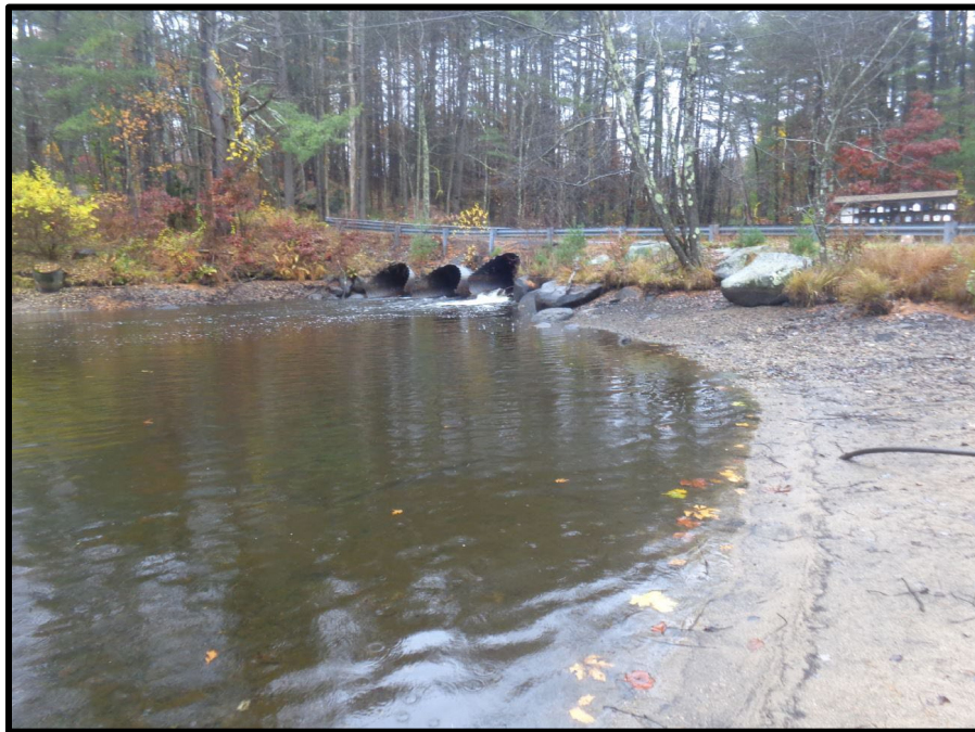
Photograph 10: View upstream showing the outfall structures from Photograph 9.
