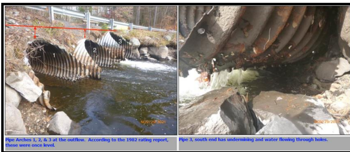
Figure 7-3. Site visit photos
