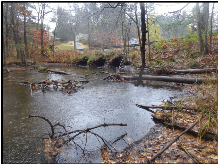
Photograph 6: View southeast of the outfall structures from Photograph 5.
