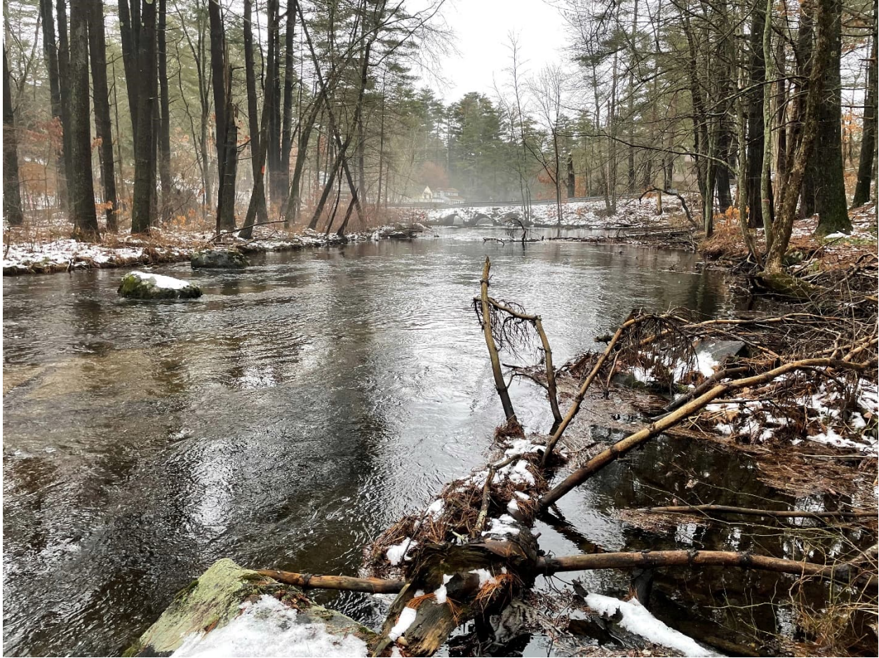
Figure 3: Upstream channel looking downstream at the culvert inlets.
