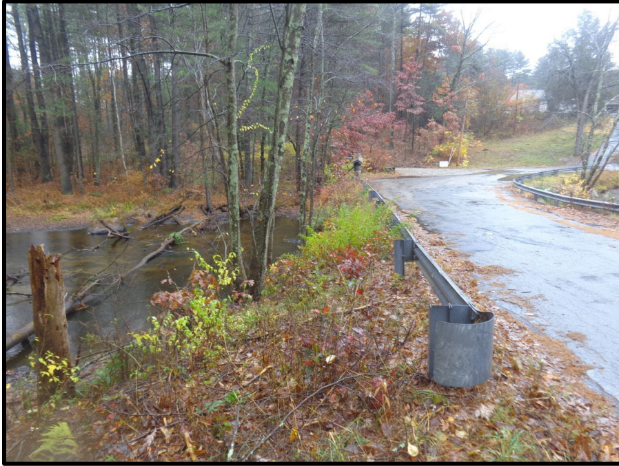
Photograph 1: View east of Piney Lane over Broad Brook.
