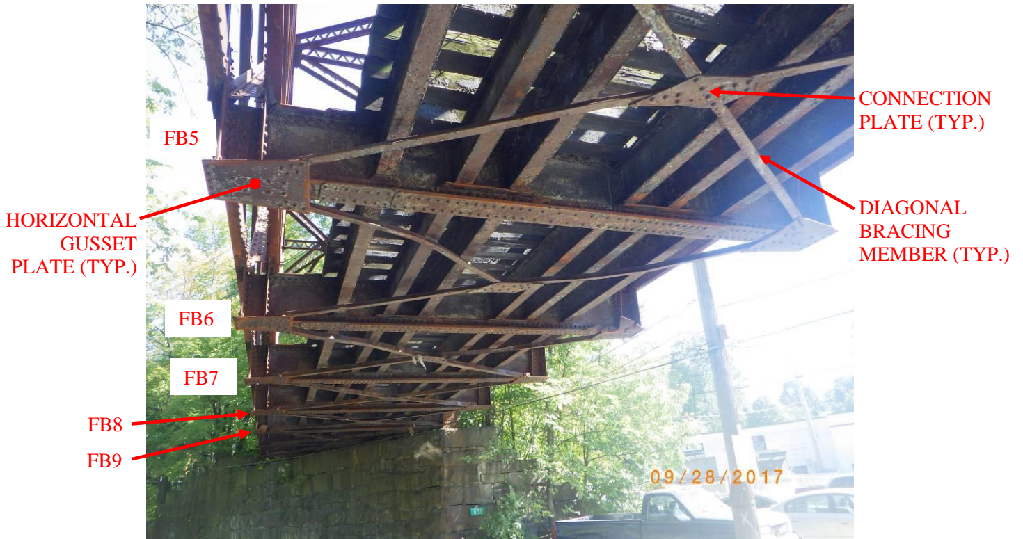
Photo 1: Overall underside view, looking east.
