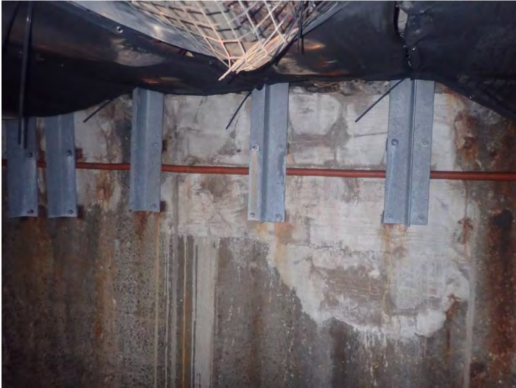
Photo 17: South breastwall/bridge seat repairs between beams #16 and #20
