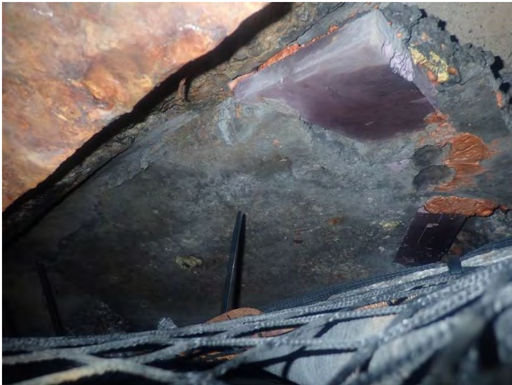
Photo 2: Deck repair between beams #17 and #18
