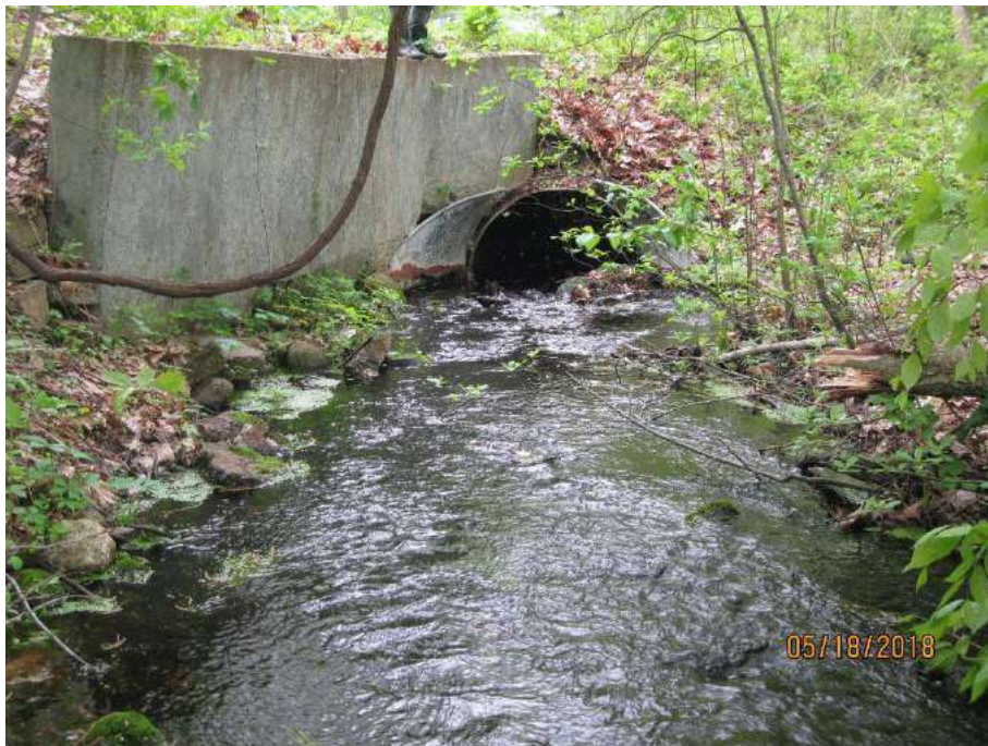
Photo 2: Previous upstream elevation, 05/18/2018
