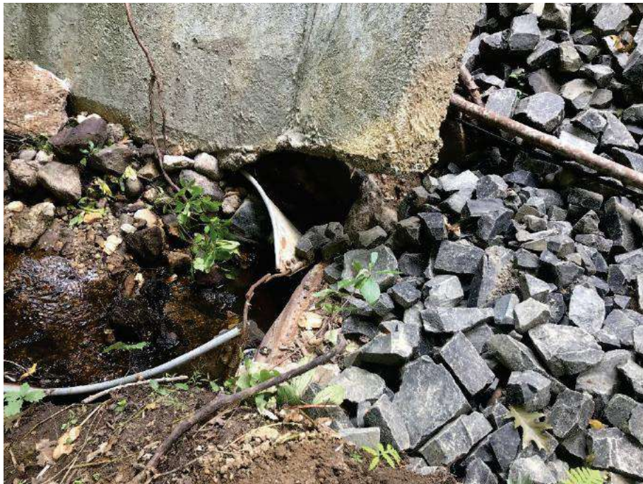
Photo 2: View from top of barrel looking down. 09/17/2021
