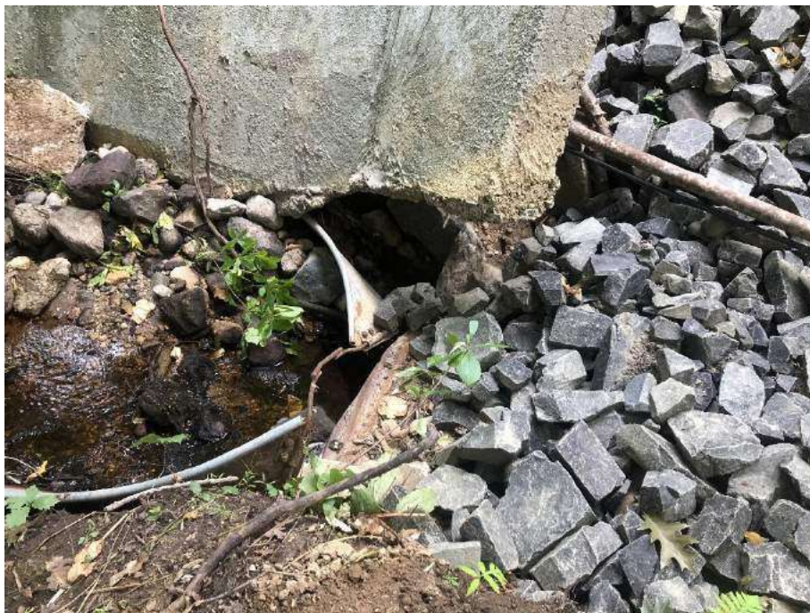
Photo 2: View from top of barrel looking down. 09/17/2021
