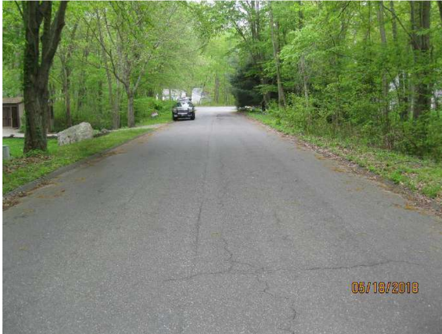
Photo 1: Previous Southbound approach, 05/18/2018
