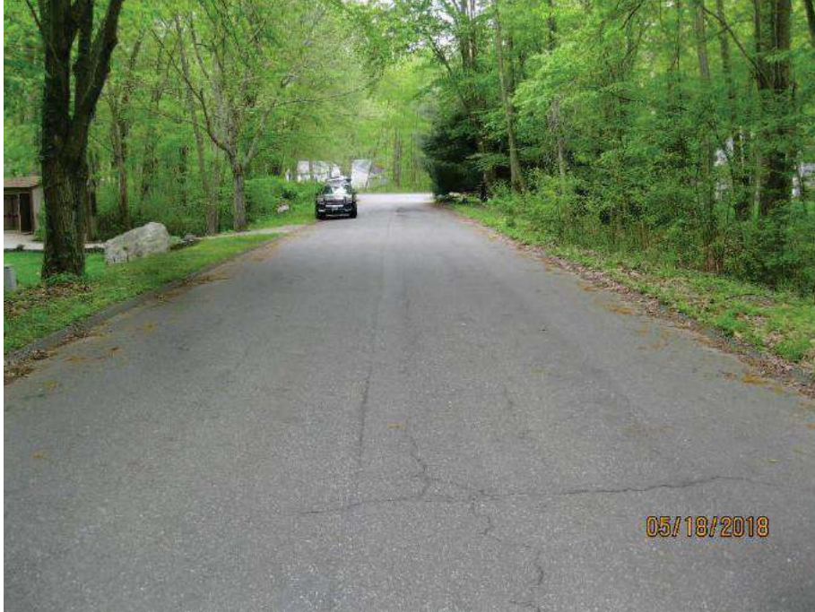
Photo 1: Previous Southbound approach, 05/18/2018
