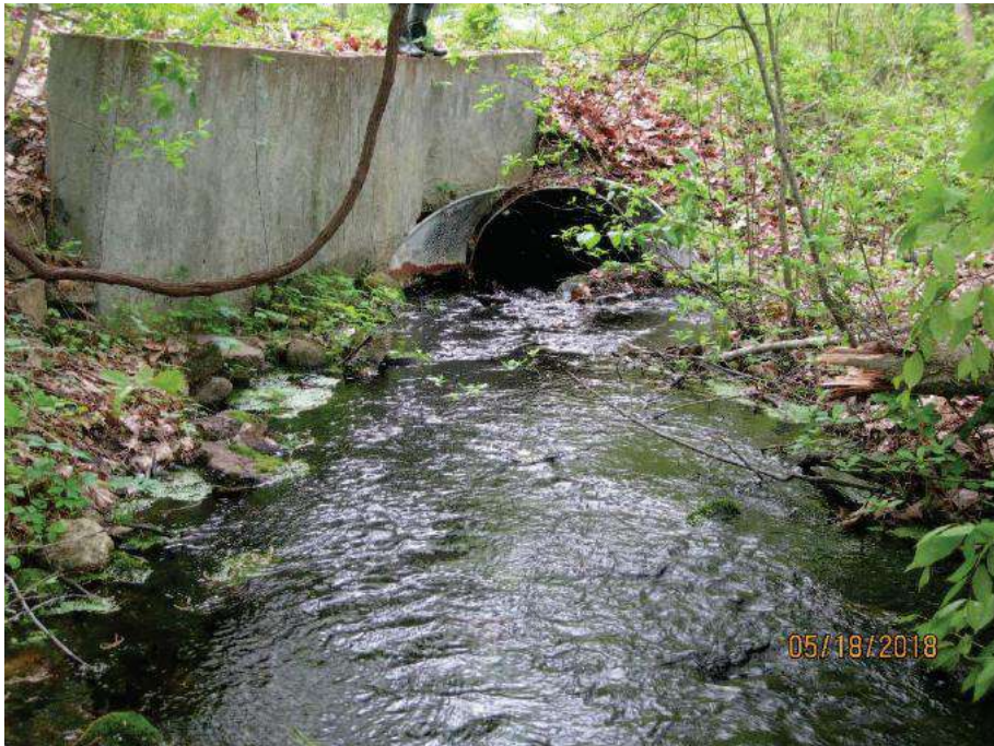
Photo 2: Previous upstream elevation, 05/18/2018
