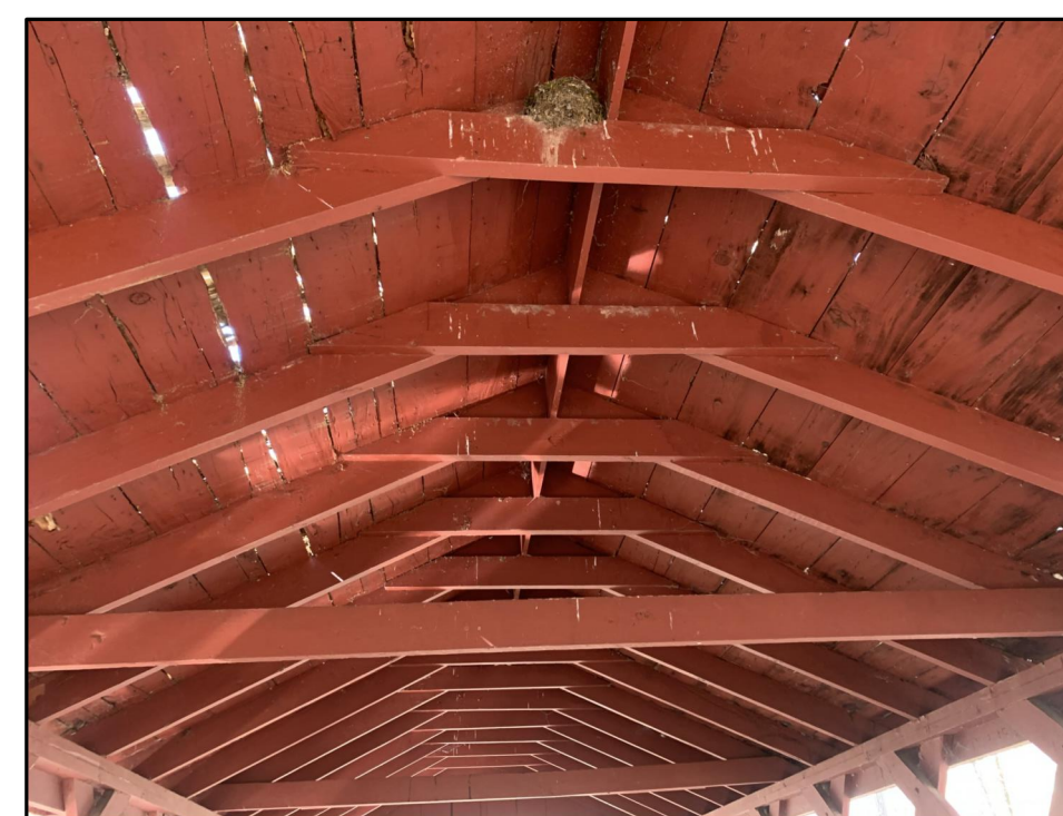
3 S3.0 PREVIOUS BRIDGE CEILING
