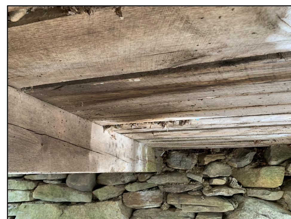
10 S3.0 PREVIOUS BRIDGE UNDERNEATH
