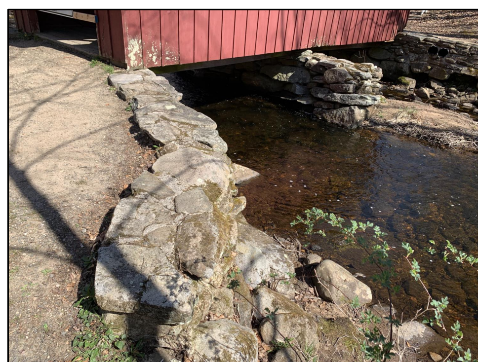
9 S3.0 PREVIOUS BRIDGE ABUTMENTS
