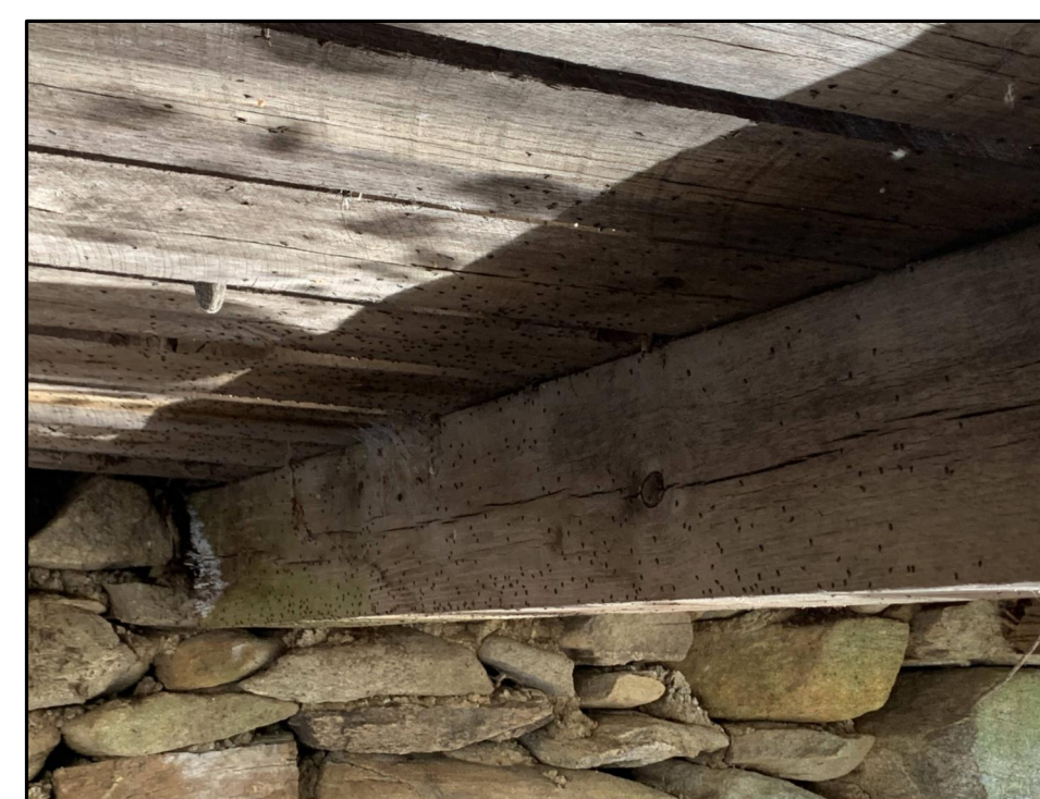
11 S3.0 PREVIOUS BRIDGE SUPPORT BEAM
