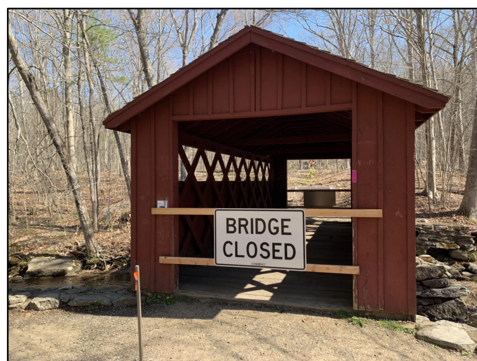
1 S3.0 PREVIOUS BRIDGE SOUTHWEST OPENING
