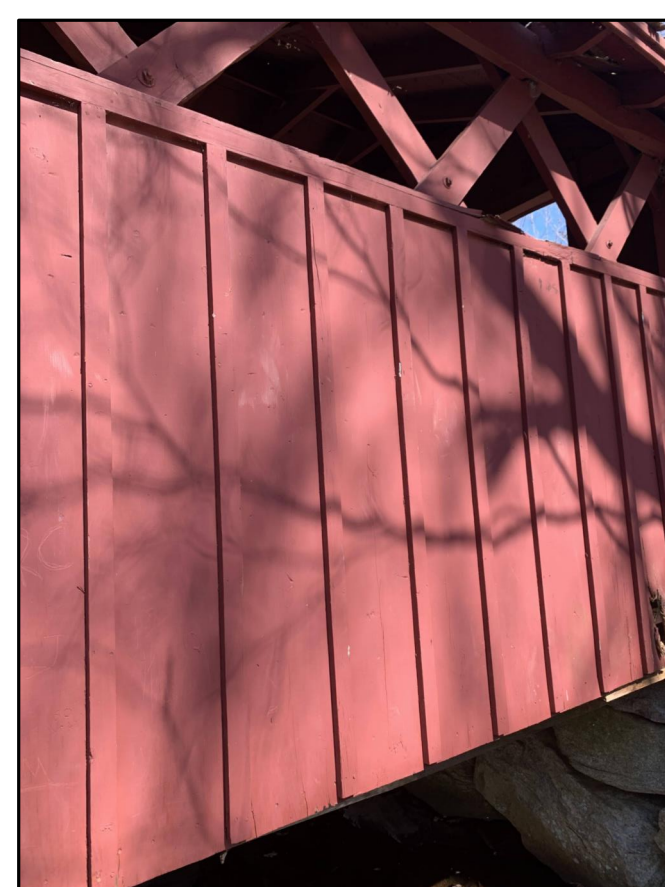
6 S3.0 PREVIOUS BRIDGE SIDING
