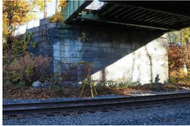
North Abutment, showing general condition of the abutment.
