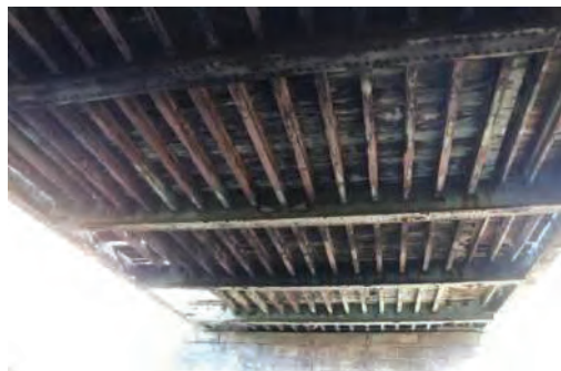
View of the underside of the bridge.
