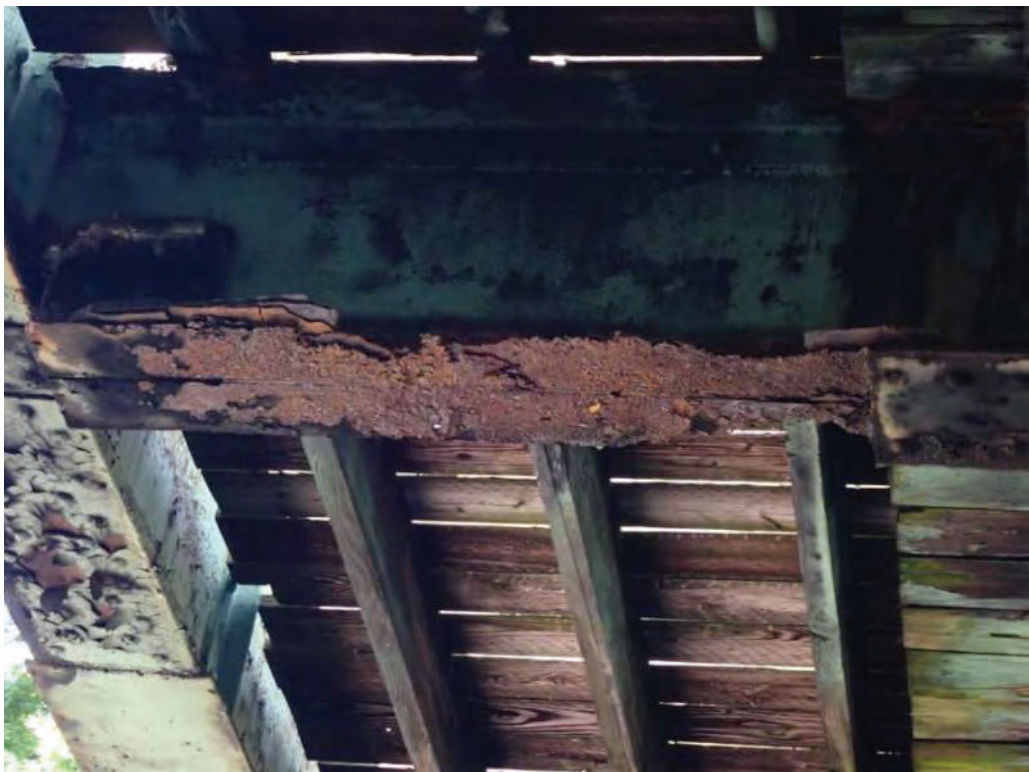
Photo 1: West end of floor beam #2.
