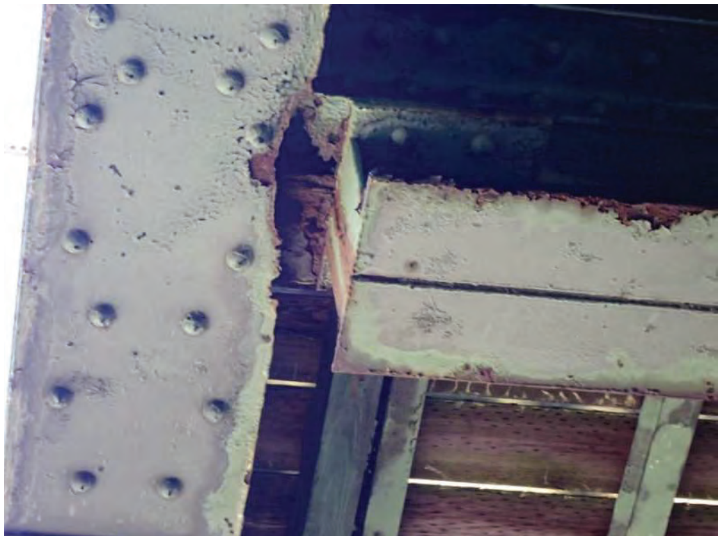
Photo 6: Girder #1 at floorbeam #1.
