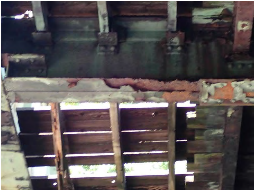
Photo 3: West end of floorbeam #3.
