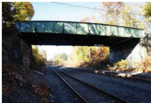
East elevation of the bridge.
