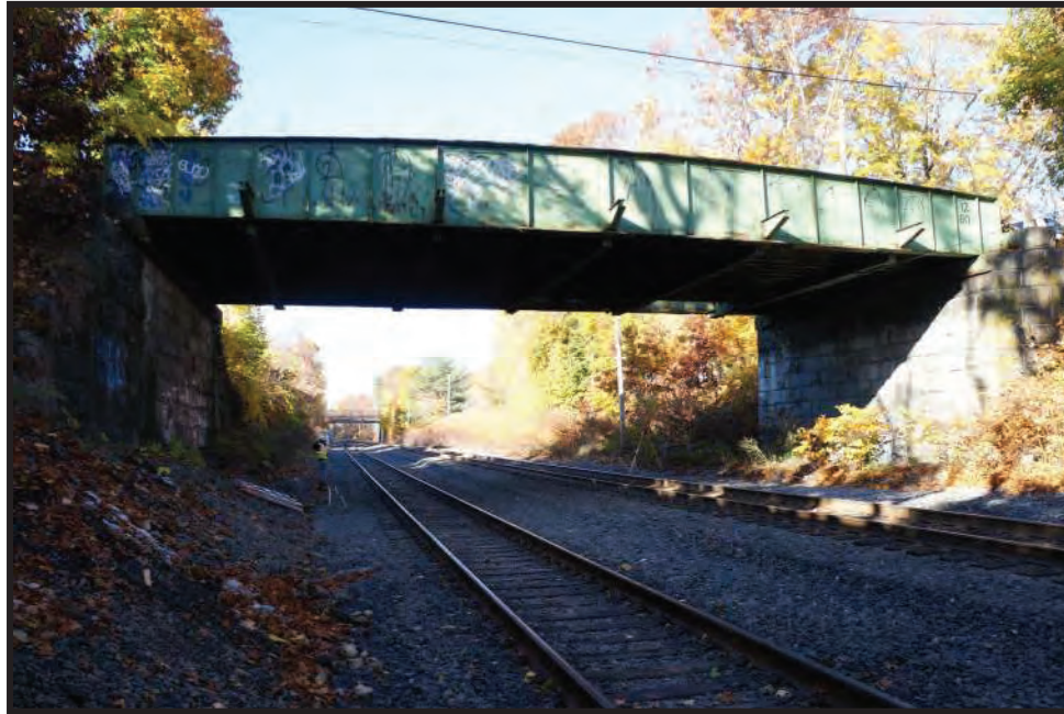
Photo 1: East elevation of the bridge, looking West.
