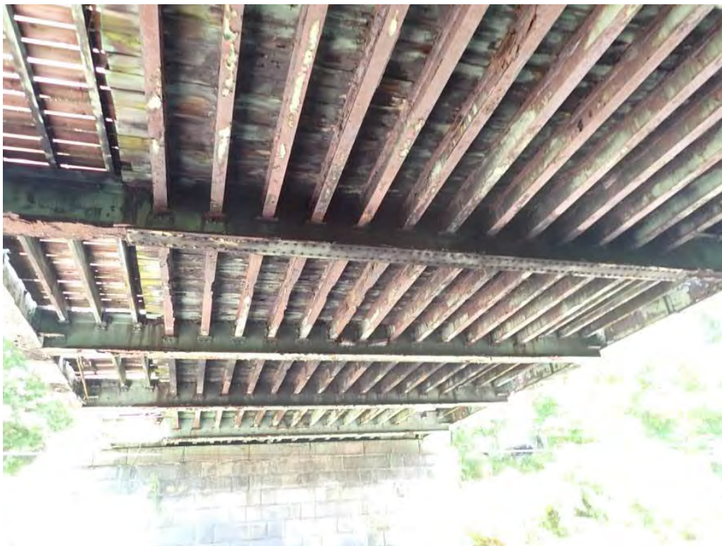
Photo 6: Underside, looking north.
