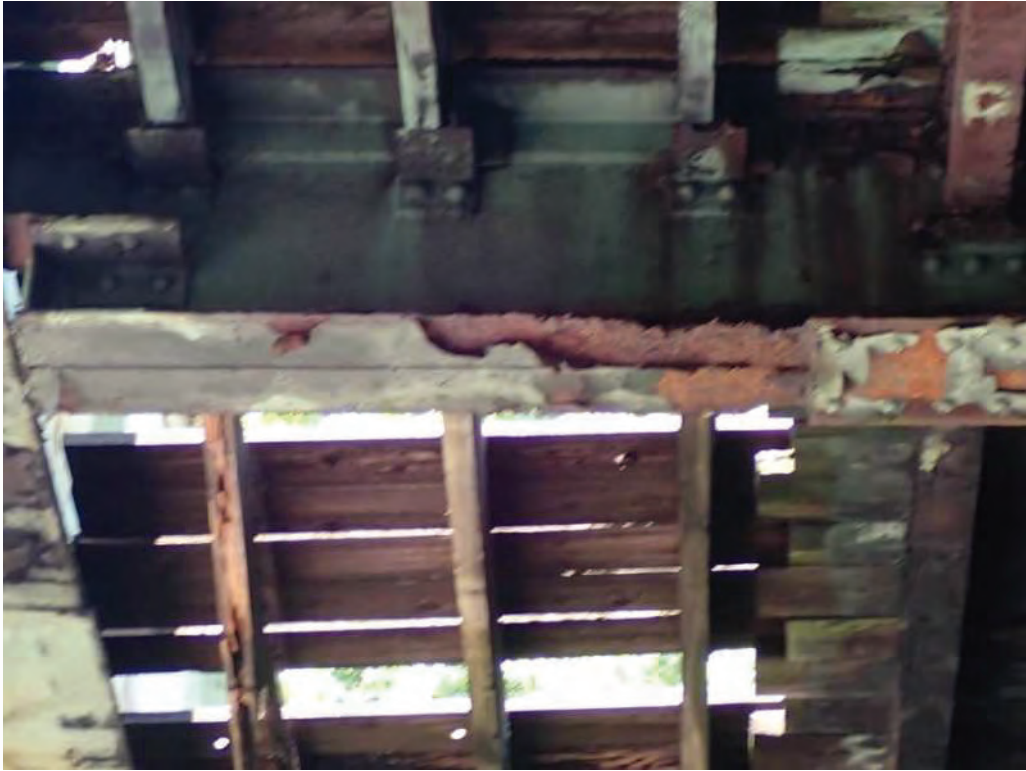
Photo 3: West end of floorbeam #3.
