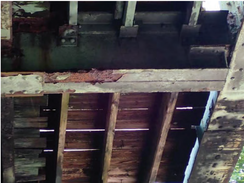
Photo 4: East end of floorbeam #3.
