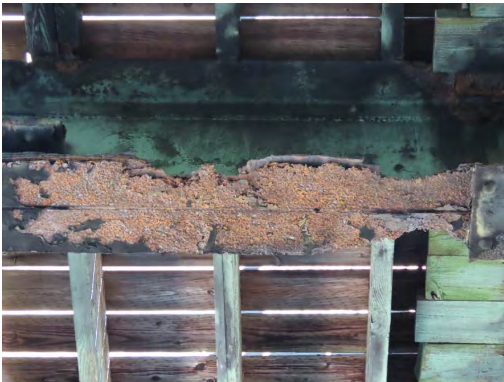
Photo 1: West end of floorbeam #2.
