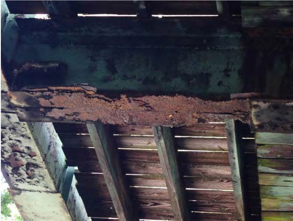
Photo 1: West end of floor beam #2.
