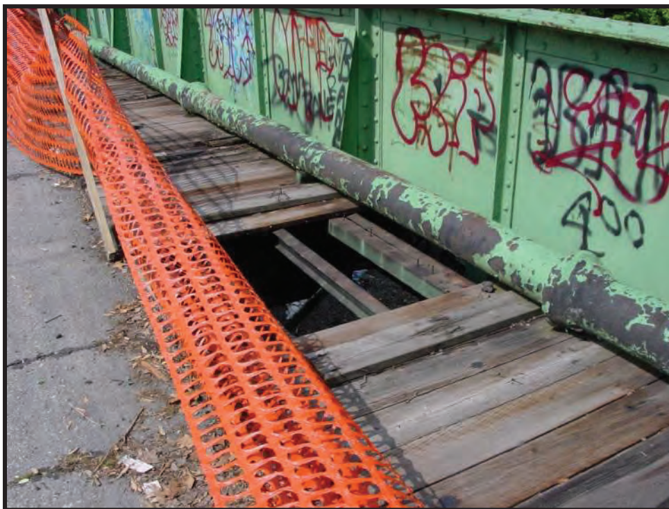
Photo 7: Water utility attached to the top of the East sidewalk (photo from 2001), looking Northeast.
