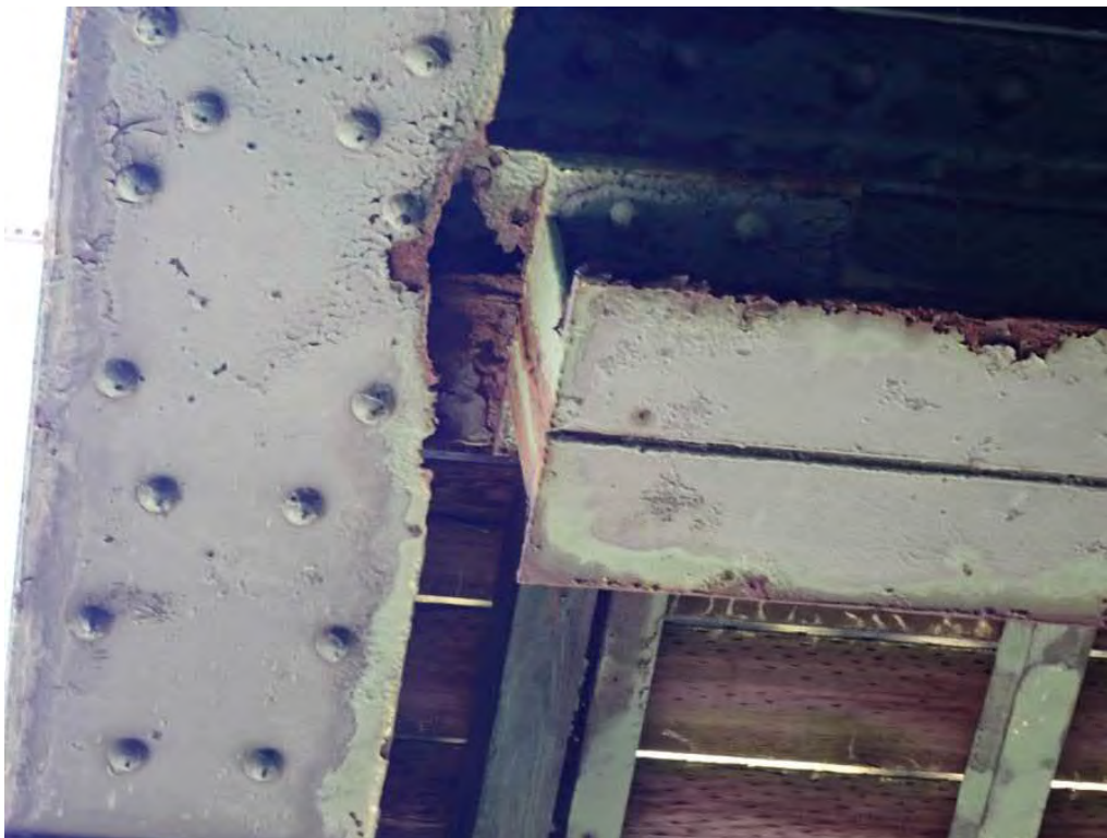
Photo 6: Girder #1 at floorbeam #1.
