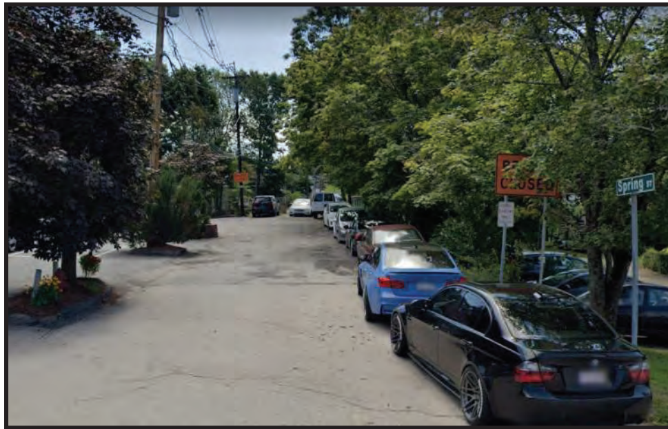
Photo 3: North approach roadway leading up to the bridge, looking South.
