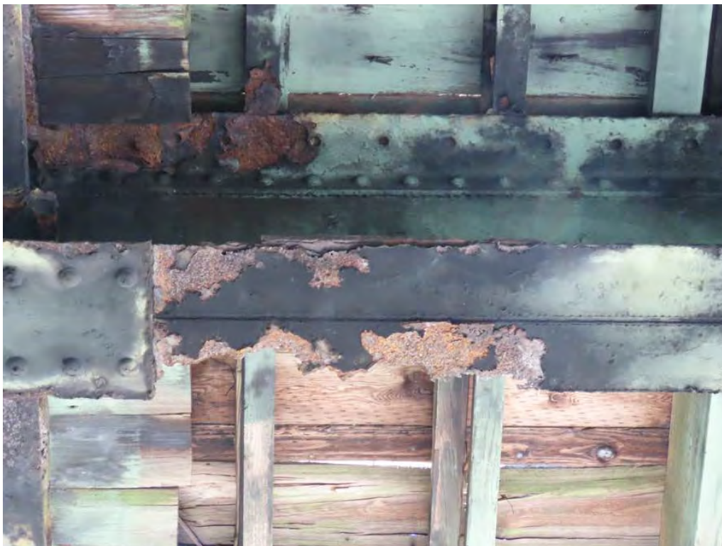
Photo 2: East end of floorbeam #2.
