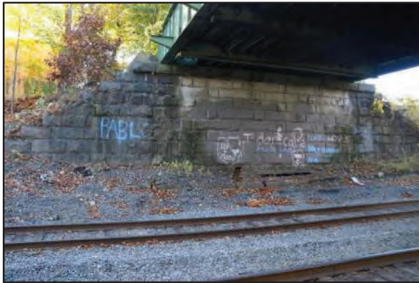
South Abutment, showing general condition of the abutment and wingwalls.
