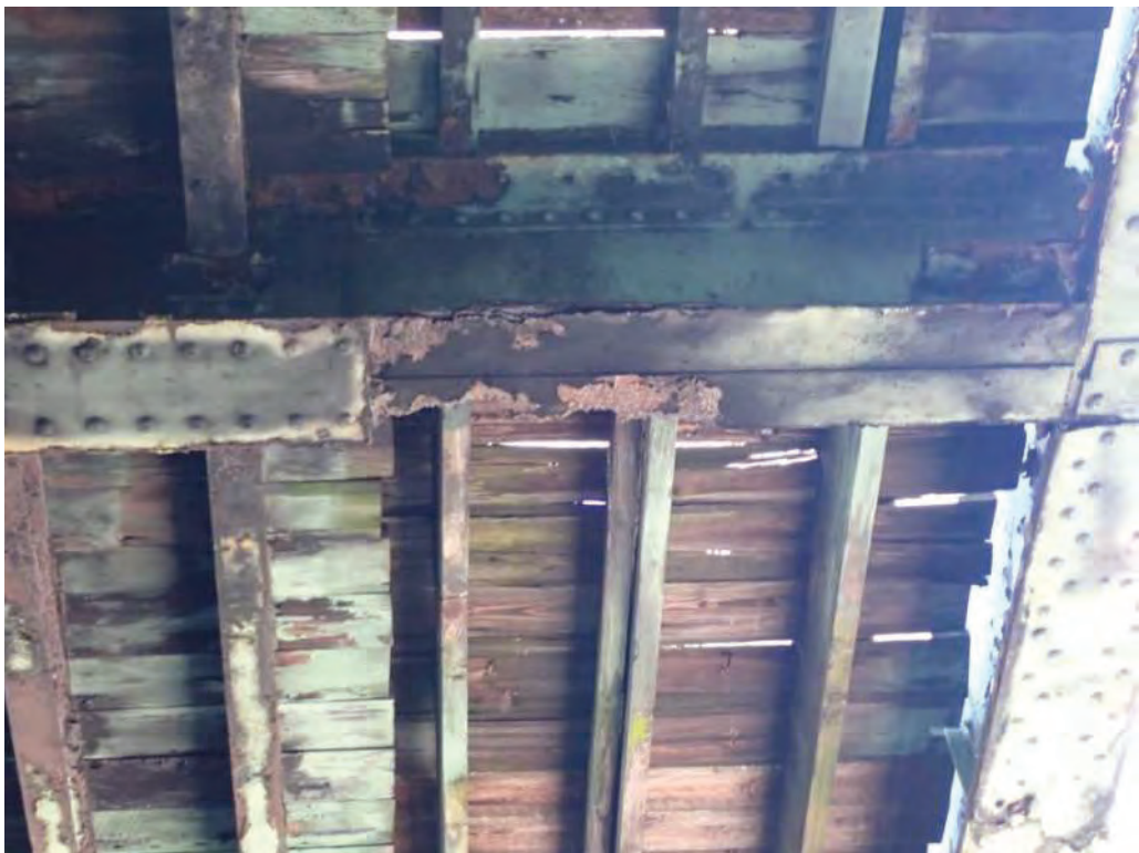
Photo 2: East end of floorbeam #2.
