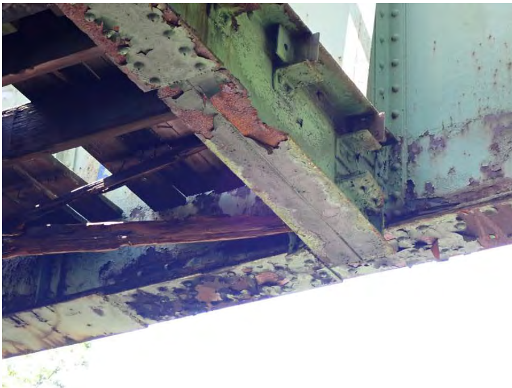
Photo 5: West end of floorbeam #4.
