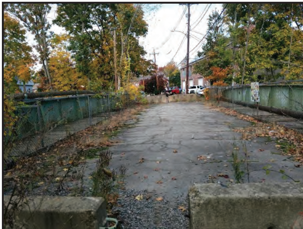
Photo 4: Roadway over the bridge, looking North.
