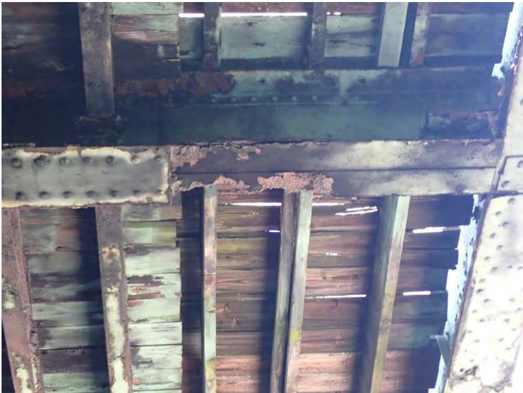
Photo 2: East end of floorbeam #2.
