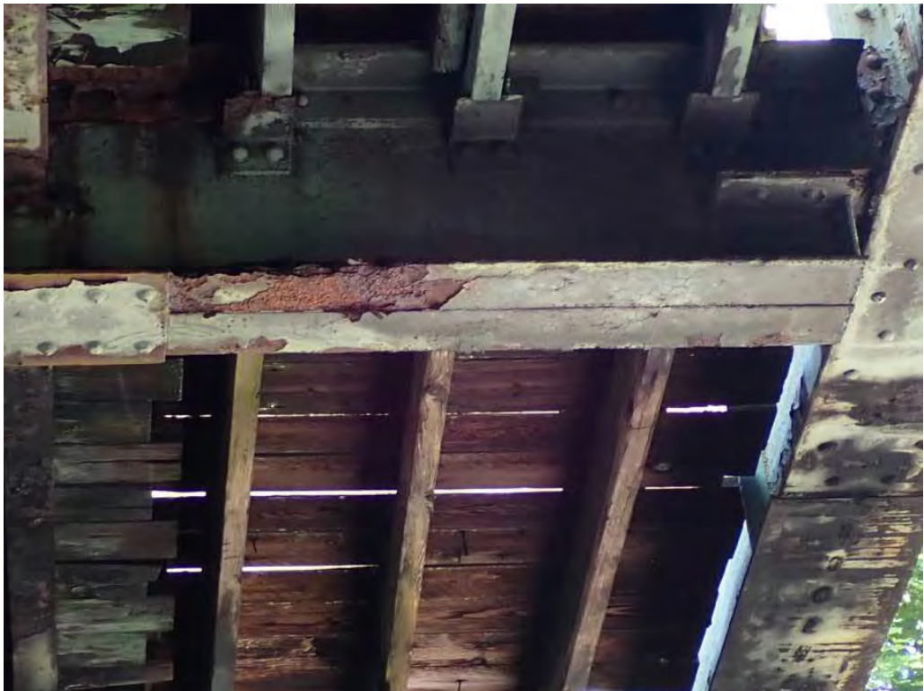
Photo 4: East end of floorbeam #3.
