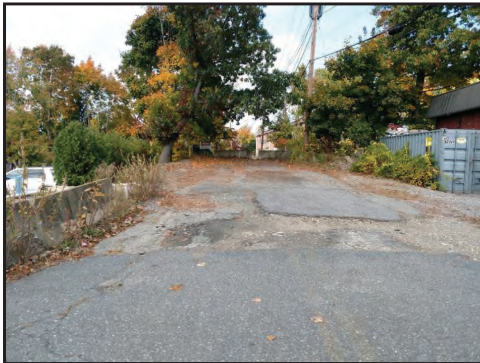
Photo 2: South approach roadway leading up to the bridge, looking North.
