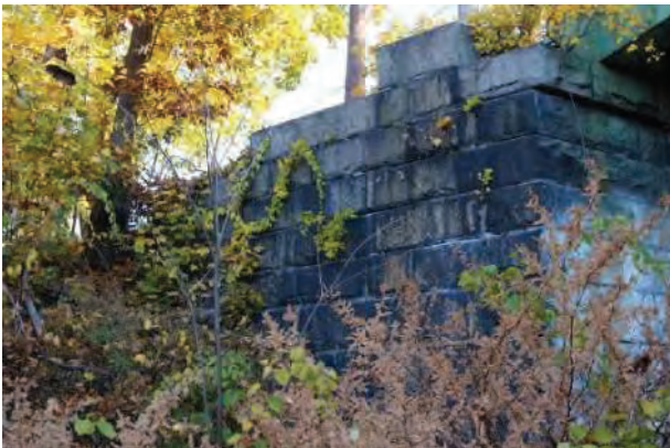
Typical condition of the North Abutment Wingwalls.
