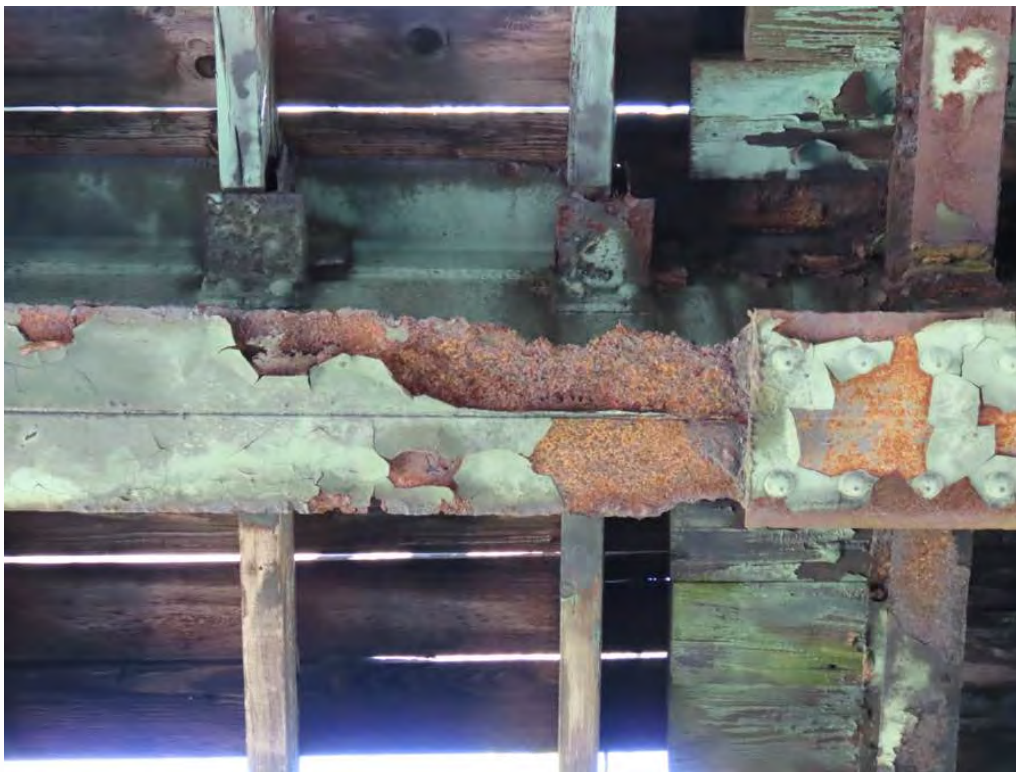
Photo 3: West end of floorbeam #3.
