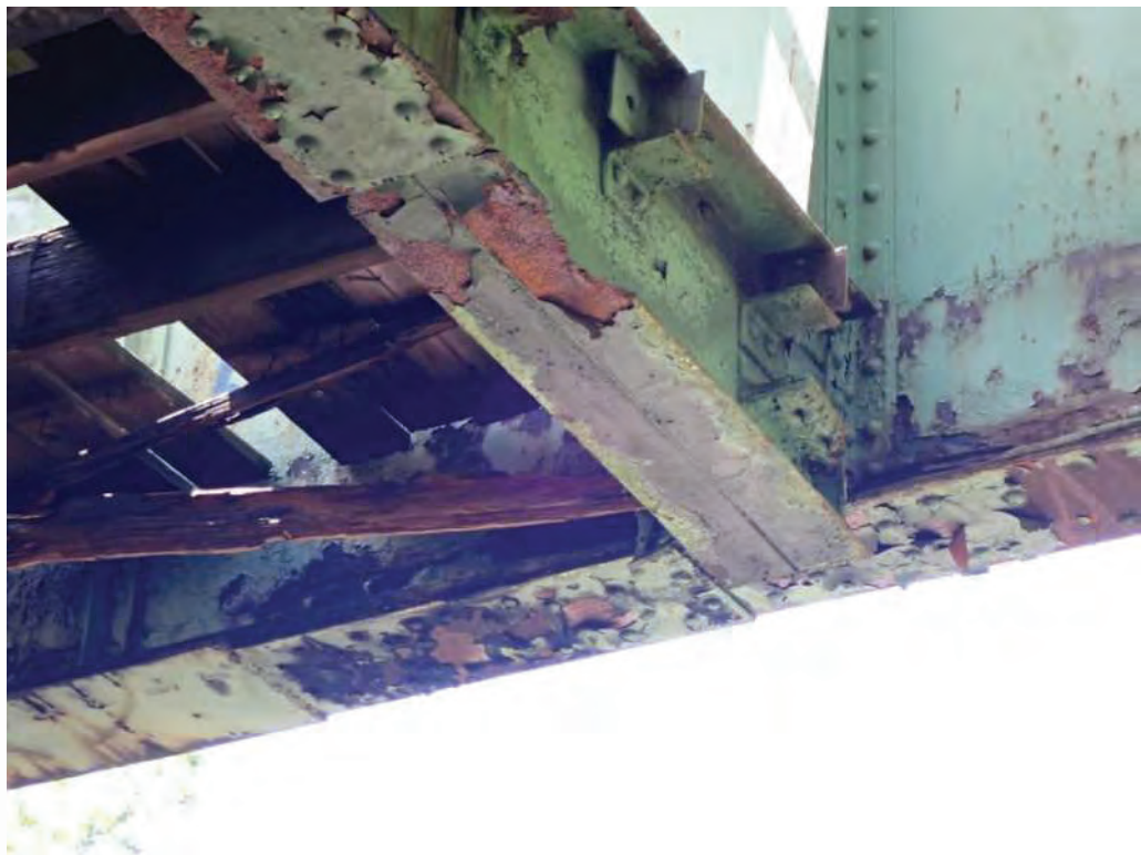
Photo 5: West end of floorbeam #4.
