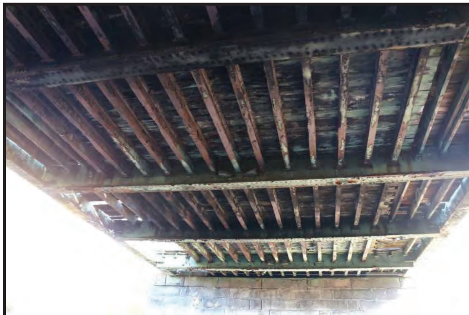
Photo 5: Typical condition of the underside of the bridge, looking North
