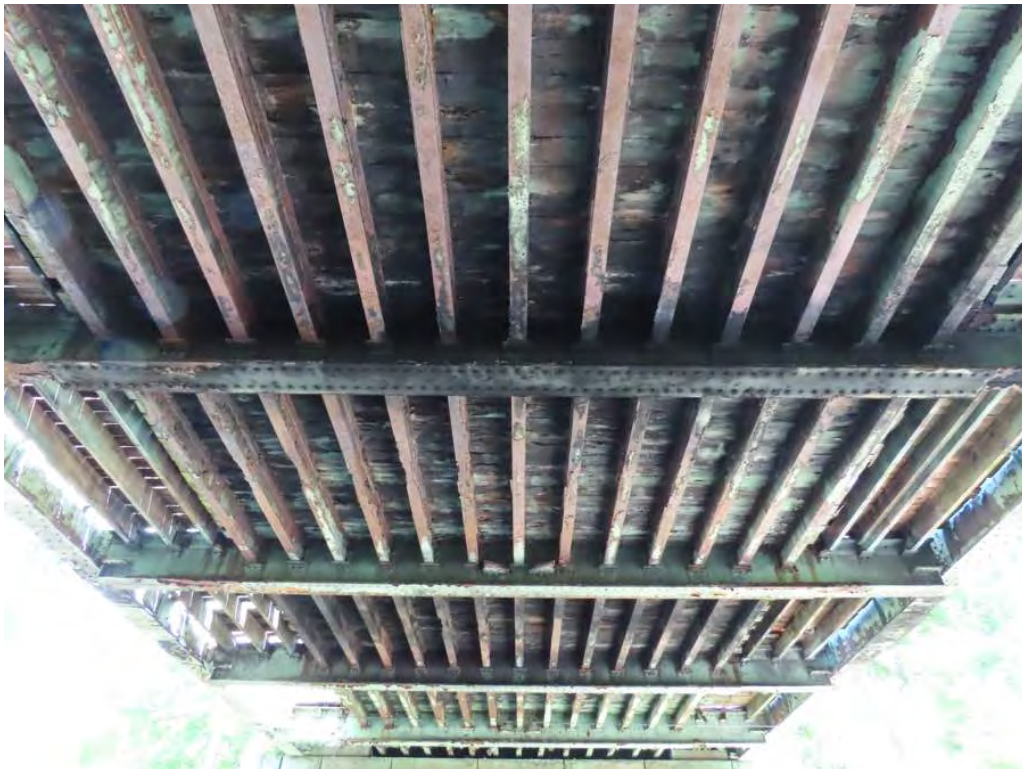
Photo 6: Underside looking North.
