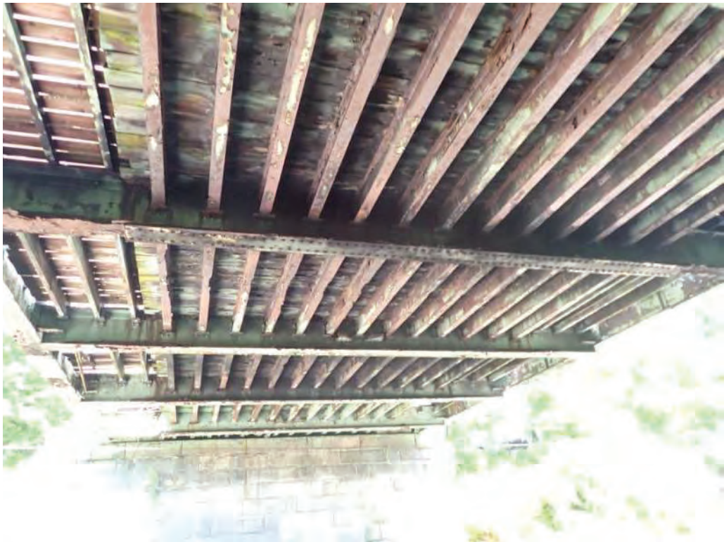
Photo 6: Underside, looking north.
