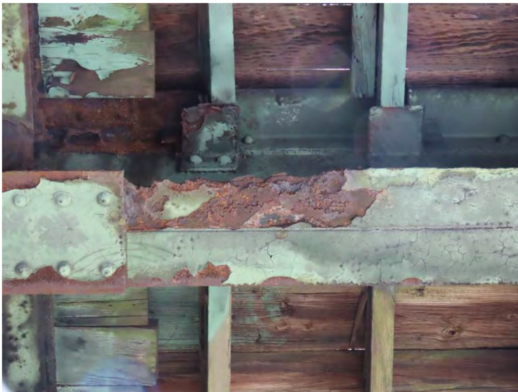
Photo 4: East end of floorbeam #3.
