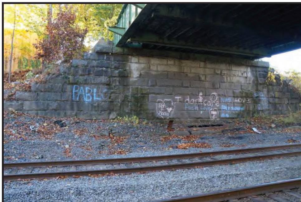
Photo 6: Typical condition of the abutments (South Abutment shown), looking South.
