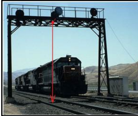
Figure 11 – Bidirectional Signal Bridge
