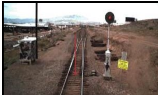
Figure 17 – Point of Switch – Slip Switch
