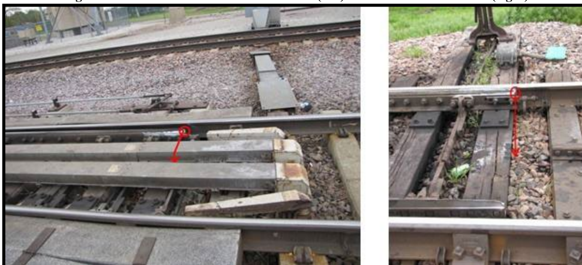
Figure 14 – Point of Switch – Power Switch (left) & Hand Thrown Switch (right)
