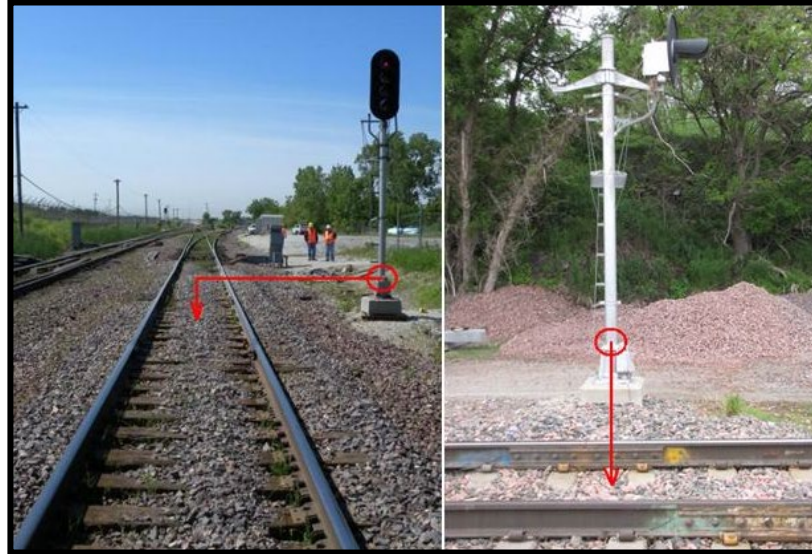
Figure 5 – High Stand Signal (unidirectional)
