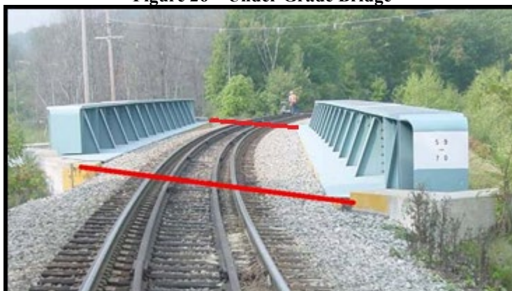
Figure 26 – Under Grade Bridge
