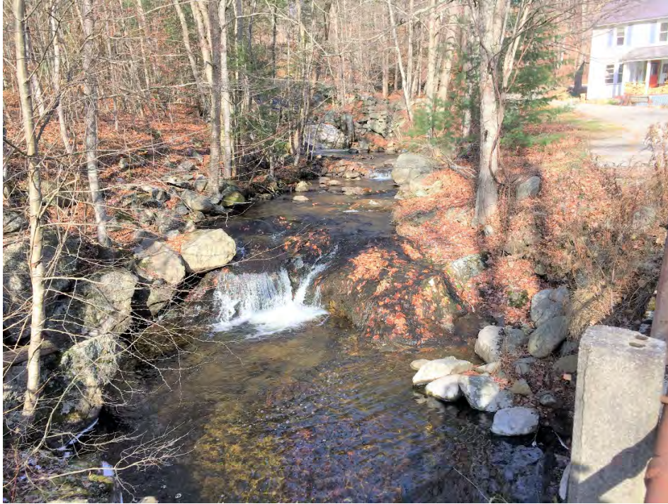
Looking upstream from bridge
