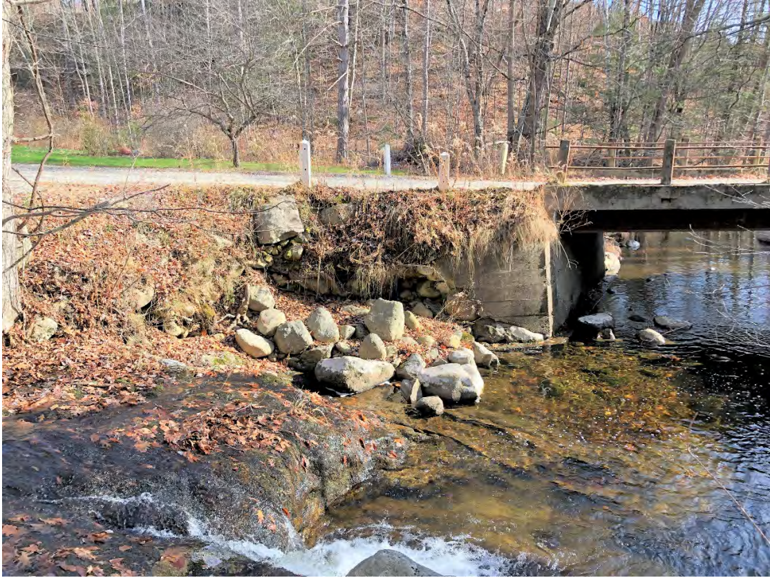
Northwest bridge quadrant
