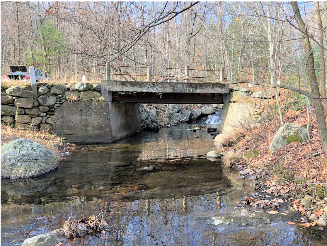
Looking upstream at bridge (looking west)
