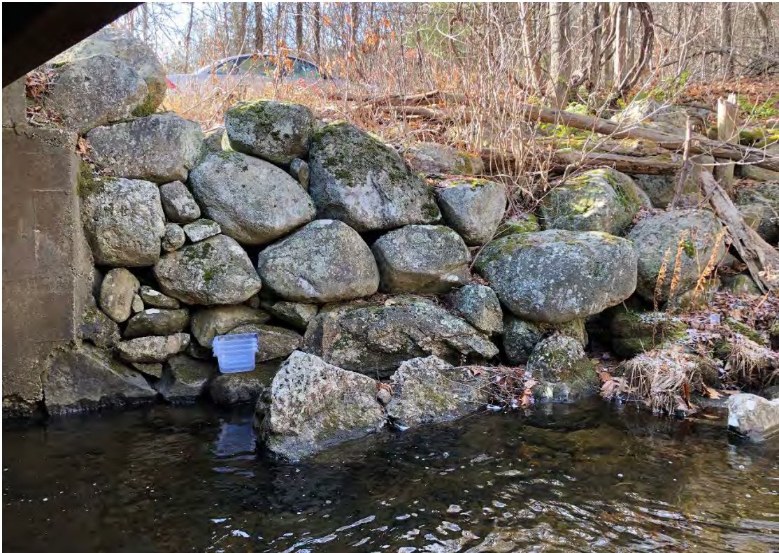
Southwest bridge quadrant
