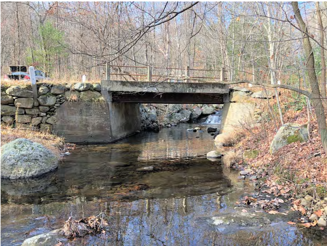
Looking upstream at bridge (looking west)
