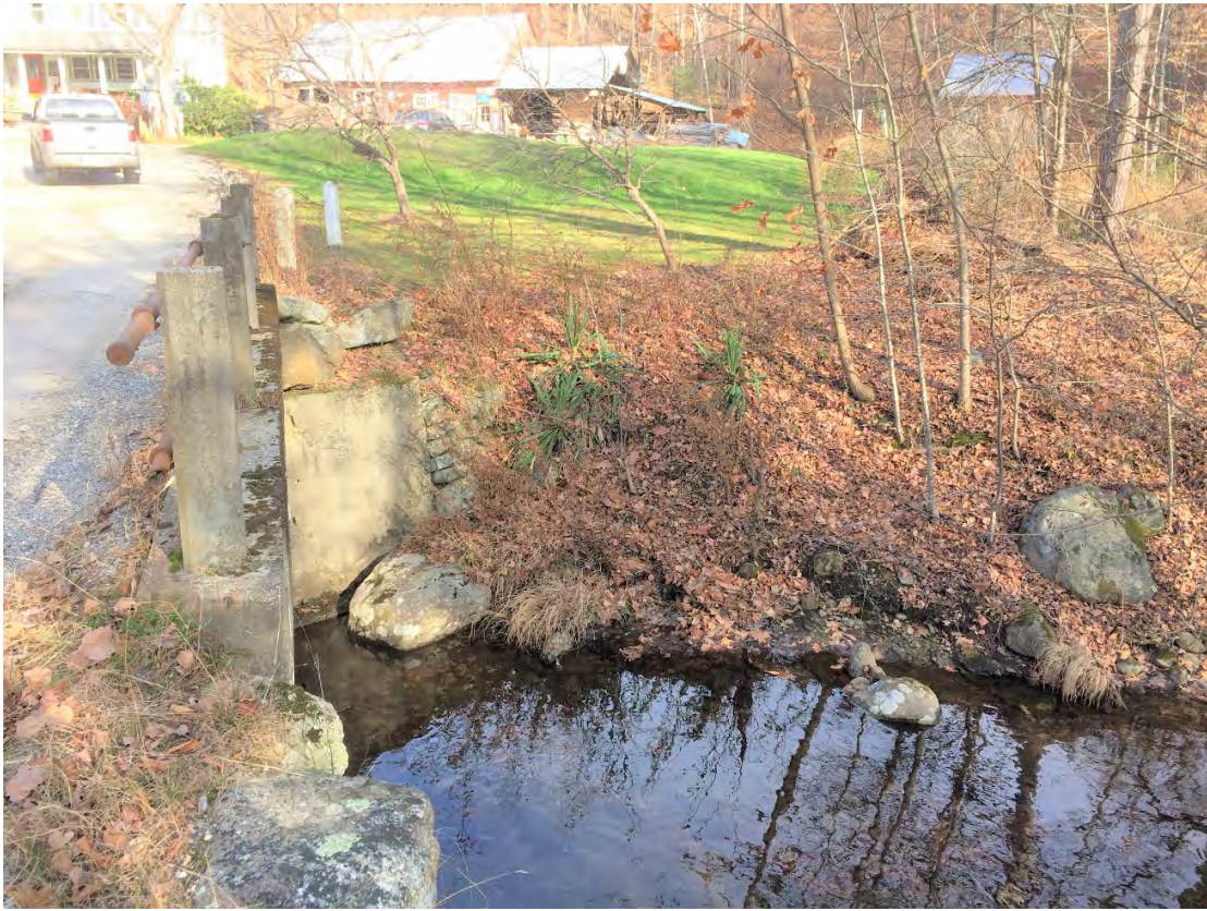
Northeast bridge quadrant
