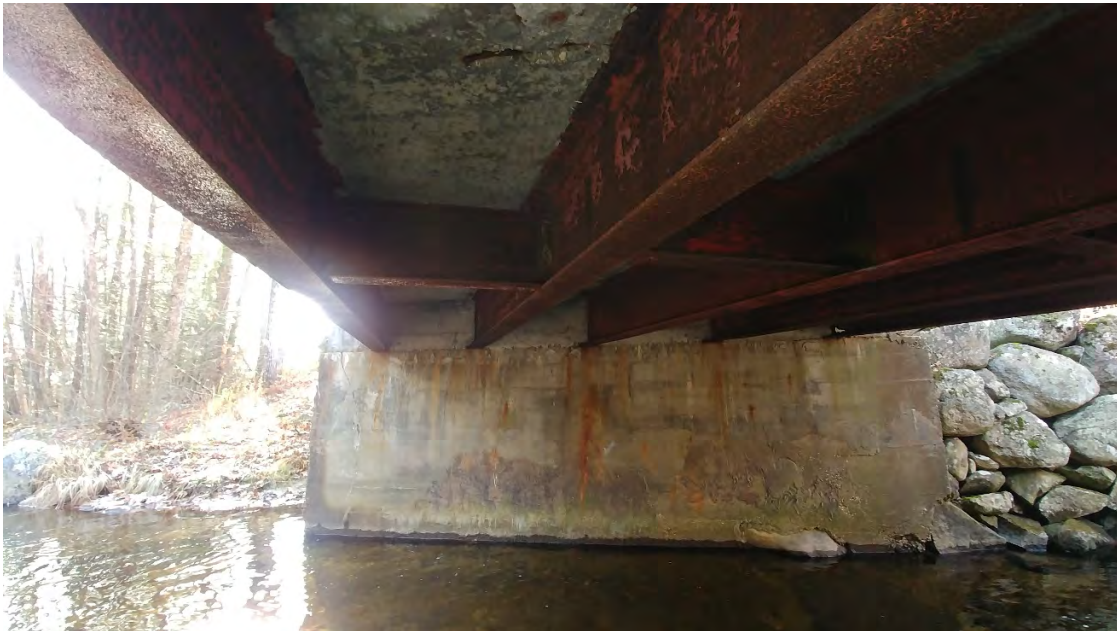
Southerly abutment wall
