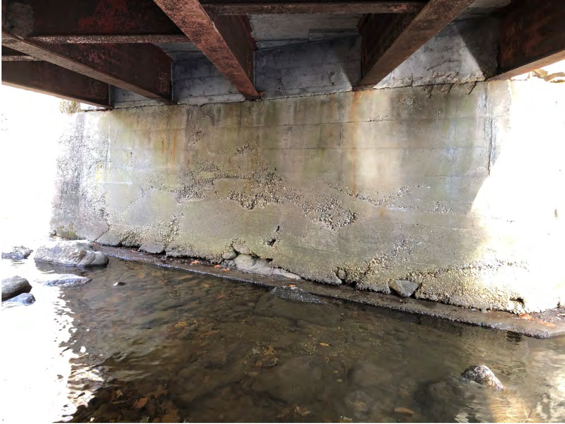
Northerly abutment wall
