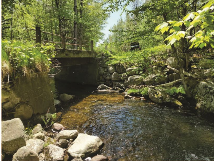
Figure 8: Upstream Face of the Existing Bridge
