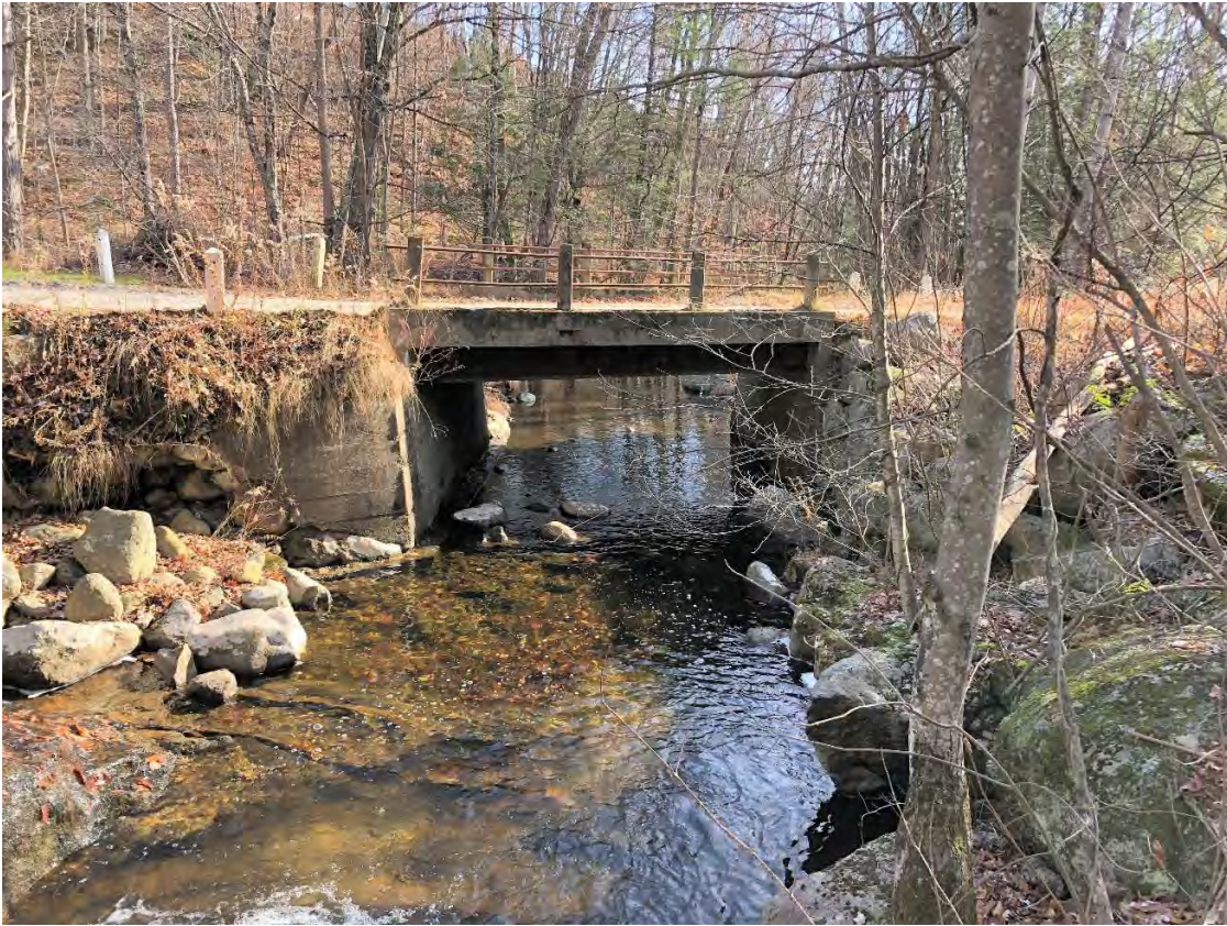
Looking downstream at bridge (looking east)
