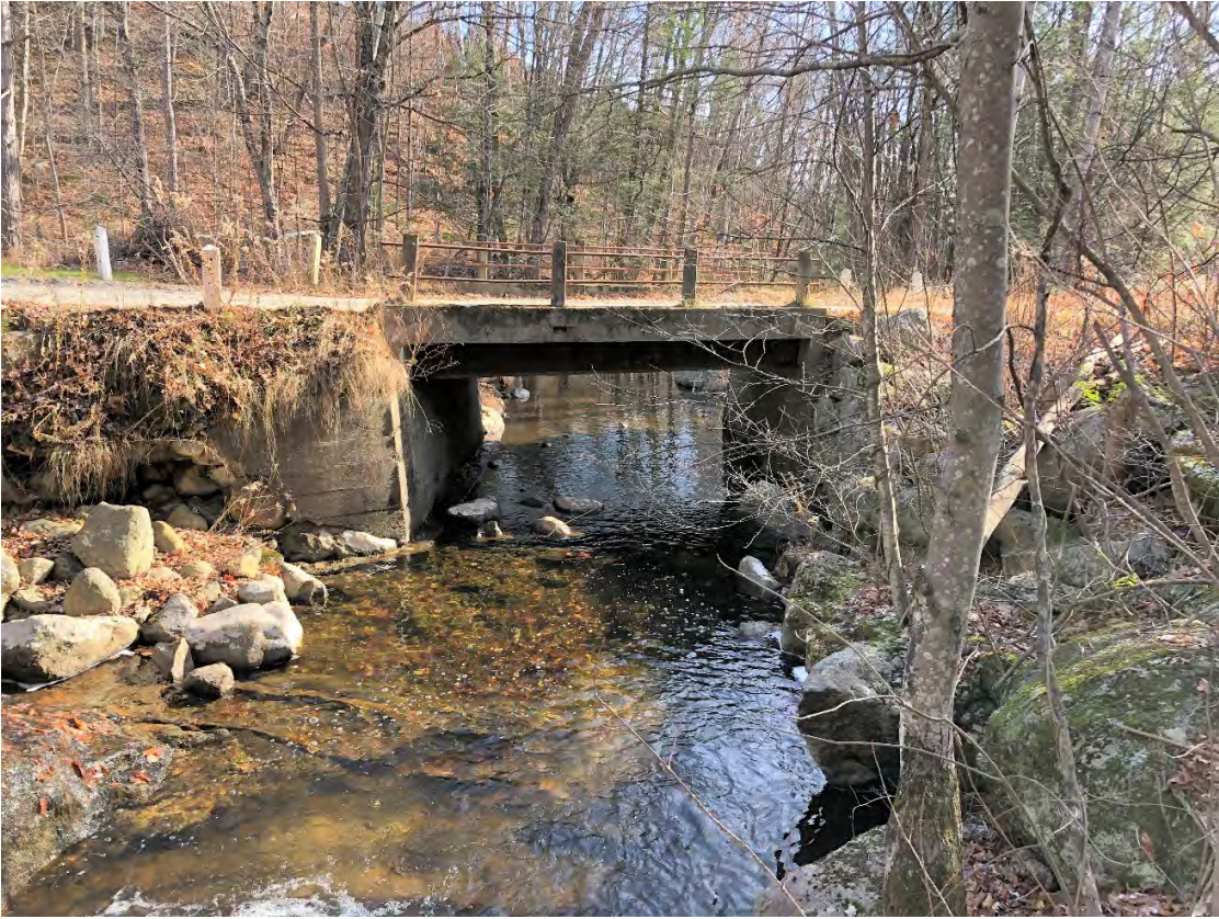
Looking downstream at bridge (looking east)
