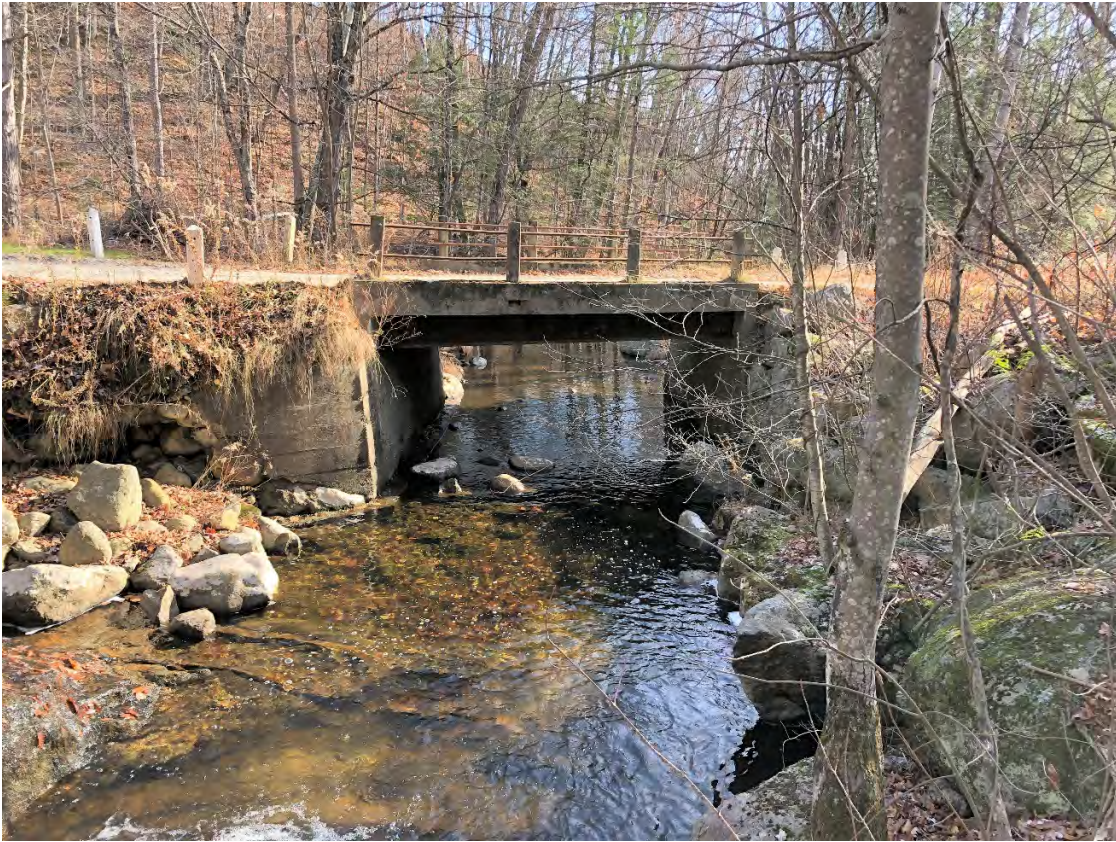
Looking downstream at bridge (looking east)
