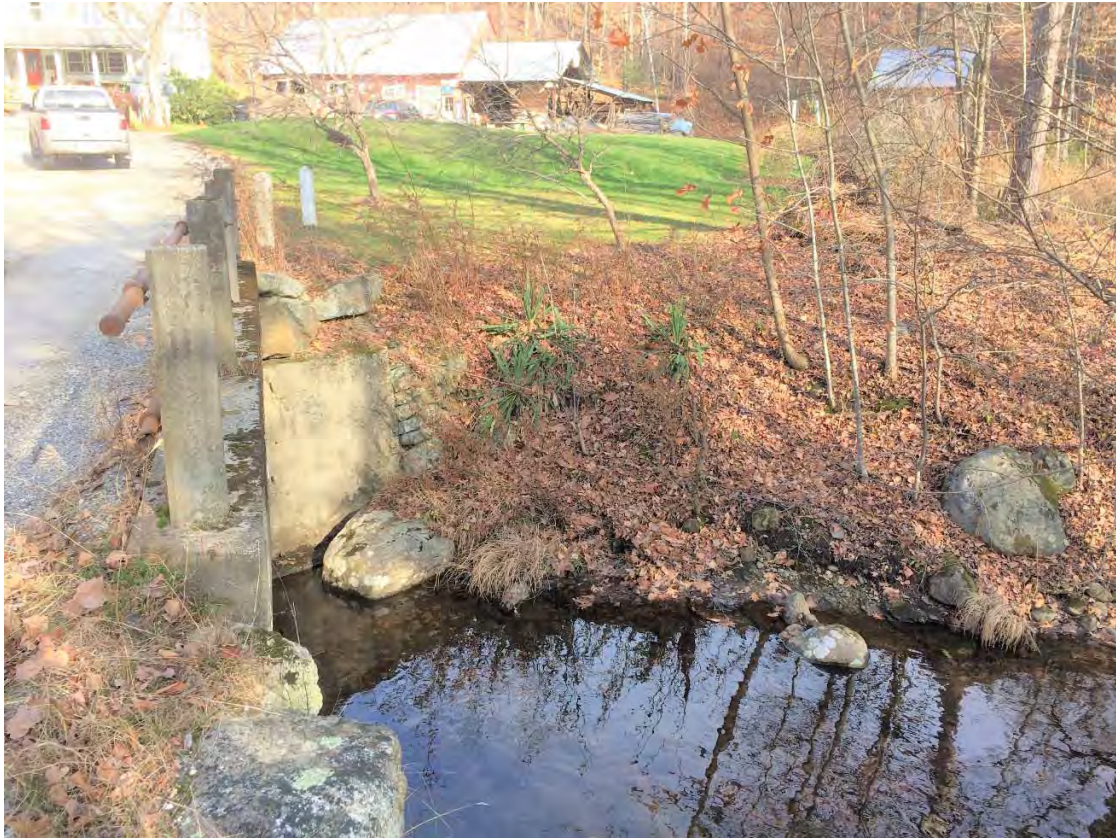
Northeast bridge quadrant
