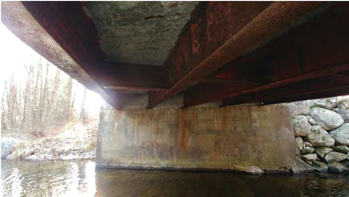
Southerly abutment wall
