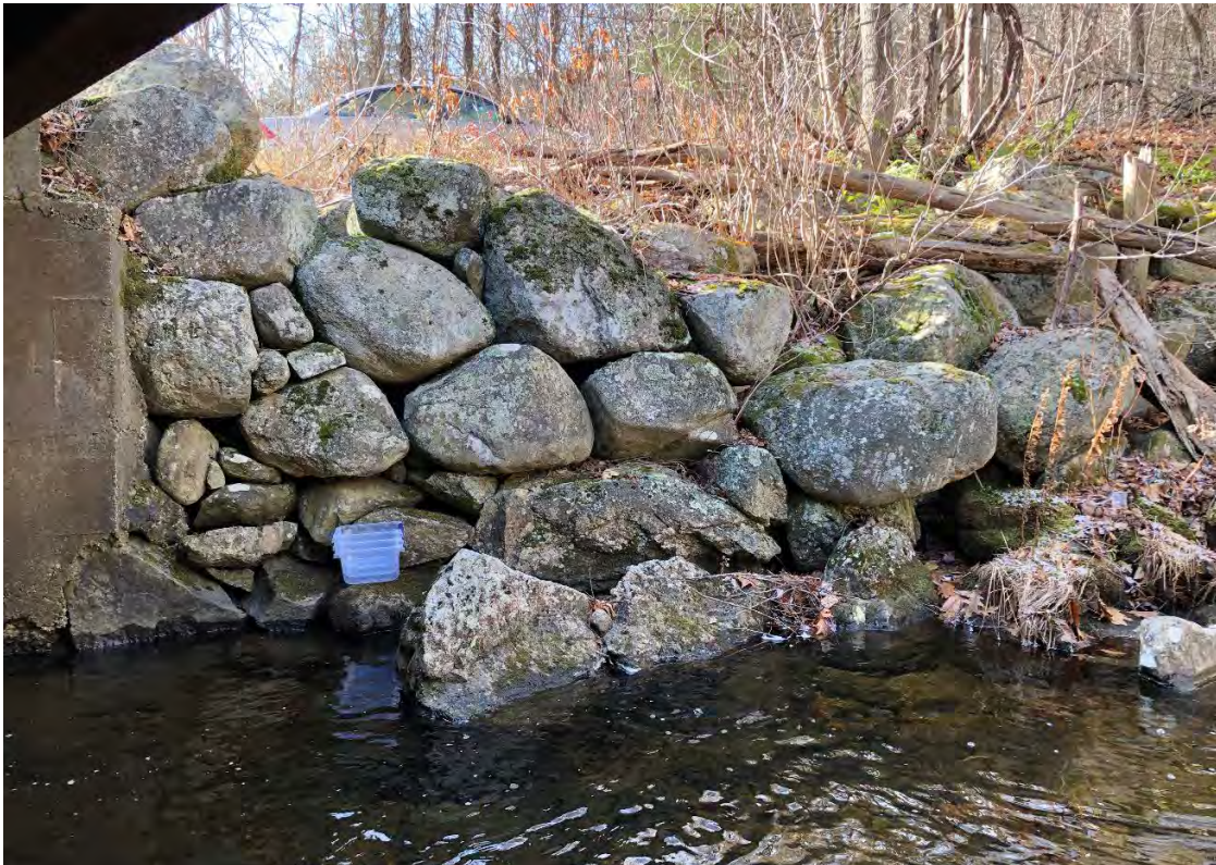
Southwest bridge quadrant
