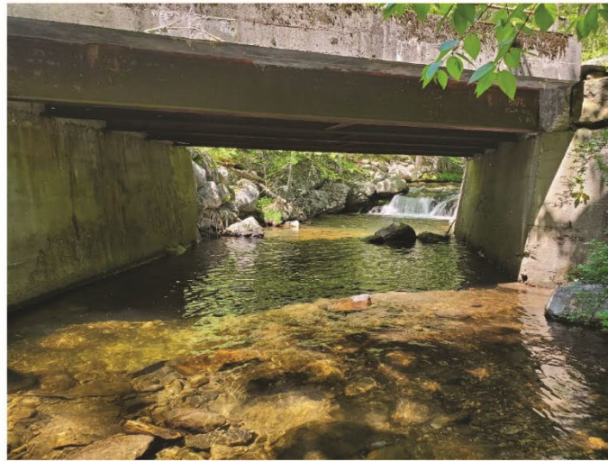
Figure 10: Upstream View Through the Bridge
