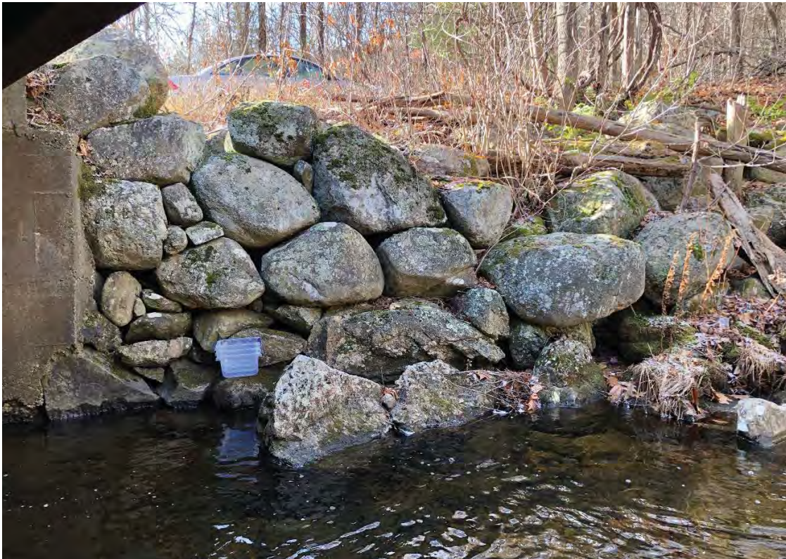
Southwest bridge quadrant
