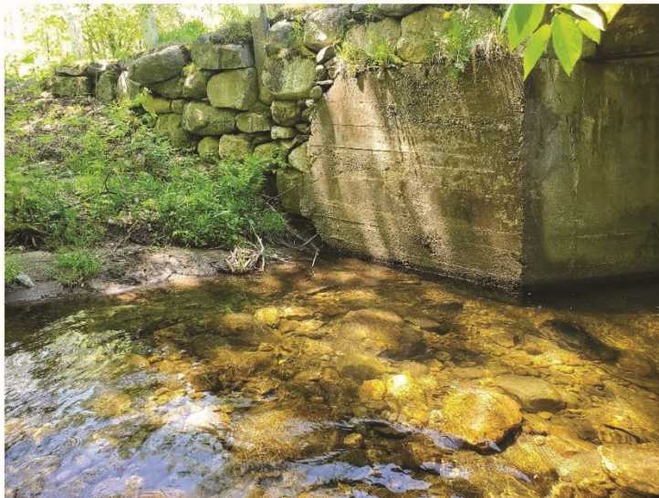
Figure 9: Downstream Right Bridge Abutment
