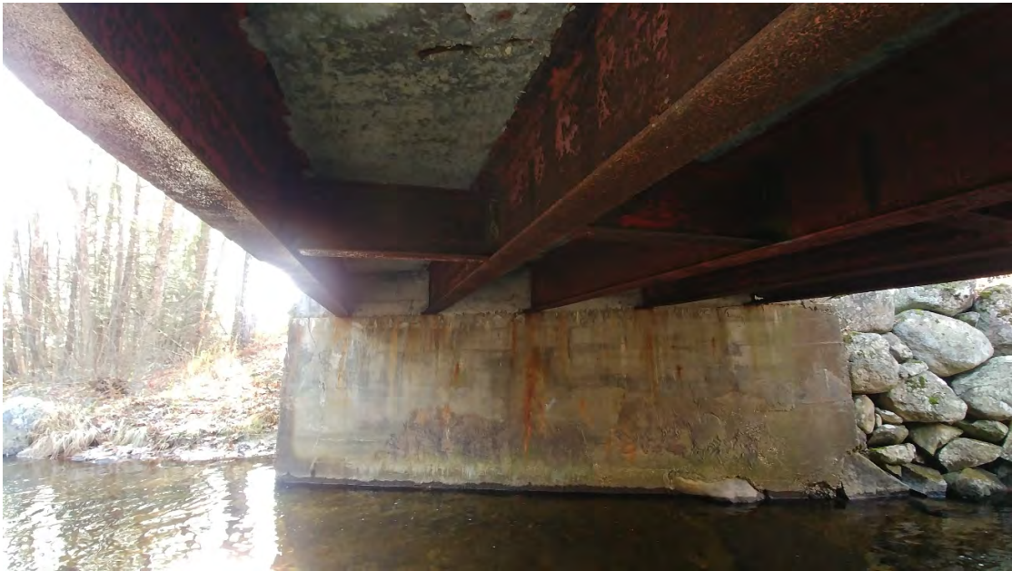
Southerly abutment wall
