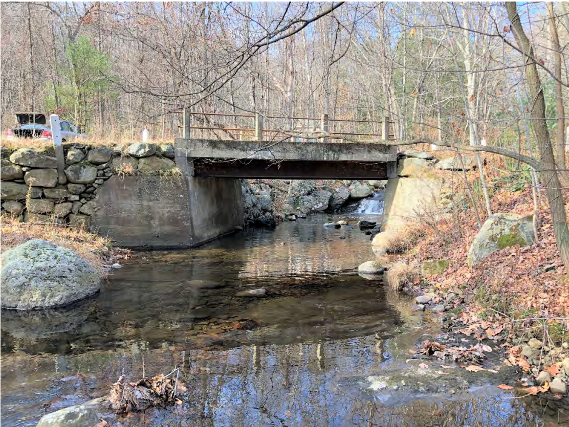
Looking upstream at bridge (looking west)
