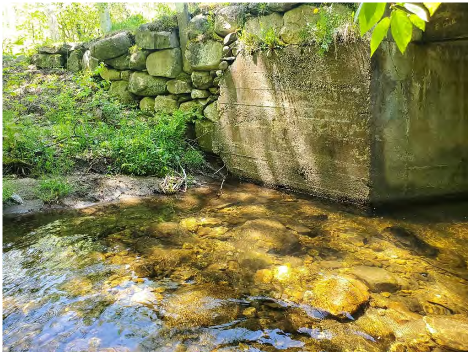
Figure 9: Downstream Right Bridge Abutment
