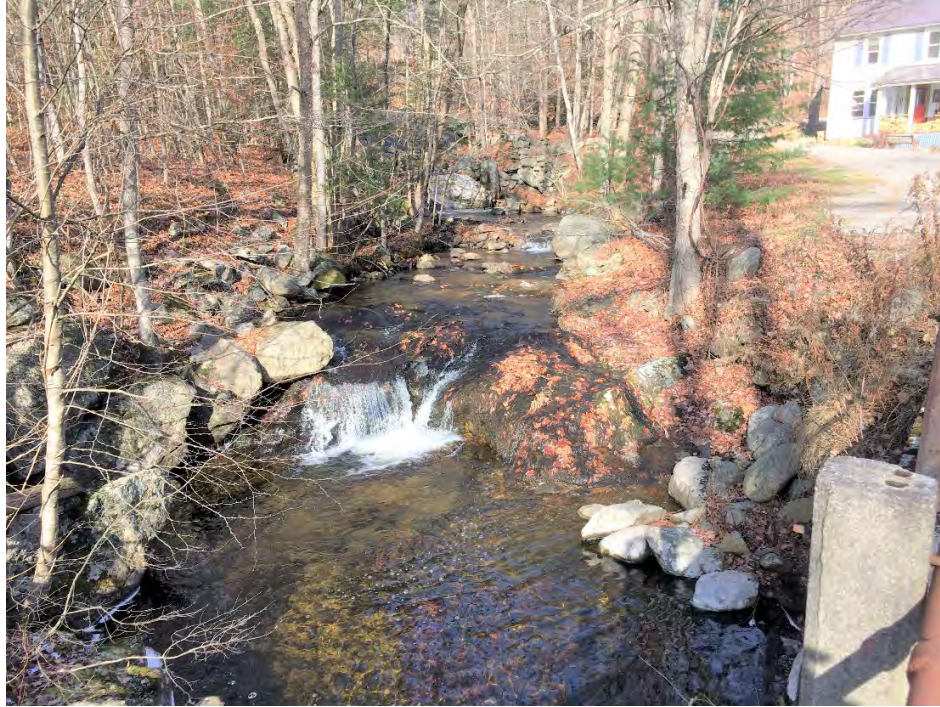
Looking upstream from bridge
