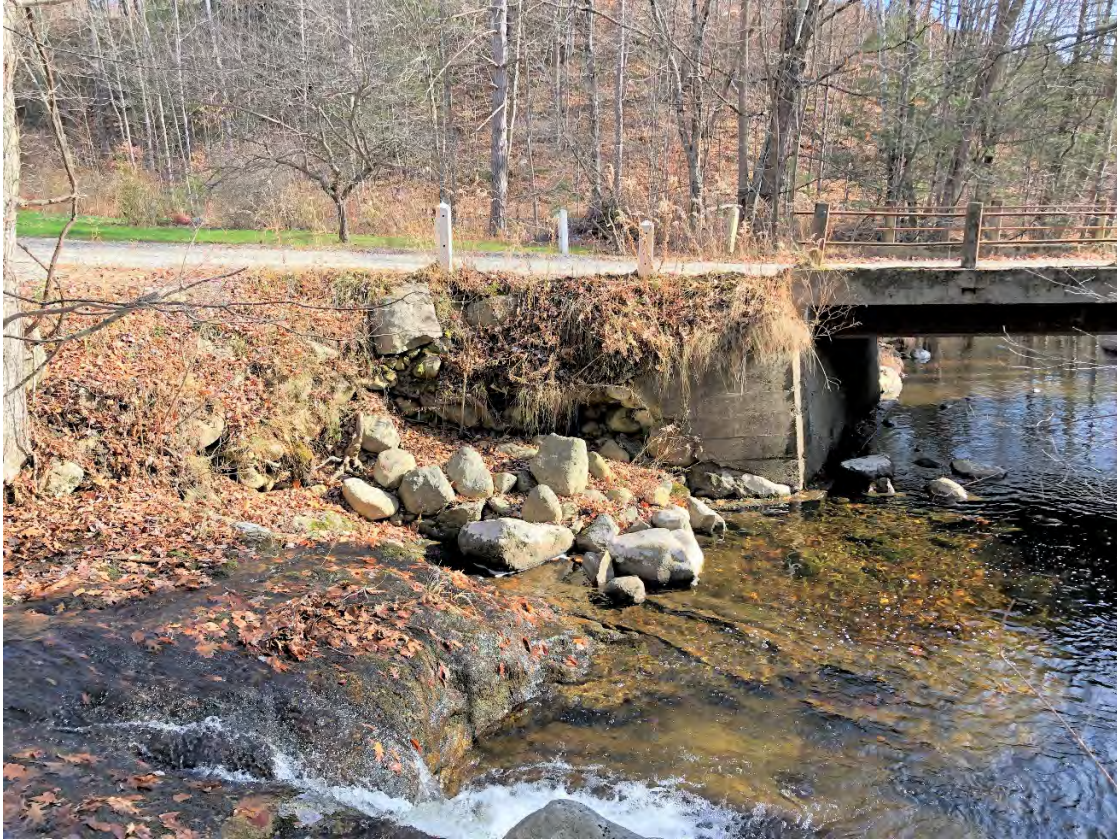
Northwest bridge quadrant
