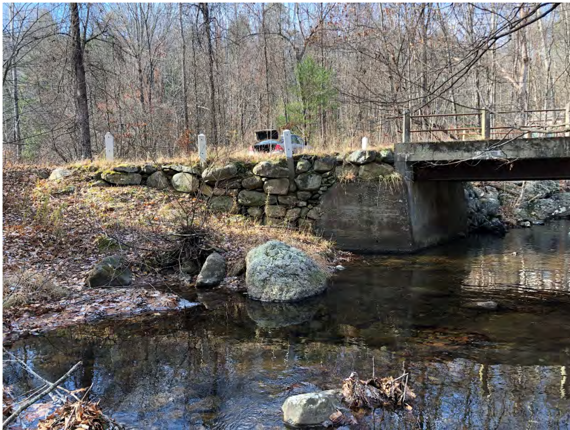
Southeast bridge quadrant
