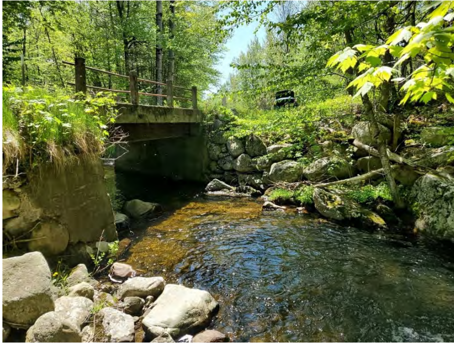
Figure 8: Upstream Face of the Existing Bridge
