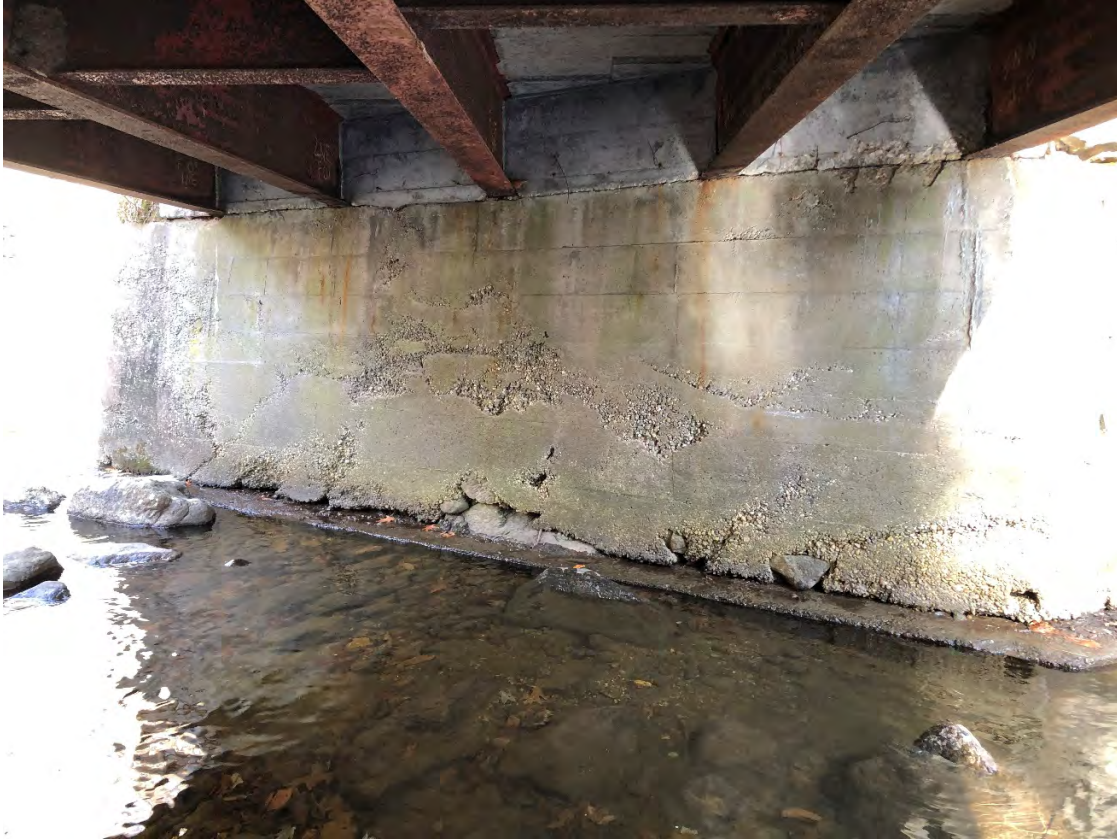
Northerly abutment wall
