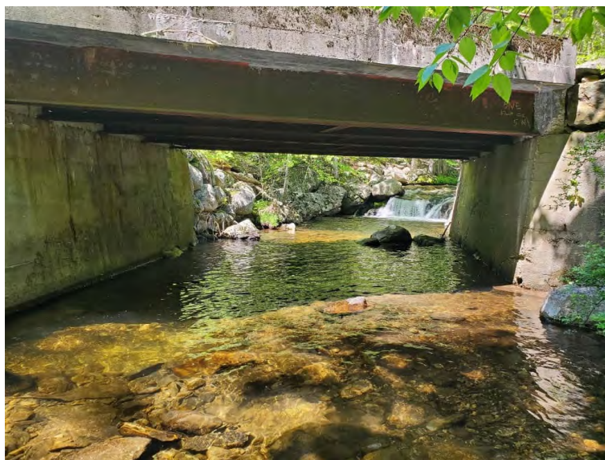
Figure 10: Upstream View Through the Bridge
