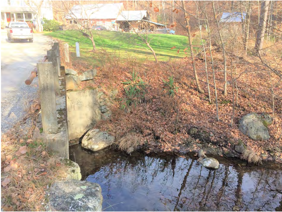
Northeast bridge quadrant
