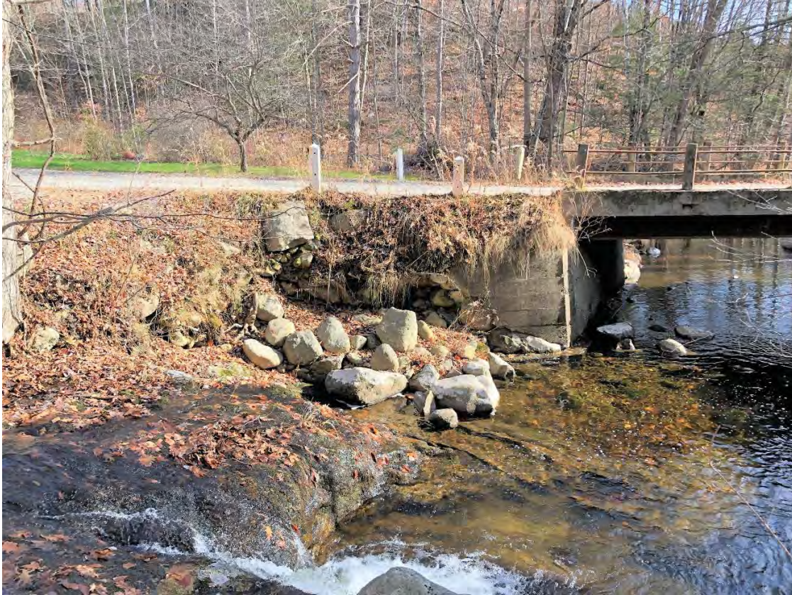
Northwest bridge quadrant
