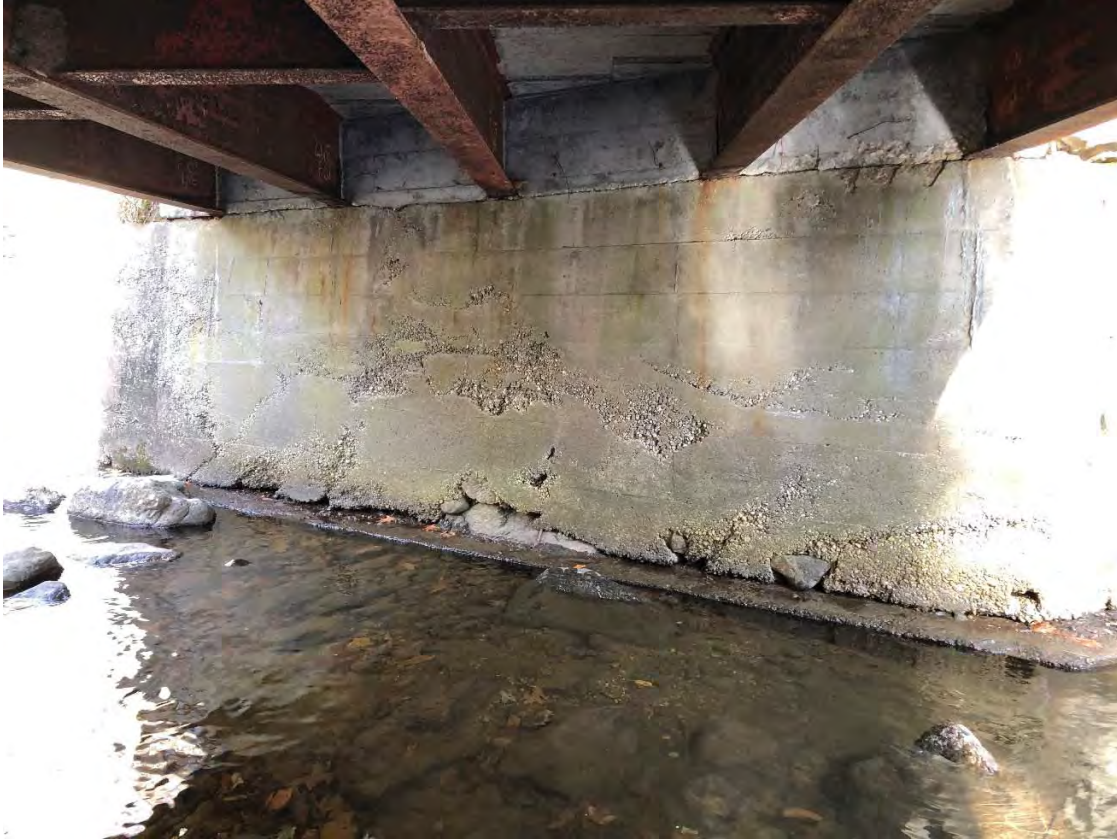
Northerly abutment wall
