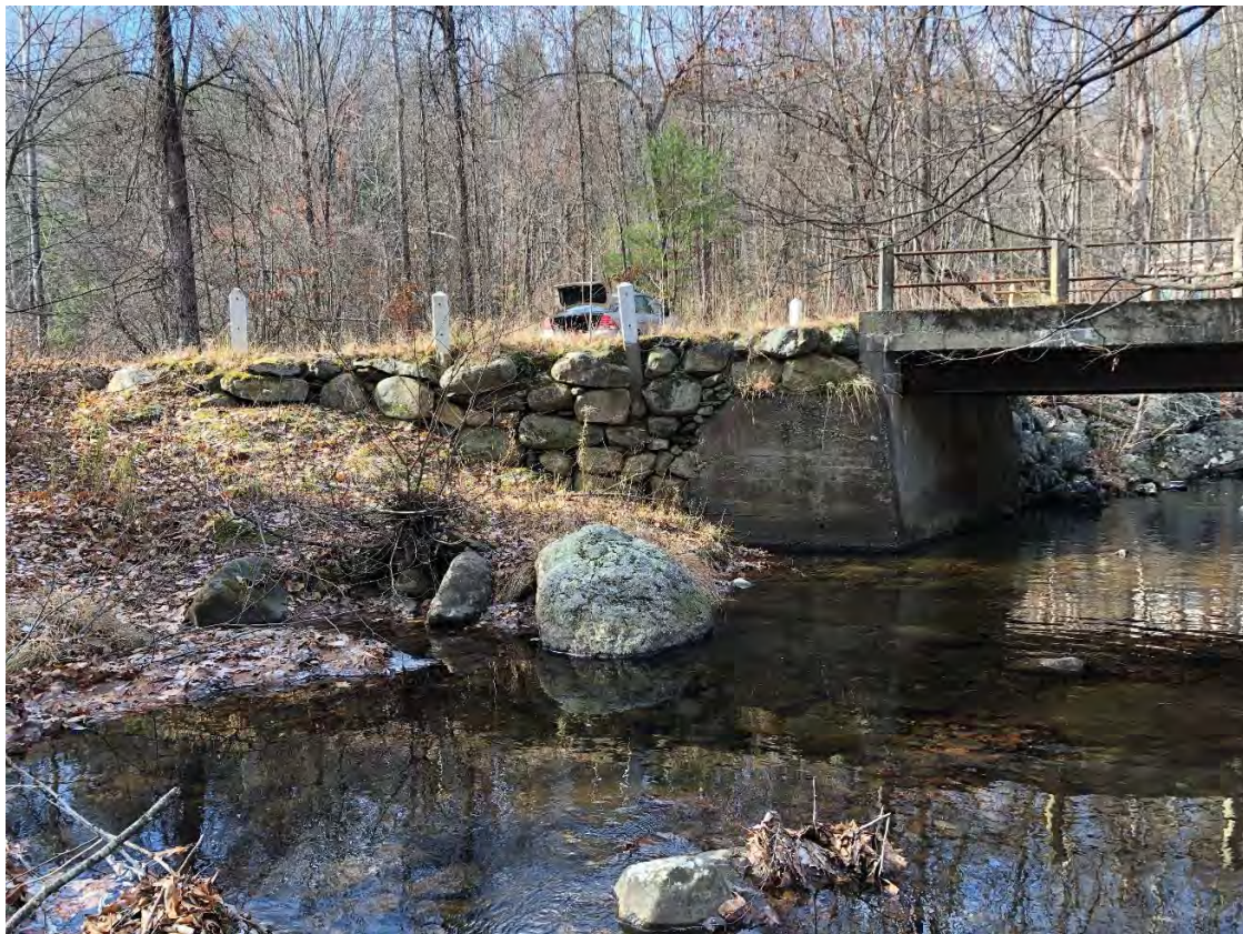
Southeast bridge quadrant
