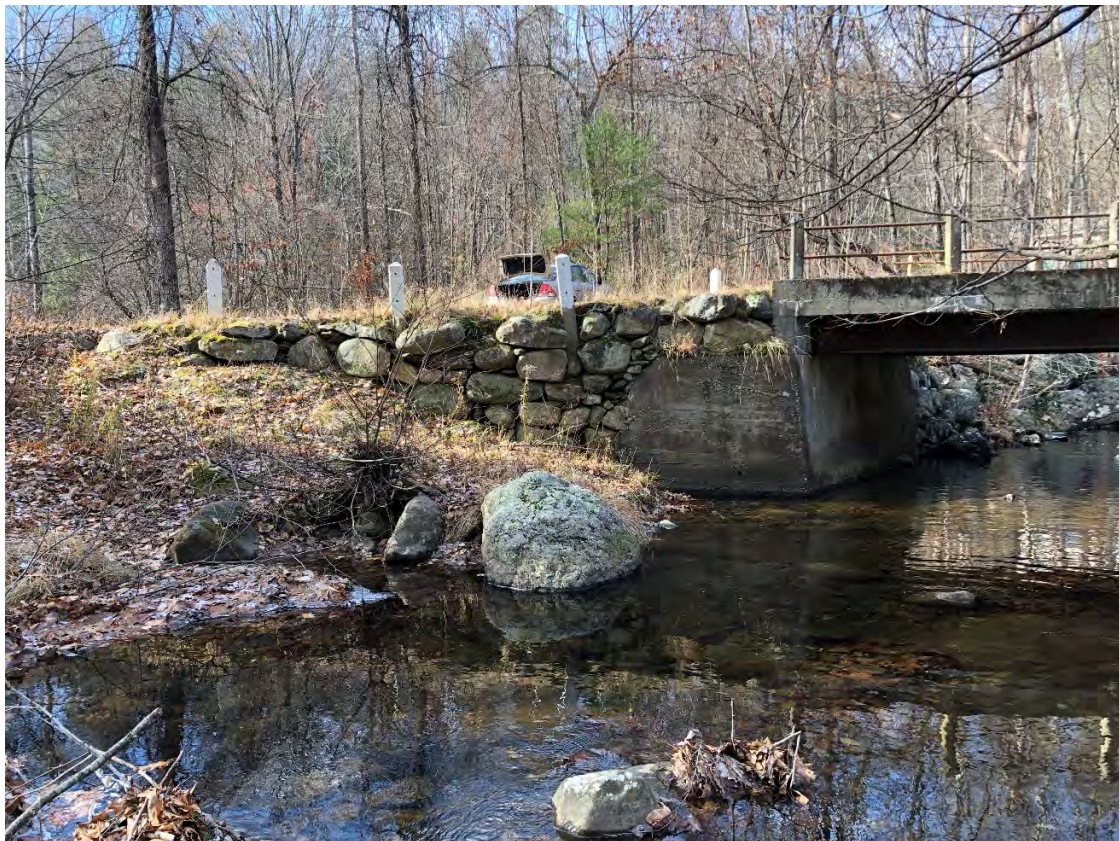
Southeast bridge quadrant
