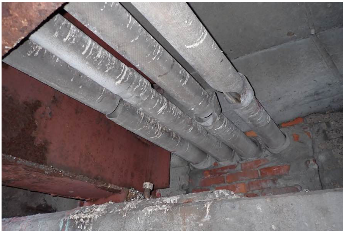
Photo 21: East end of bay 1 in span 2.
