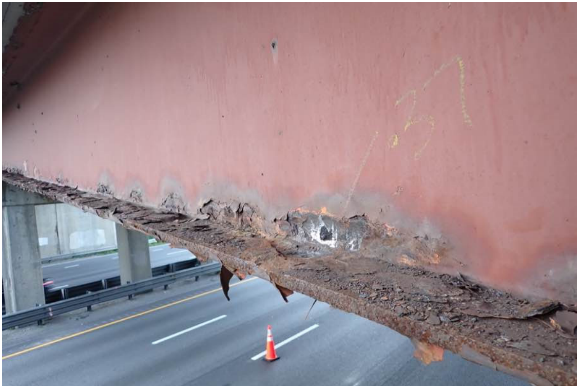
Photo 26: Beam S1 looking east.
