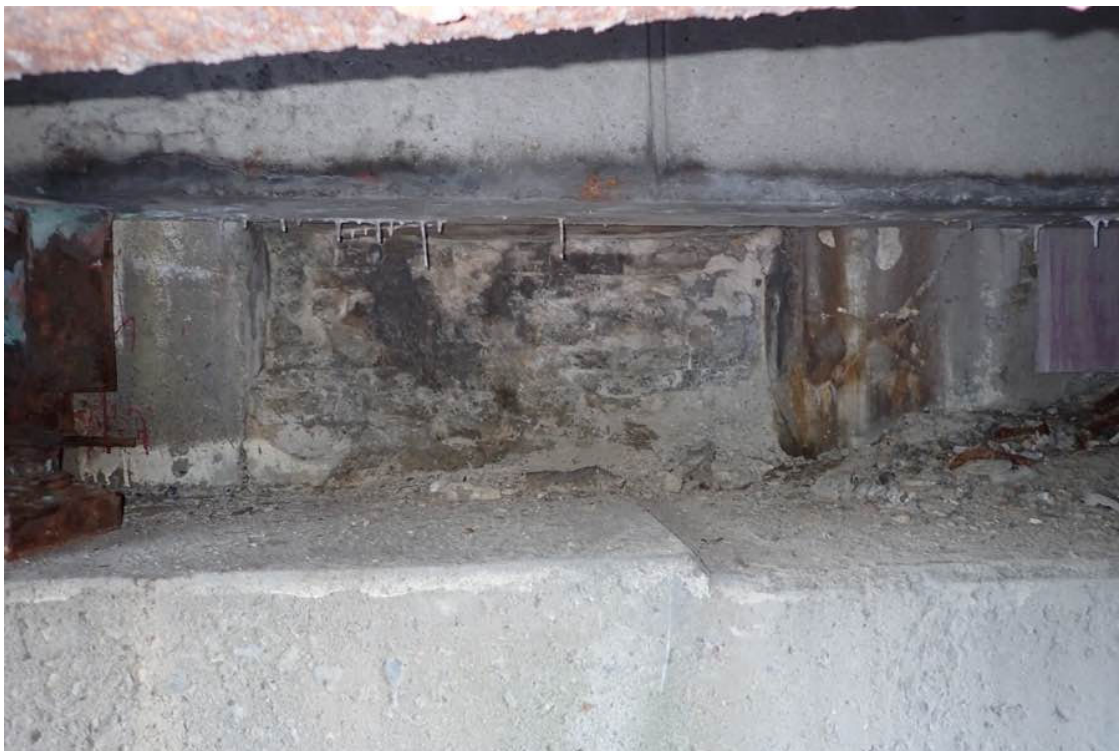
Photo 52: West backwall, bay #5.
