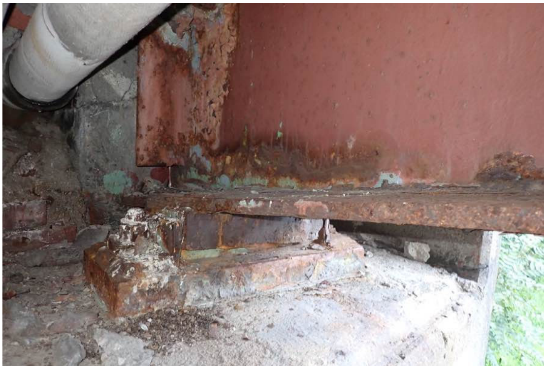
Photo 33: Beam S1 opposite side.
