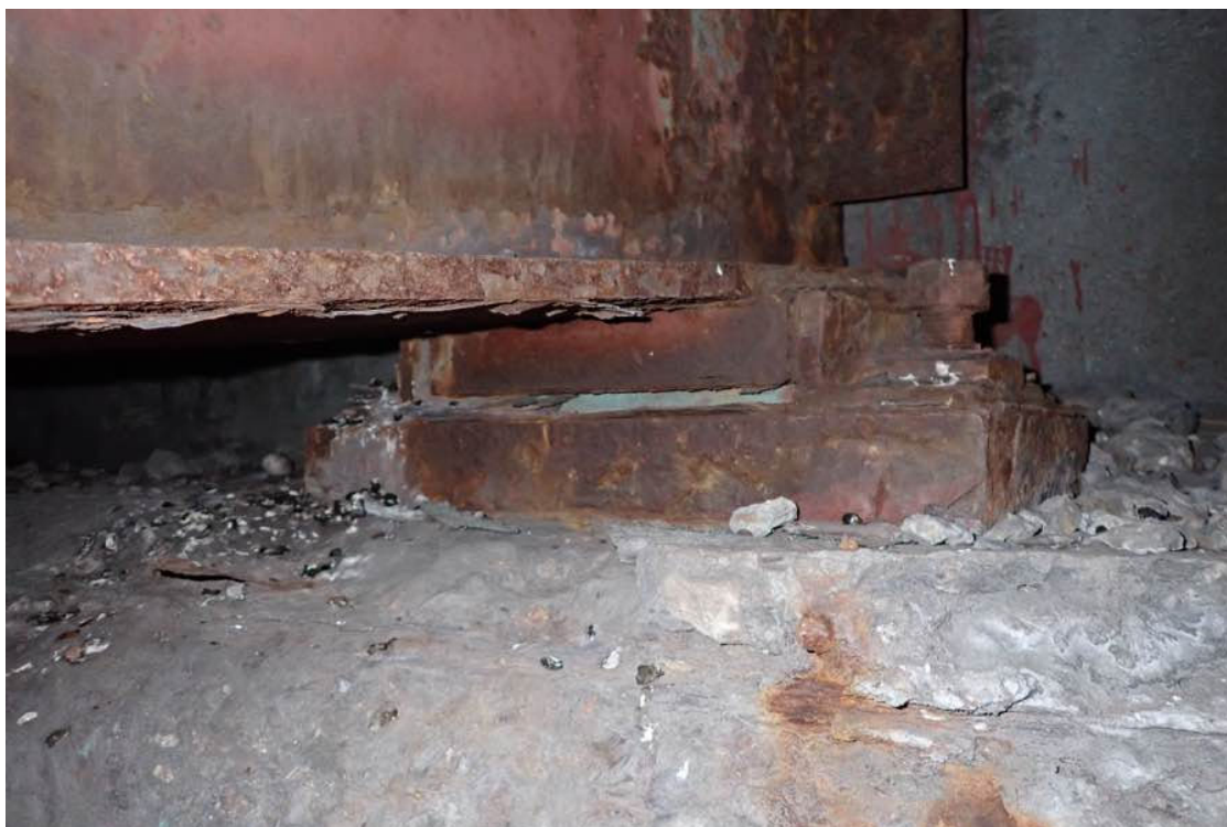
Photo 46: Typical condition of the abutment bearings, bearing to beam S11 shown.
