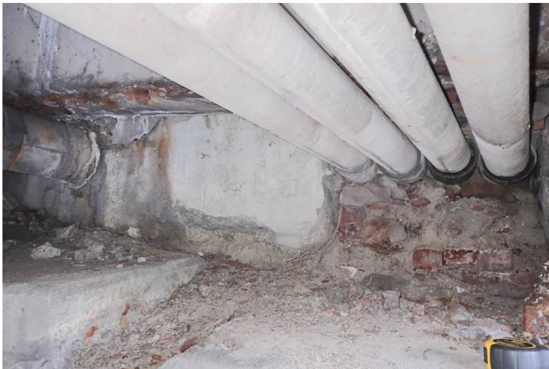
Photo 53: West backwall, bay #1.
