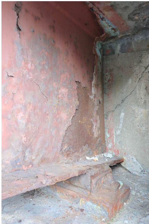
Photo 32: Beam S1 at the west abutment.
