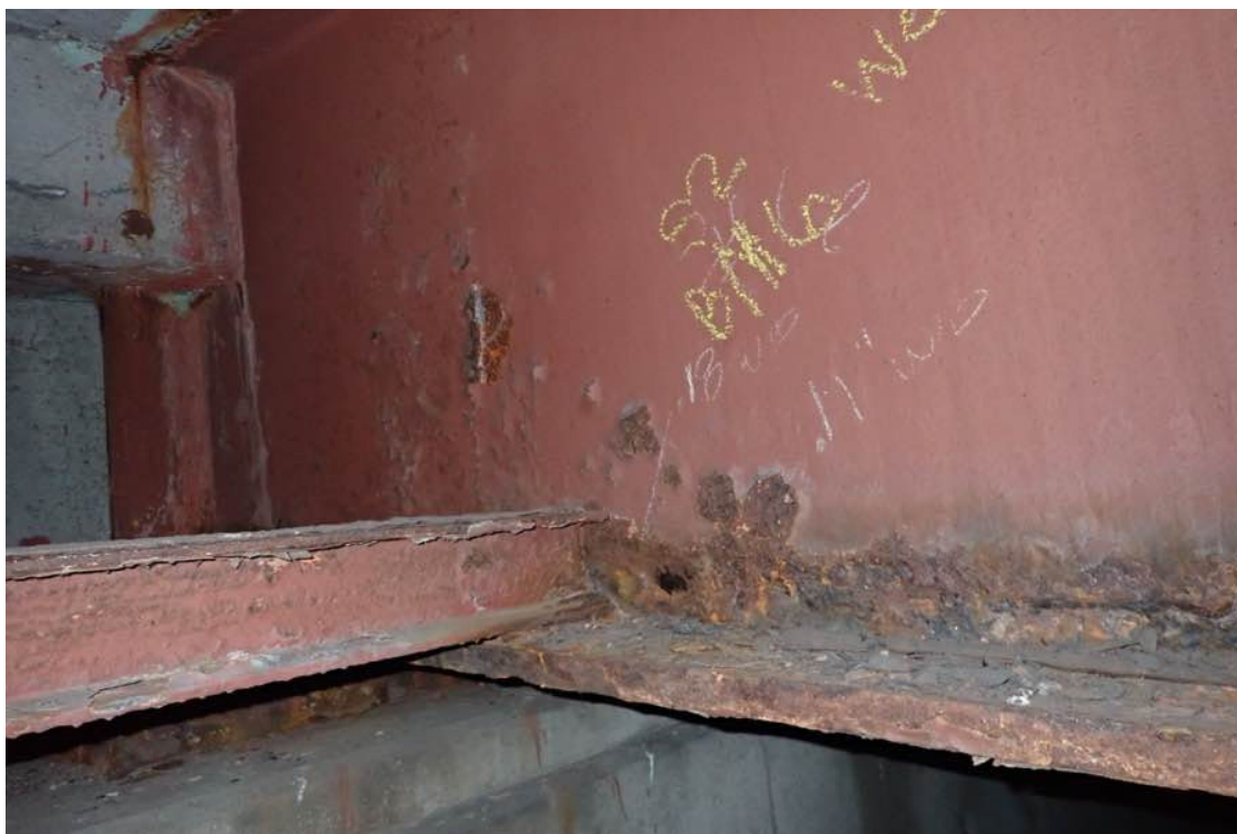
Photo 40: Beam 9 at the east abutment.
