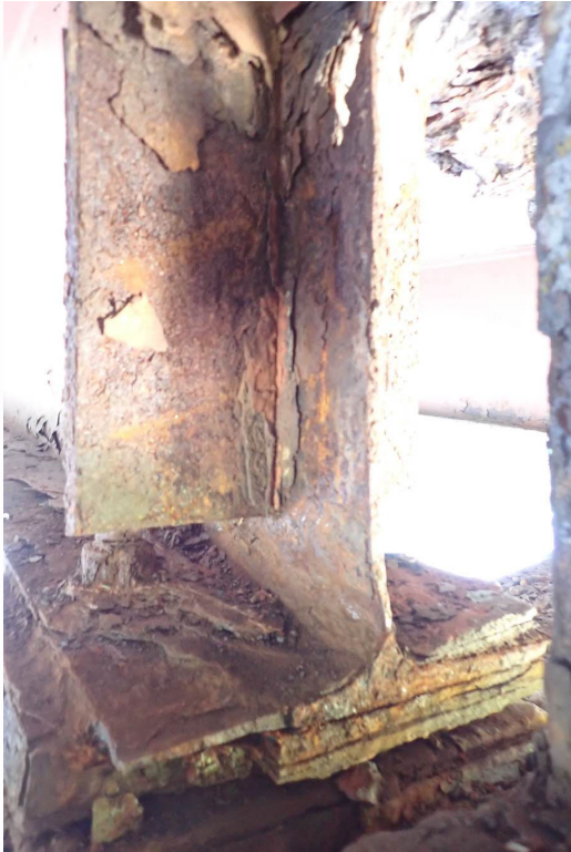
Photo 41: Beam S10 at the pier.
