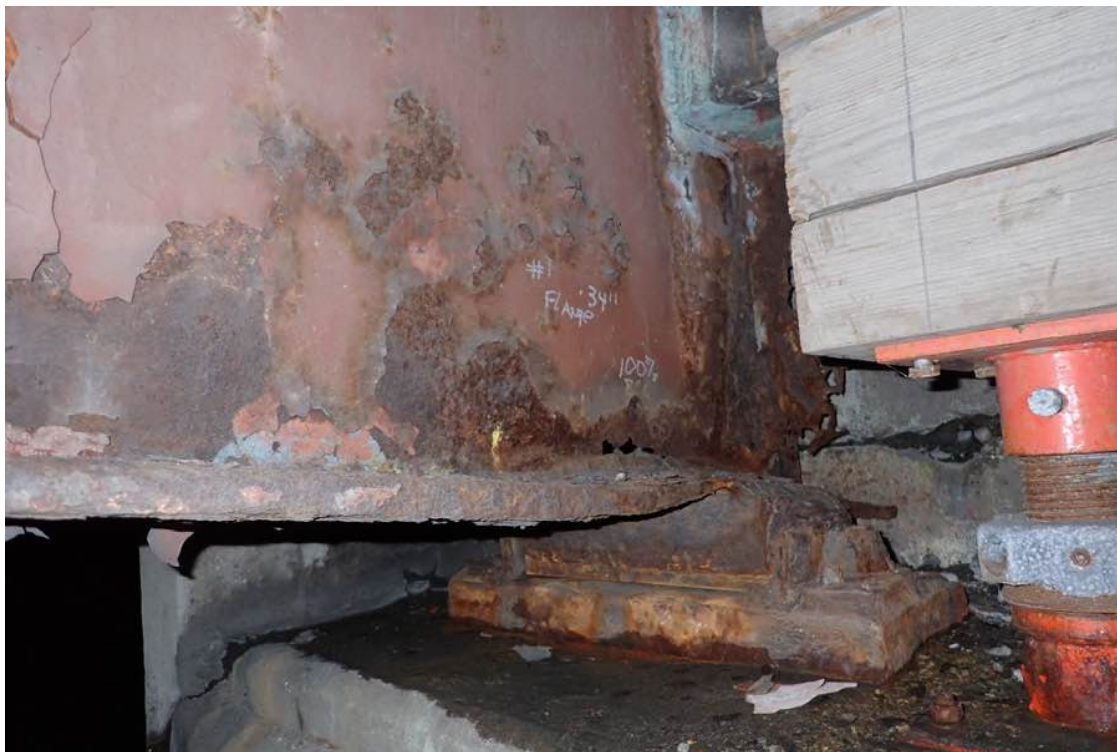
Photo 37: Beam 7 at the west abutment.
