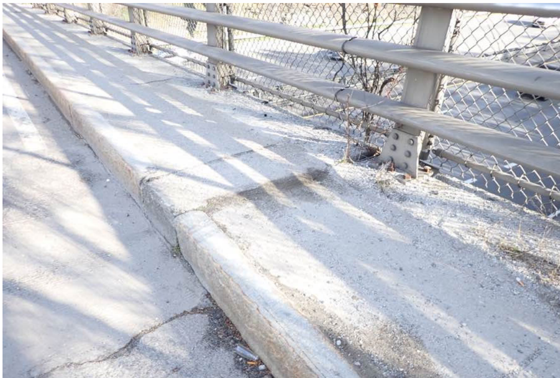
Photo 19: Northeast approach sidewalk.
