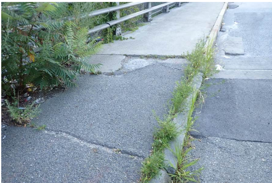
Photo 24: Northwest approach sidewalk.
