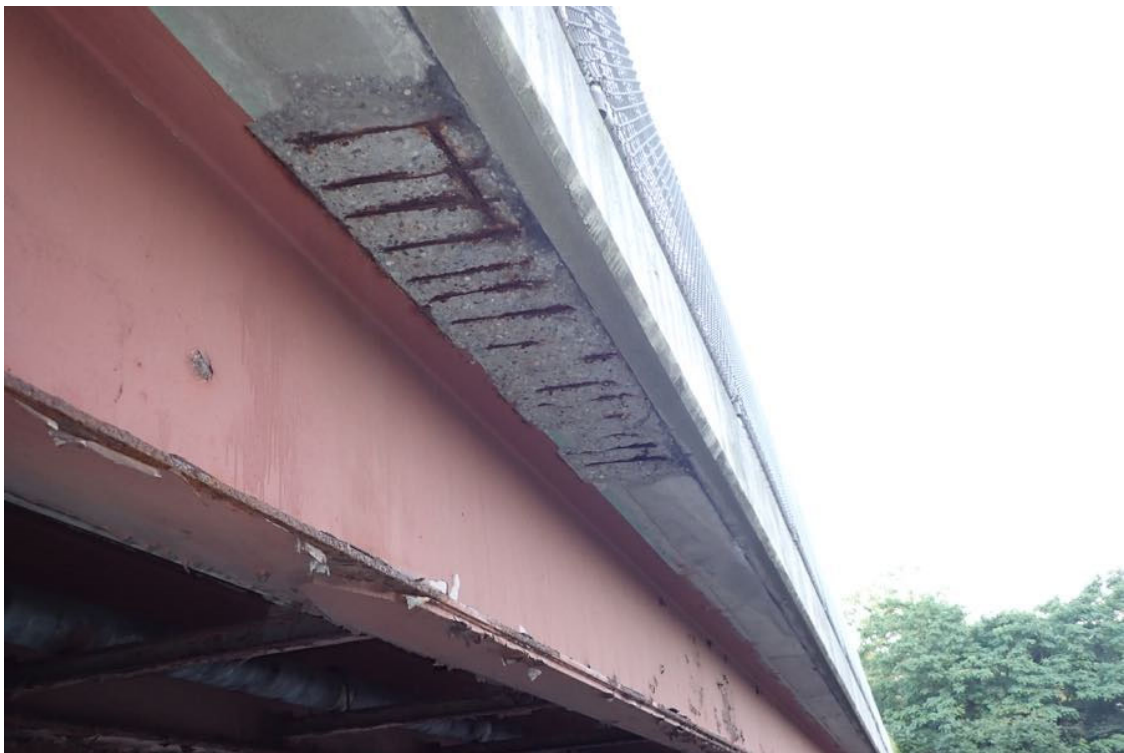
Photo 16: North deck fascia looking west from the ramp lane.
