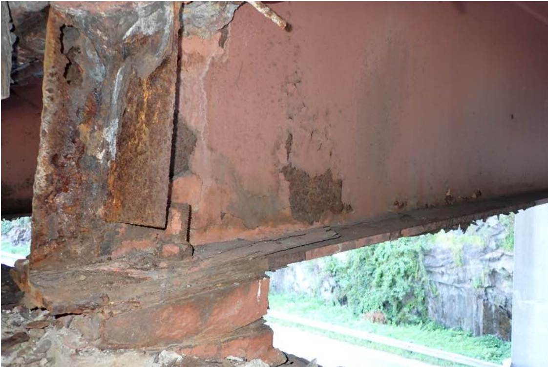
Photo 42: Beam S9 at the pier.
