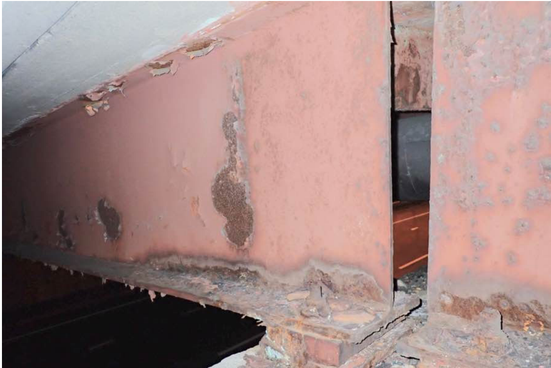
Photo 25: Beam 7 in span 1 at the pier.
