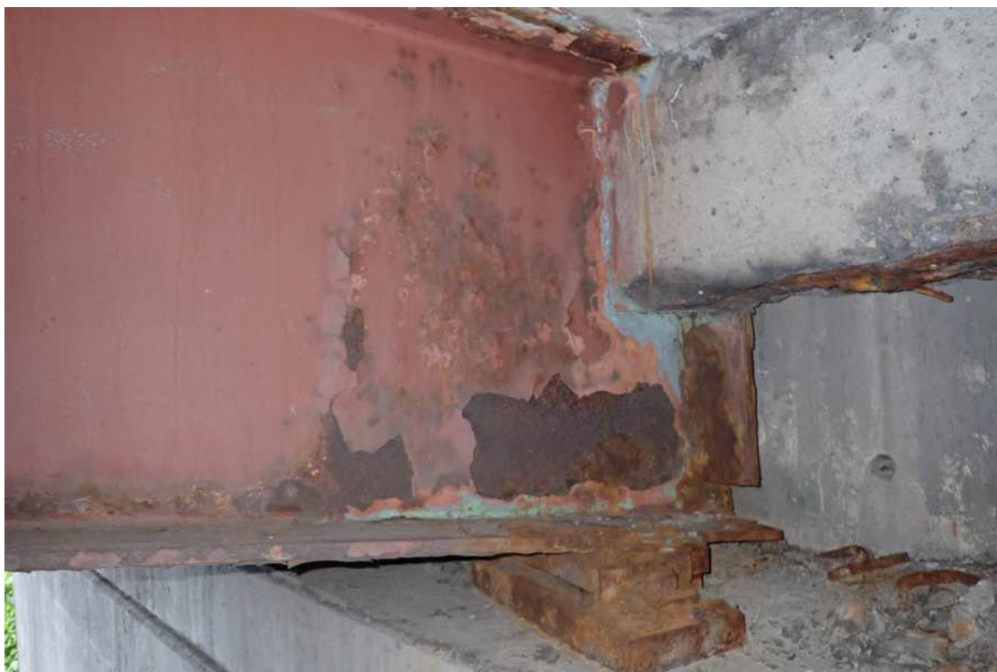
Photo 30: Beam S4 at the west abutment.
