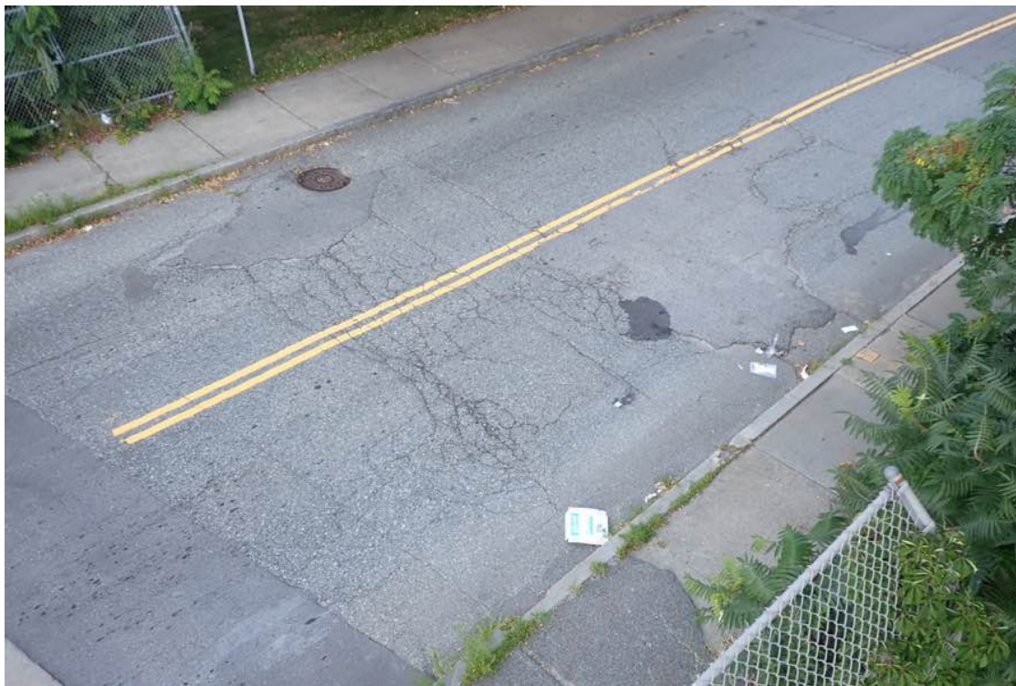
Photo 23: West approach pavement.
