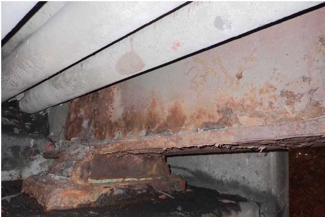
Photo 26: Beam 1 span 1 at the west end.
