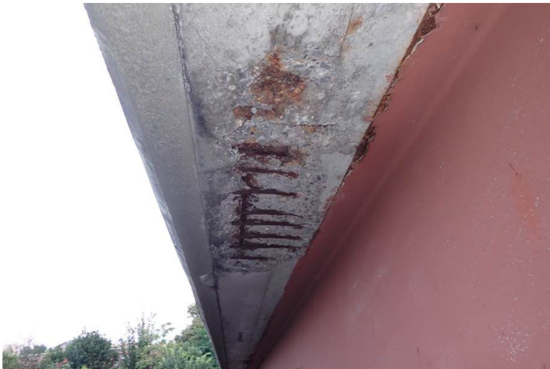
Photo 14: The south deck fascia looking west from the ramp lane.
