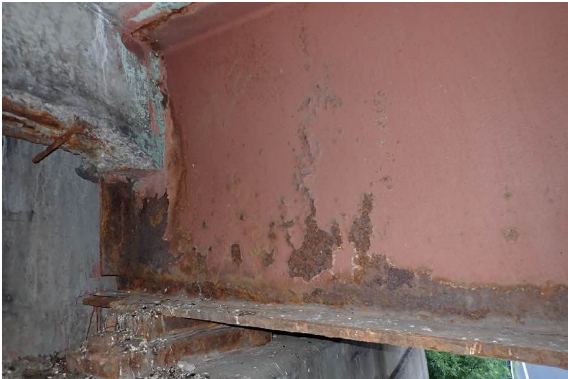
Photo 44: Beam S11 at the east abutment.
