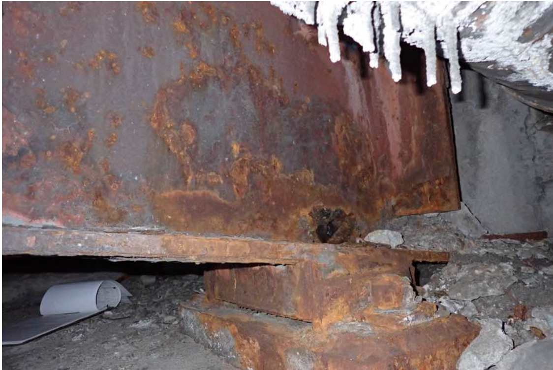
Photo 31: Beam S2 at the west abutment.
