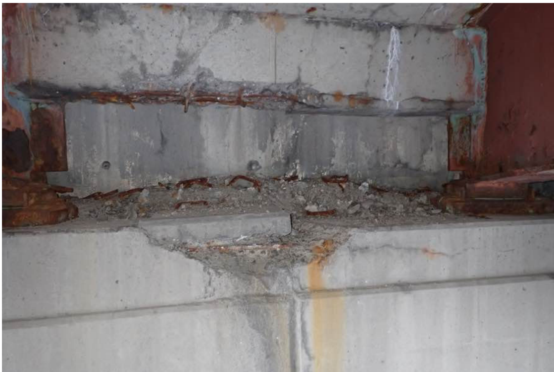
Photo 50: West bridge seat under bay #3.
