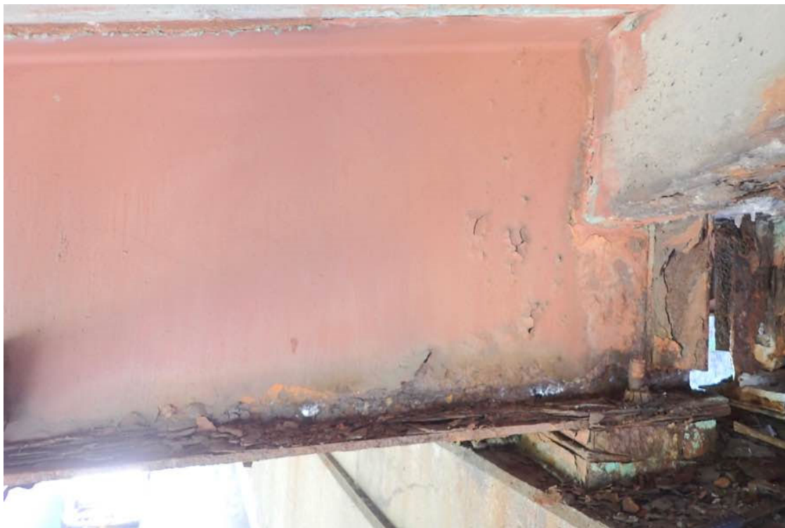
Photo 34: Beam S5 at the pier.
