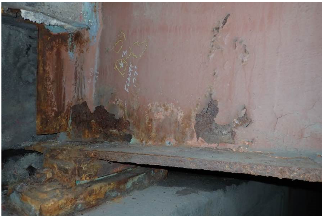
Photo 32: Beam 5 at the west end.
