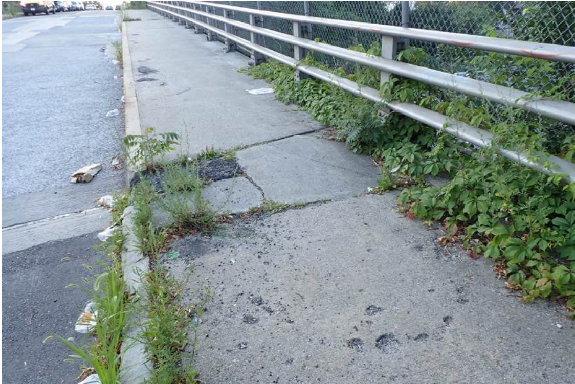
Photo 25: Southwest approach sidewalk.
