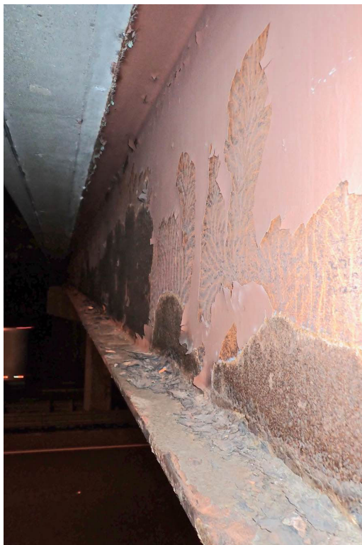
Photo 24: Beam 1 in span 1 looking east.
