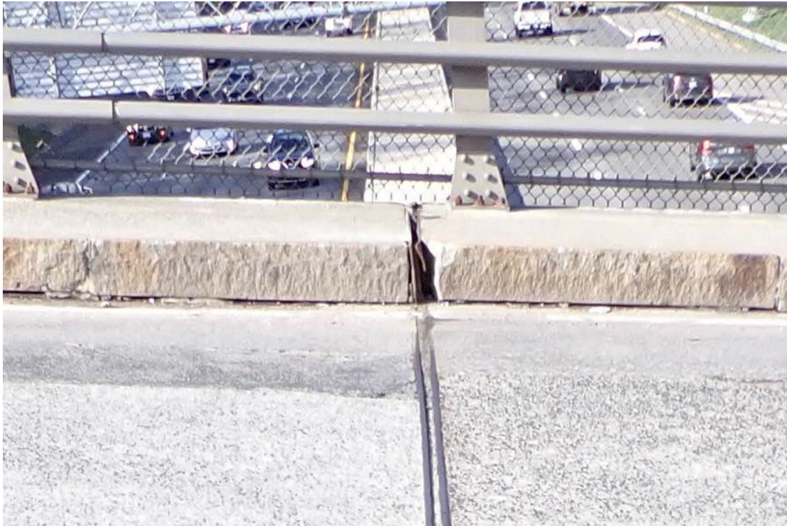
Photo 15: Pier joint collision damage at the south sidewalk.
