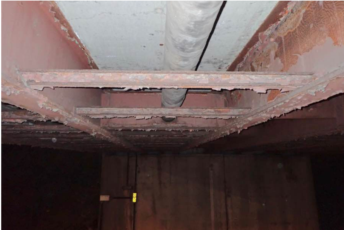
Photo 21: Bay 2 in span 2.
