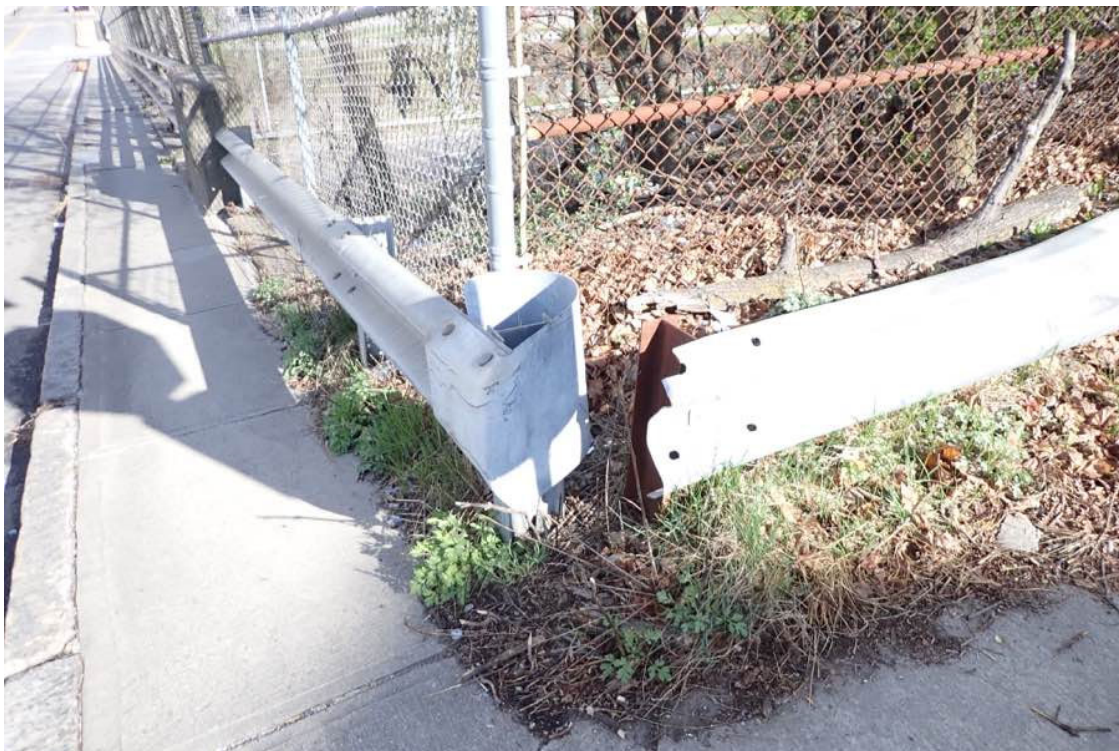
Photo 52: Northeast guardrail end.
