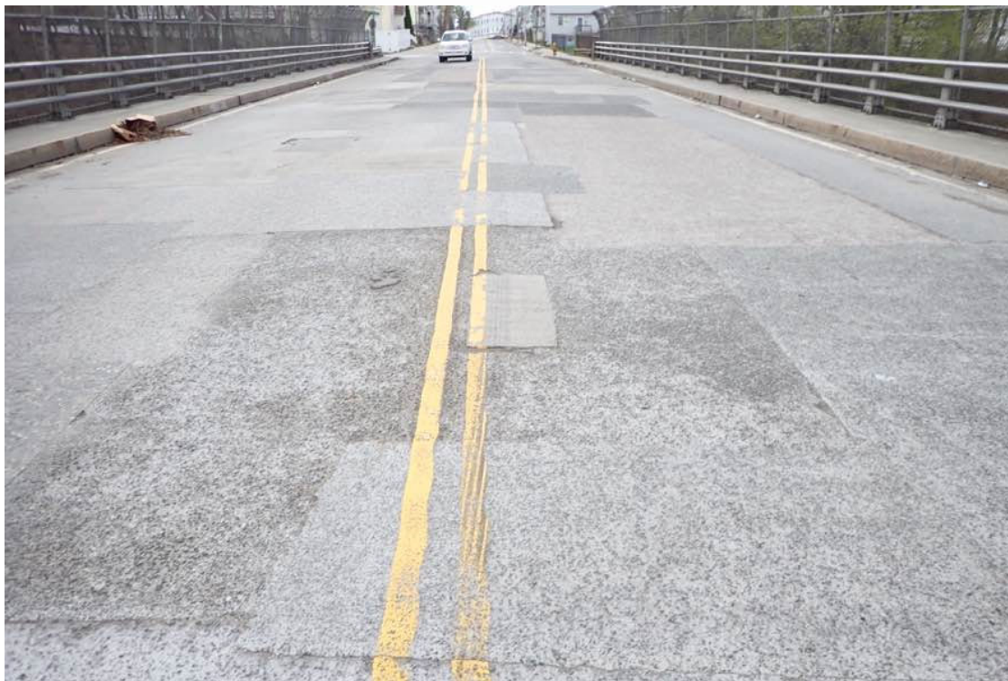
Photo 1: View of the condition of the Duracal patches.
