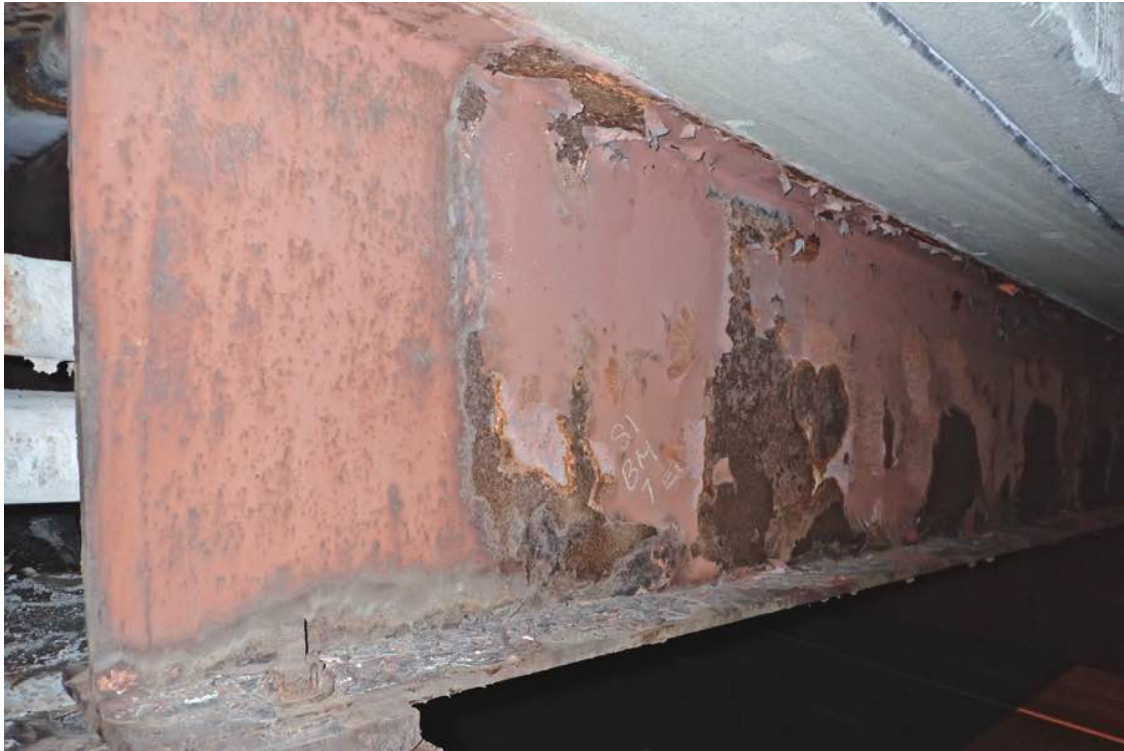
Photo 27: Beam 1 span 1 at the east end.
