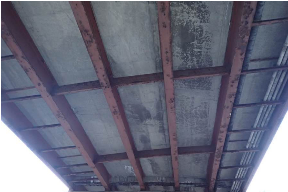
Photo 8: Deck underside span 2.
