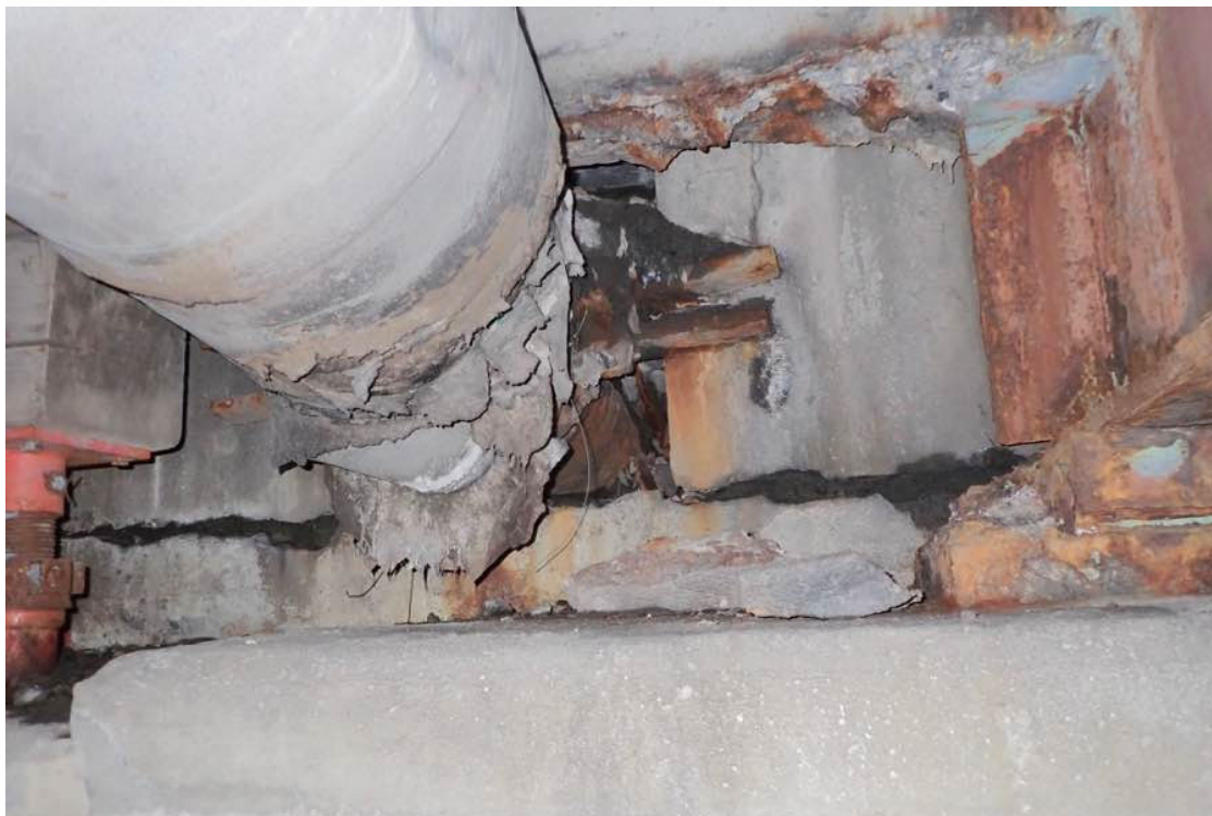
Photo 11: Utility pipe in bay 6, west abutment.
