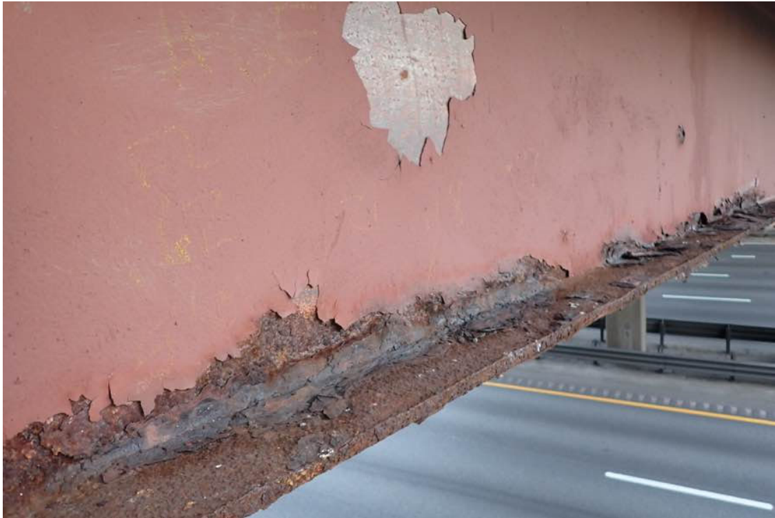
Photo 27: Beam S7 looking west.
