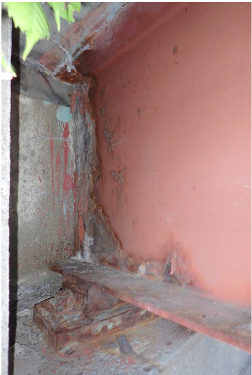
Photo 28: Beam S6 at the west abutment.
