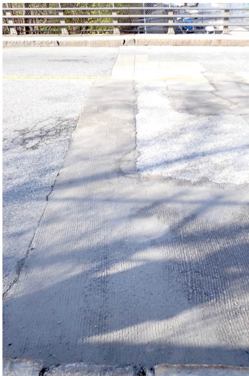
Photo 14: East abutment joint repair.
