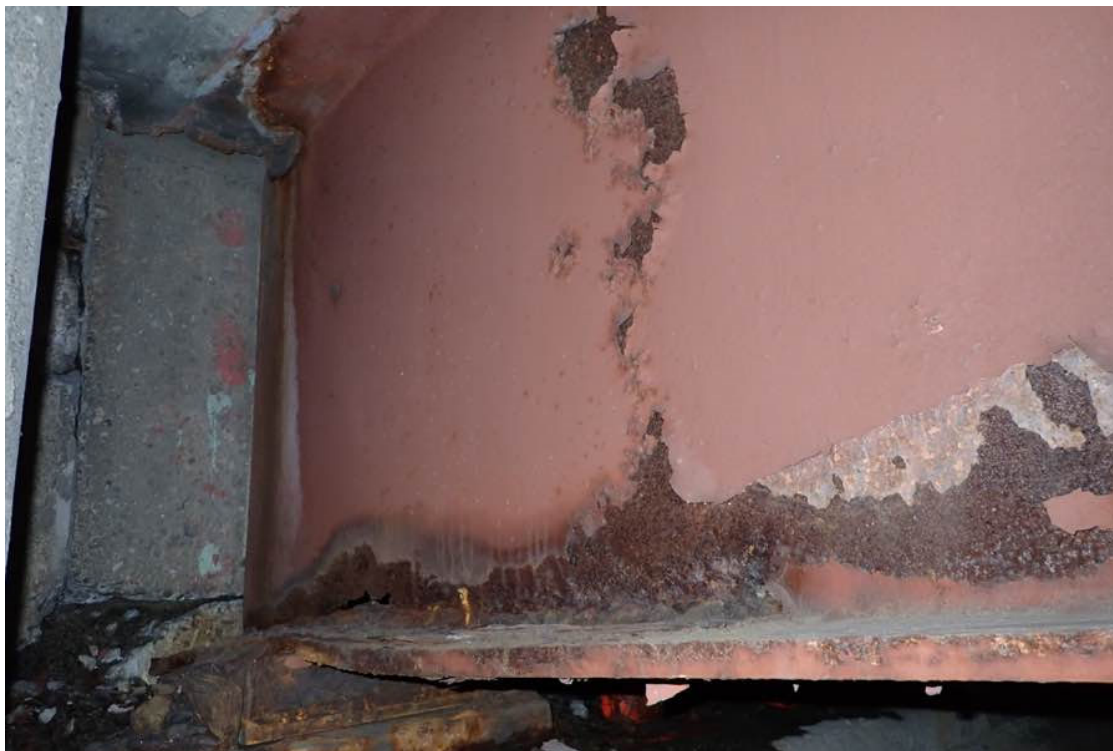
Photo 36: Beam 7 at the west abutment.
