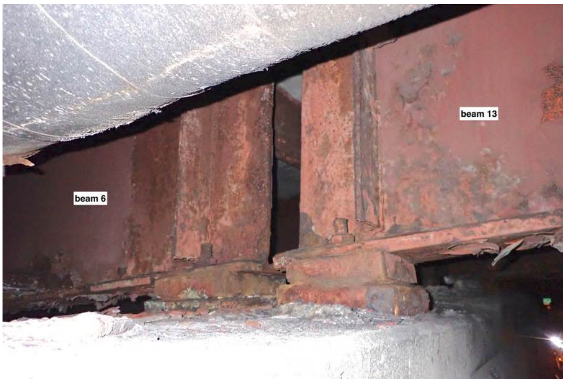
Photo 20: Beams 6 and 13 at the pier.
