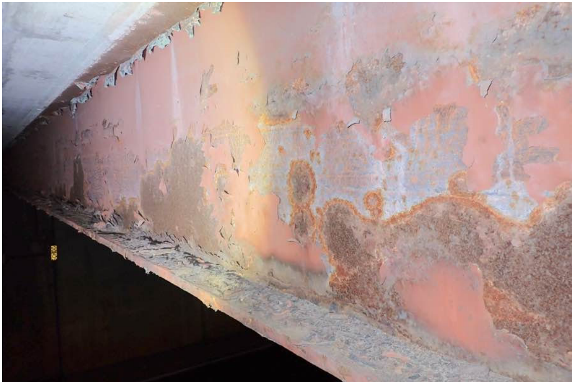
Photo 22: Beam 8 in span 2 looking east.
