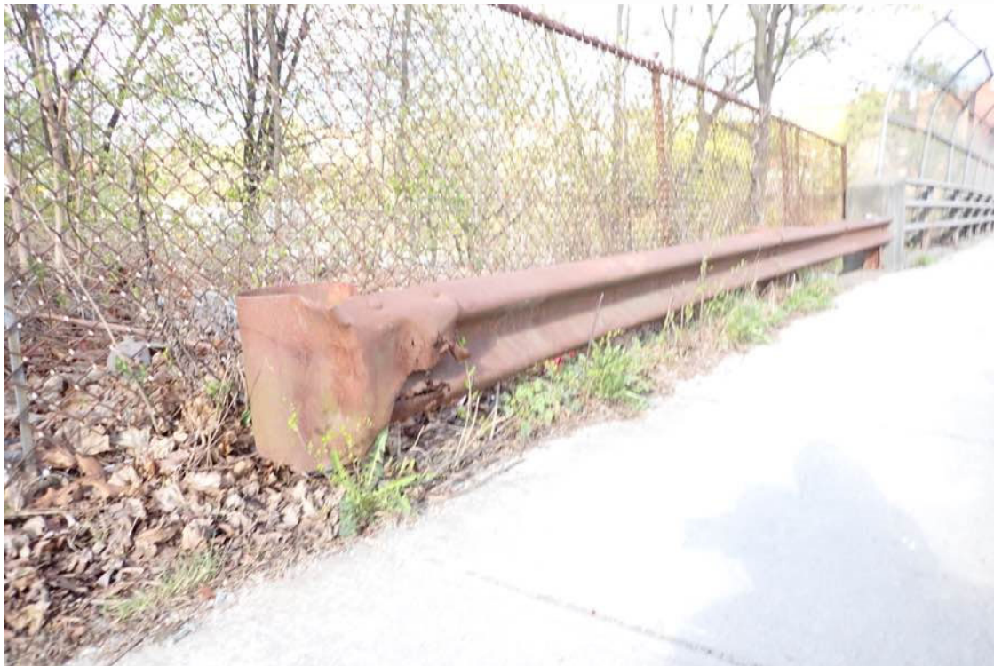
Photo 51: Southeast approach guardrail.
