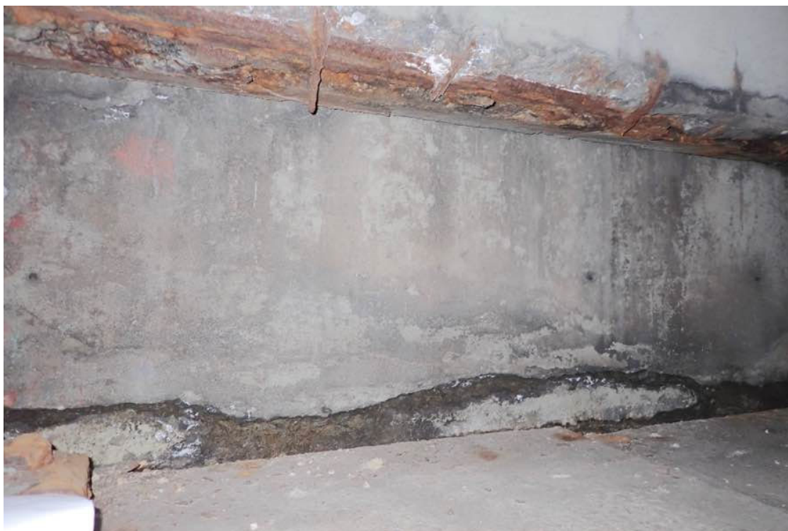
Photo 46: Bay 3, west abutment backwall.
