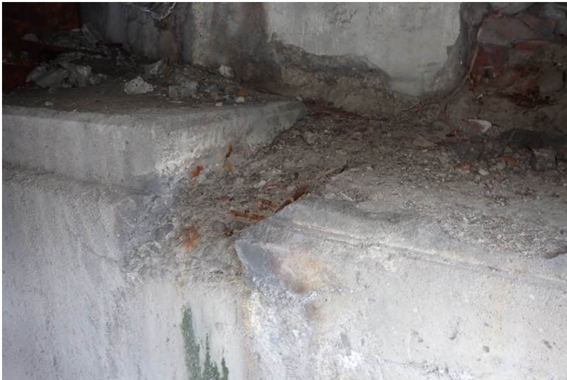
Photo 51: West bridge seat under bay #1.
