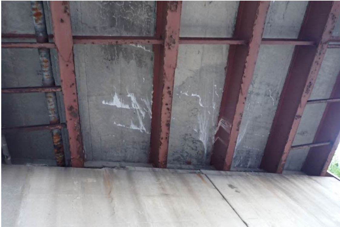
Photo 9: Deck underside span 2 at the east abutment.
