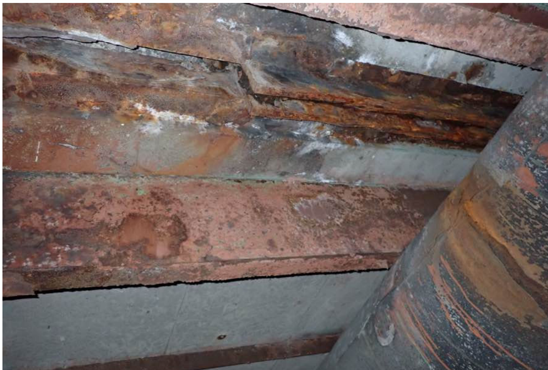
Photo 17: Pier joint in bay 6, sidewalk bay.
