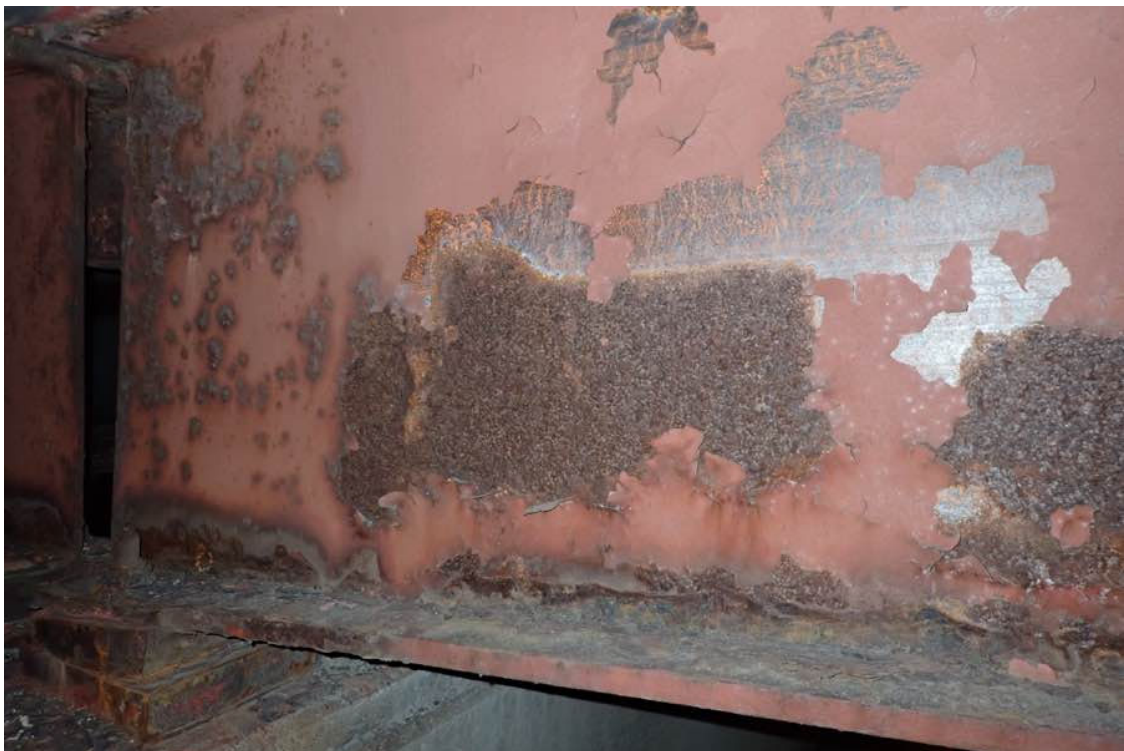
Photo 42: Beam 14 at the pier.
