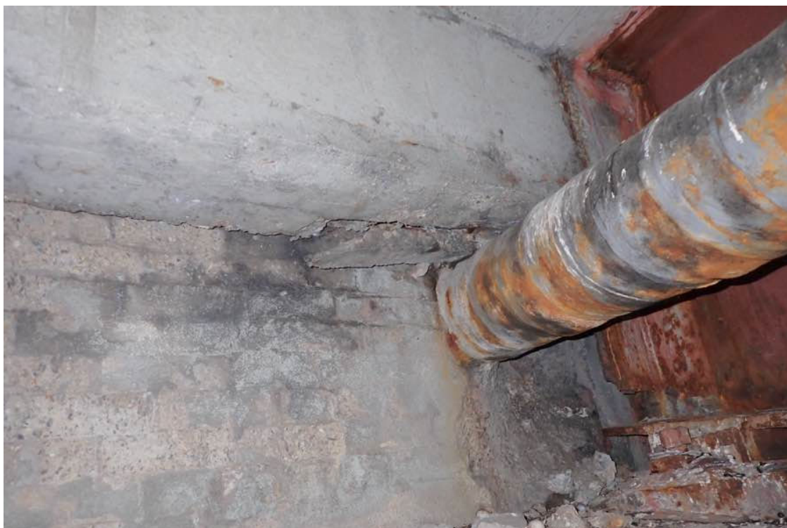
Photo 54: East backwall in bay #1.
