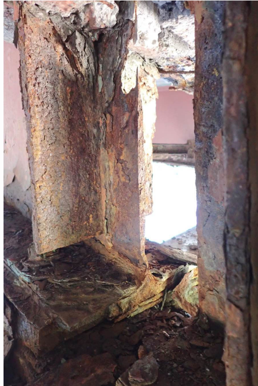
Photo 39: Beam S11 at the pier.
