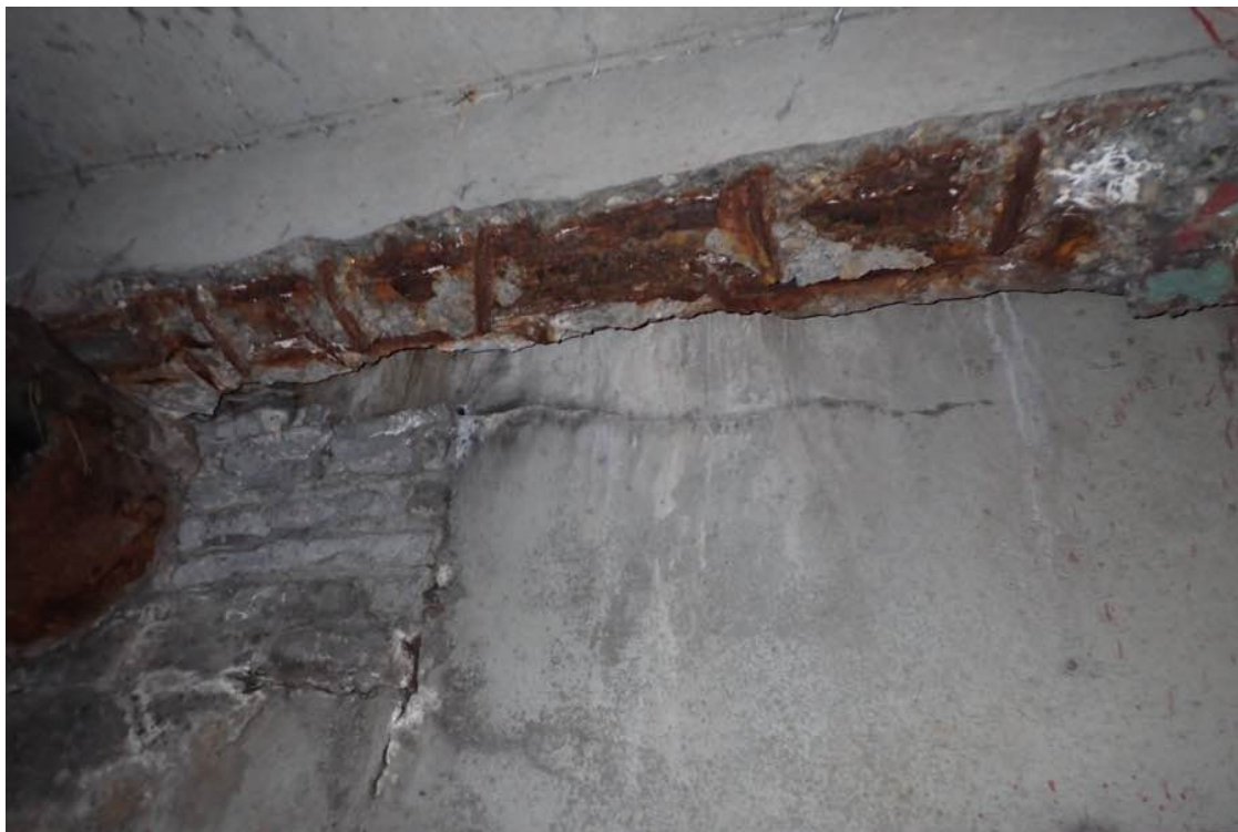
Photo 44: End diaphragm in bay 5, east abutment.
