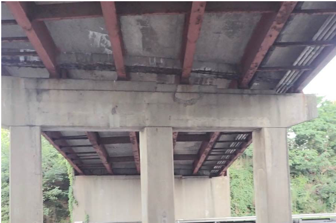
Photo 60: East face of the pier.
