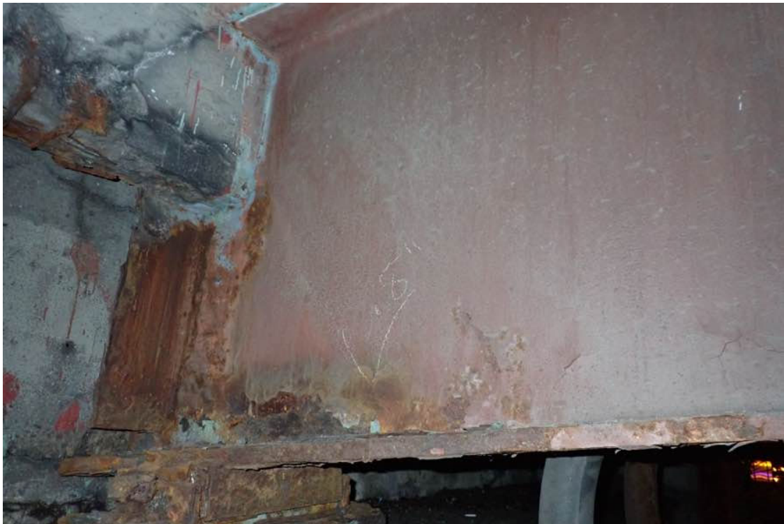
Photo 28: Beam 2 at the west end.
