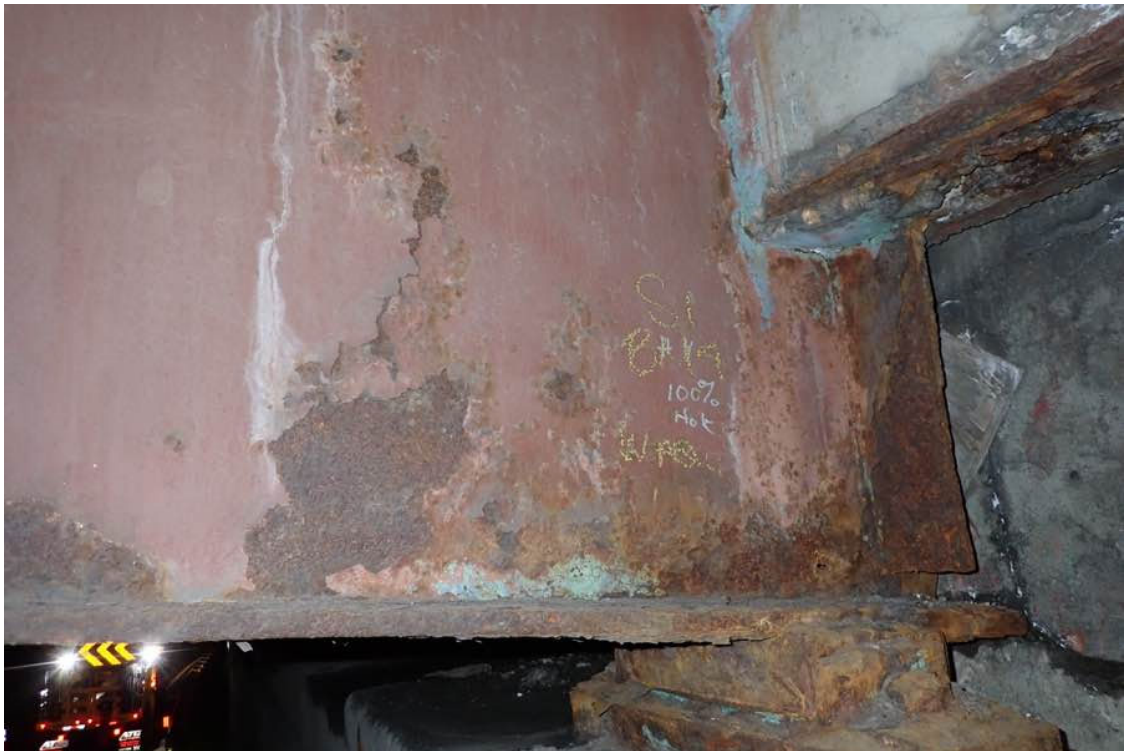
Photo 30: Beam 4 at the west end.
