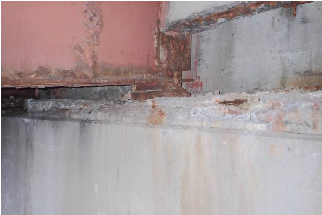
Photo 49: East bridge seat under bays #1 and #2.
