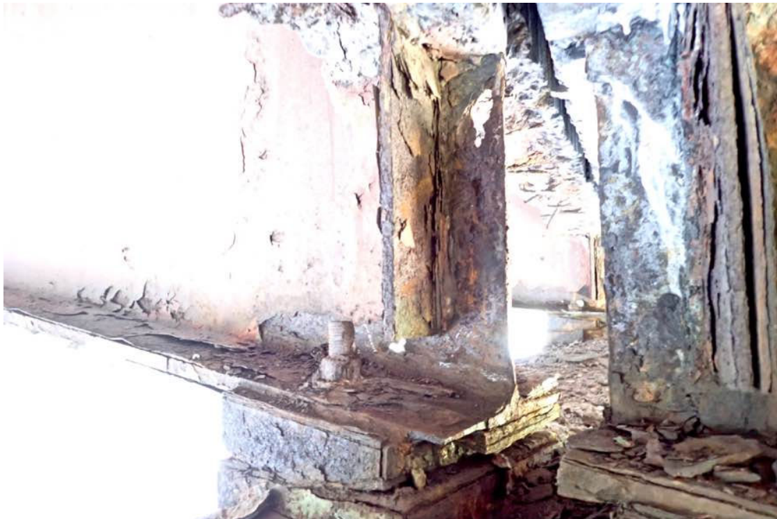
Photo 40: Beam S10 at the pier.
