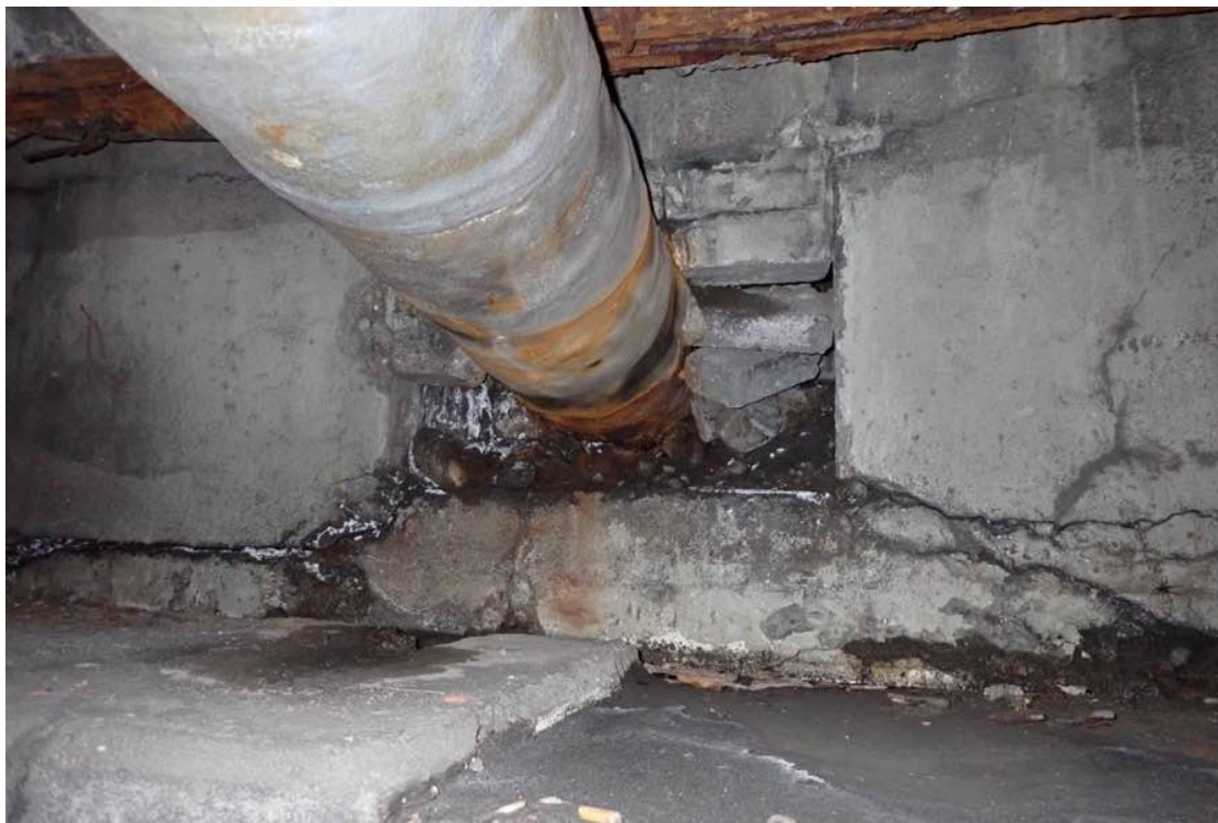
Photo 45: Bay 2 west abutment.
