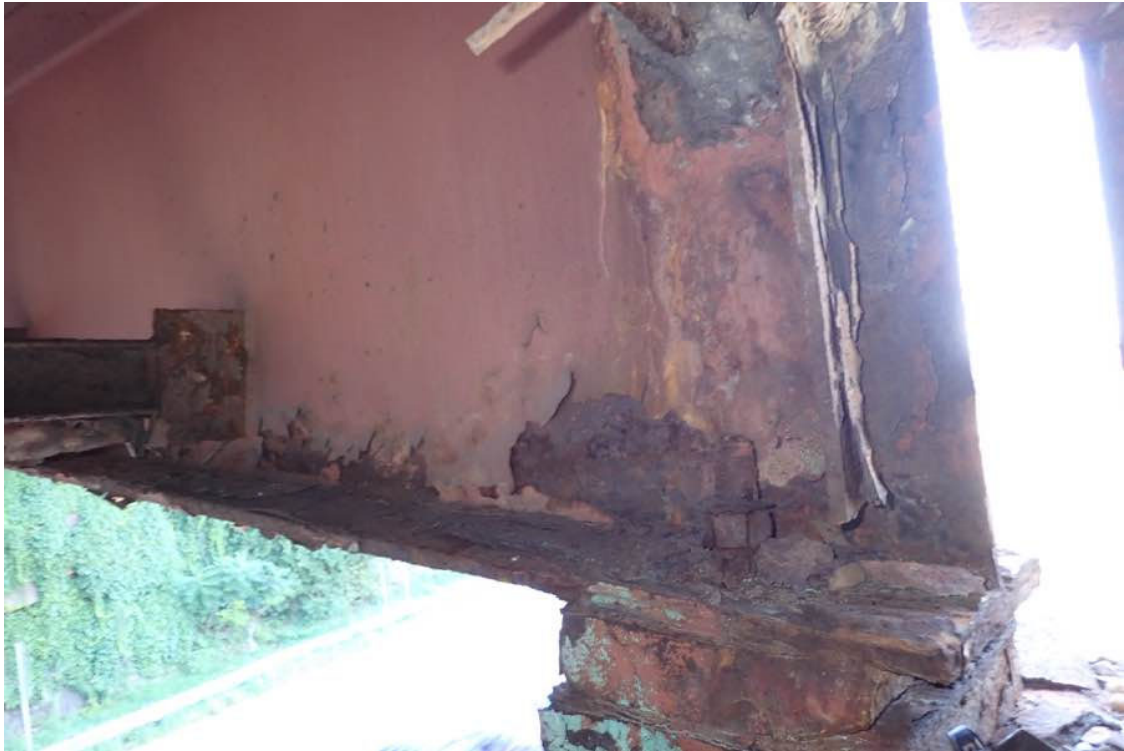
Photo 37: Beam S12 at the pier.
