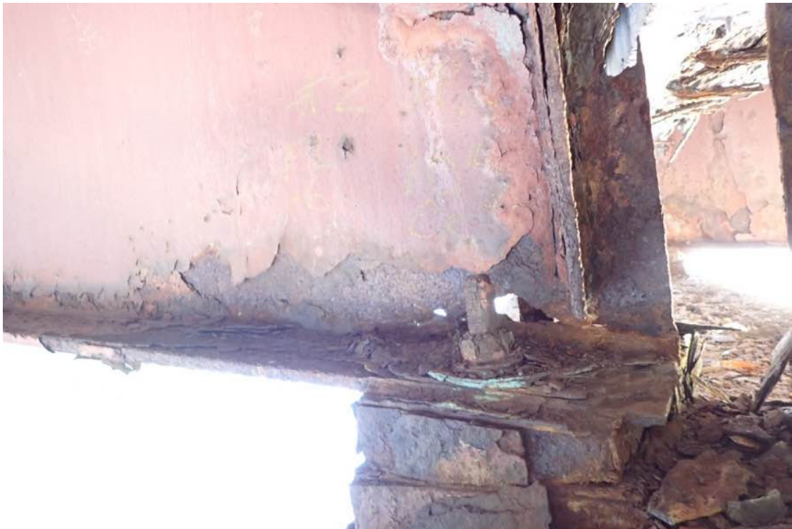
Photo 38: Beam S11 at the pier.
