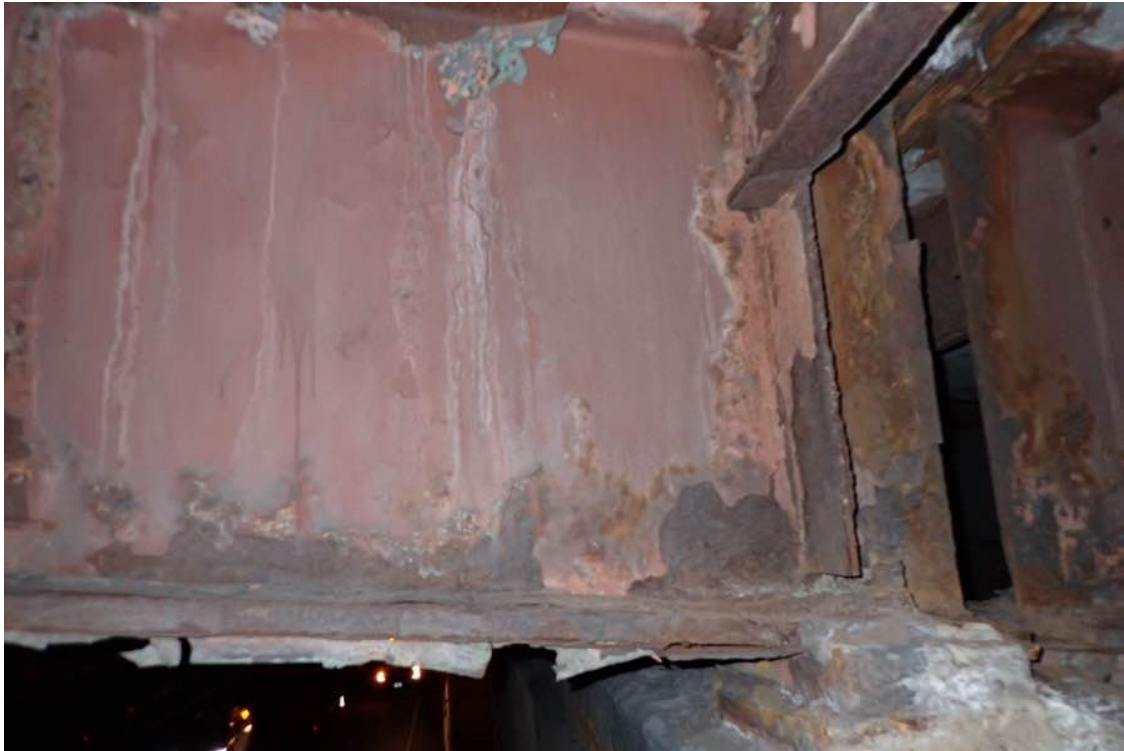
Photo 41: Beam 12 at the pier.
