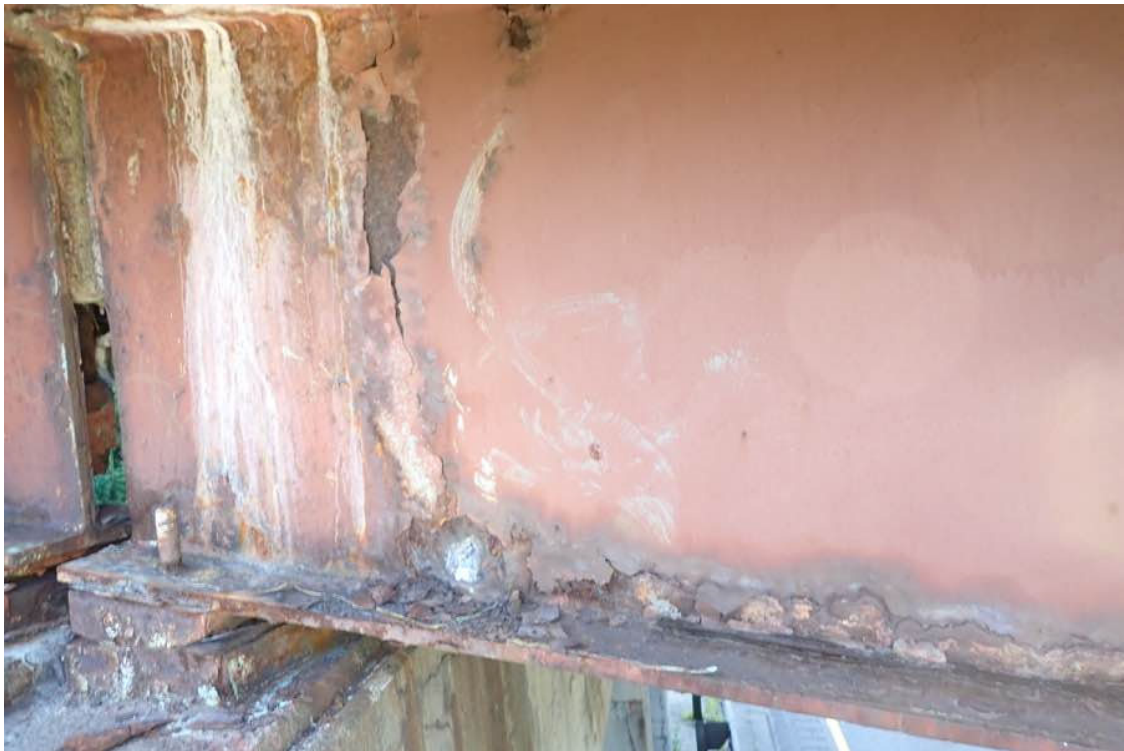
Photo 36: Beam S1 at the pier.
