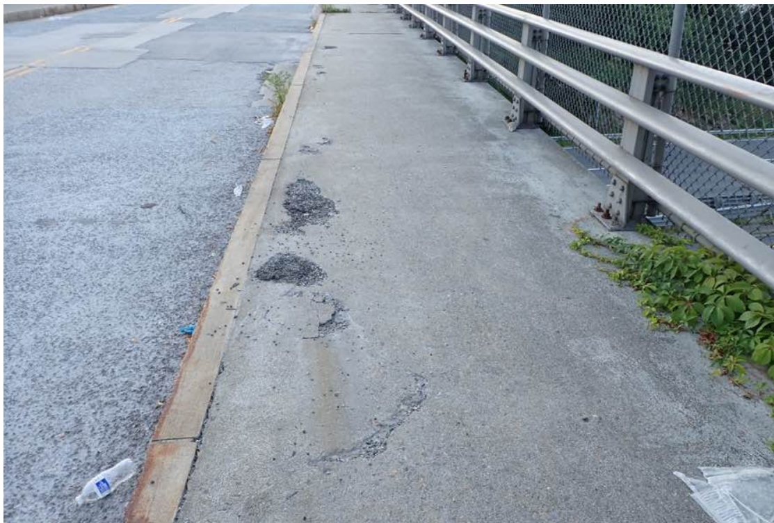
Photo 17: South sidewalk in span 1.
