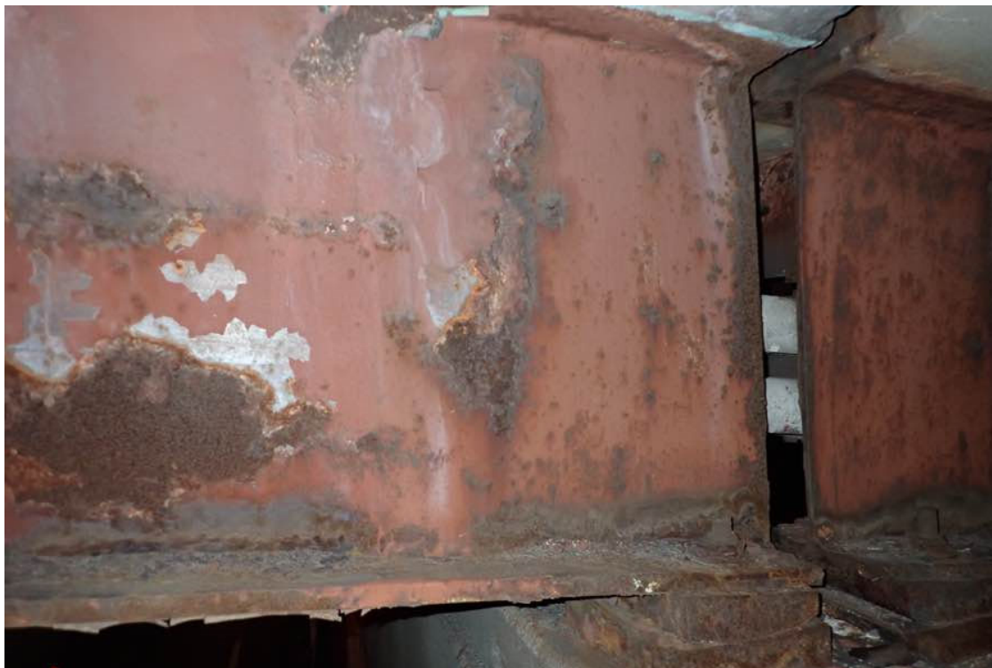
Photo 39: Beam 8 at the pier.
