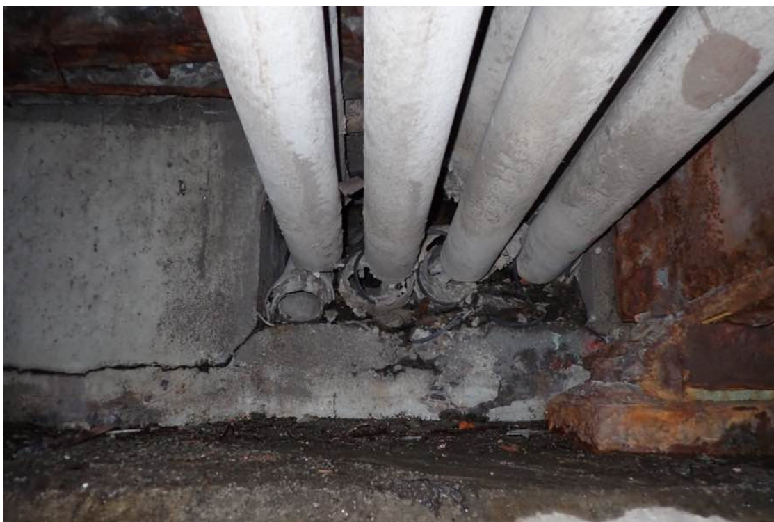
Photo 12: Utility conduit bank in bay 1 at the west abutment.
