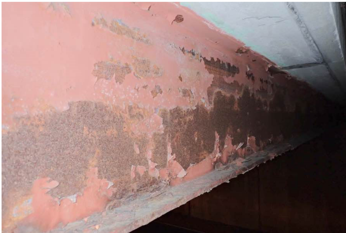
Photo 23: Beam 14 in span 2 looking east.
