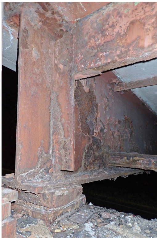
Photo 34: Beam 7 at the east end.
