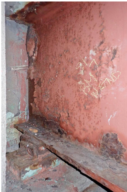
Photo 38: Beam 8 at the east abutment.
