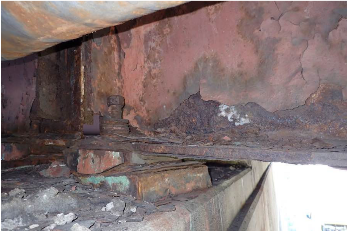
Photo 35: Beam S2 at the pier.
