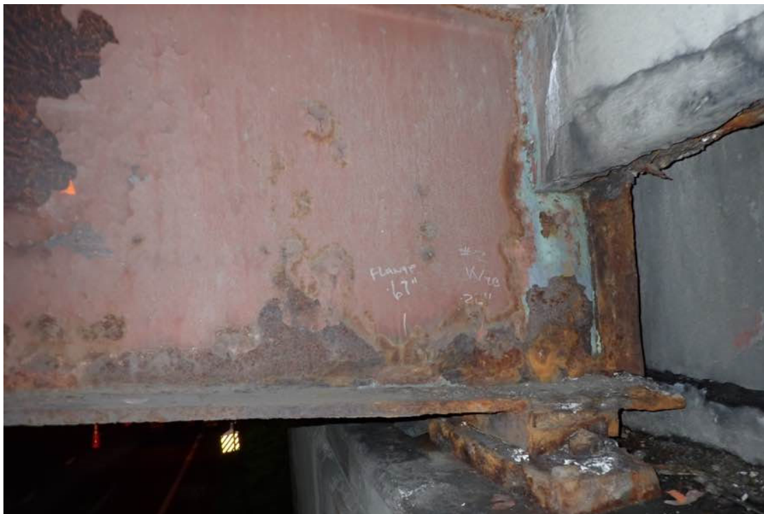
Photo 33: Beam 6 at the west end.
