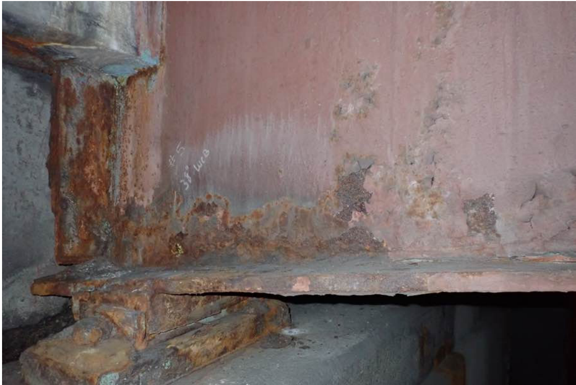
Photo 29: Beam 3 at the west end.
