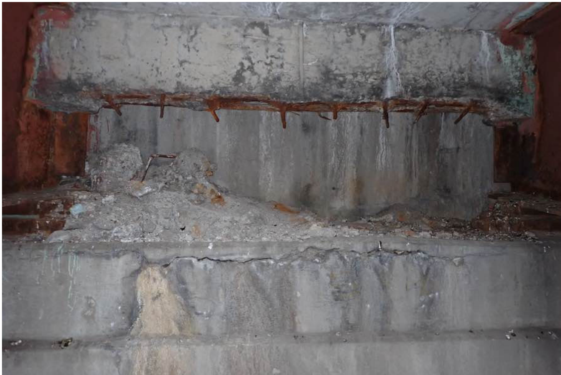
Photo 48: East bridge seat under bay #5.
