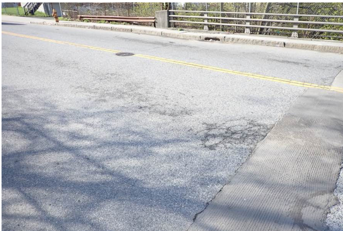
Photo 18: East approach pavement.
