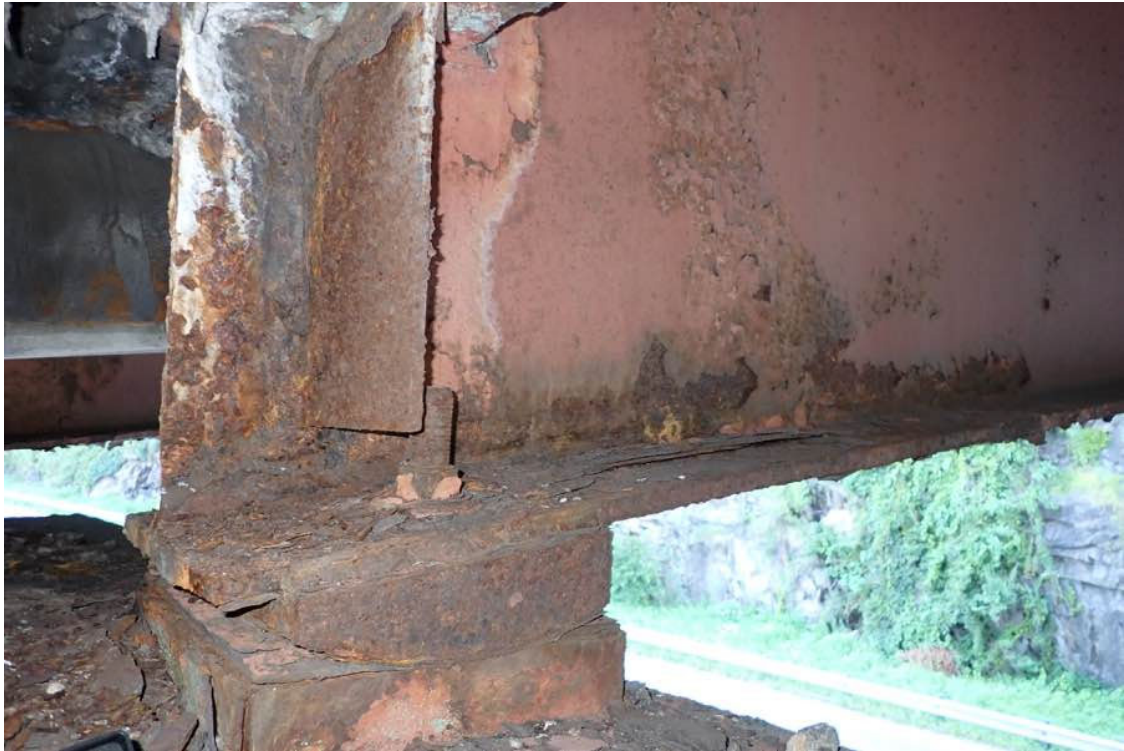
Photo 43: Beam S8 at the pier.
