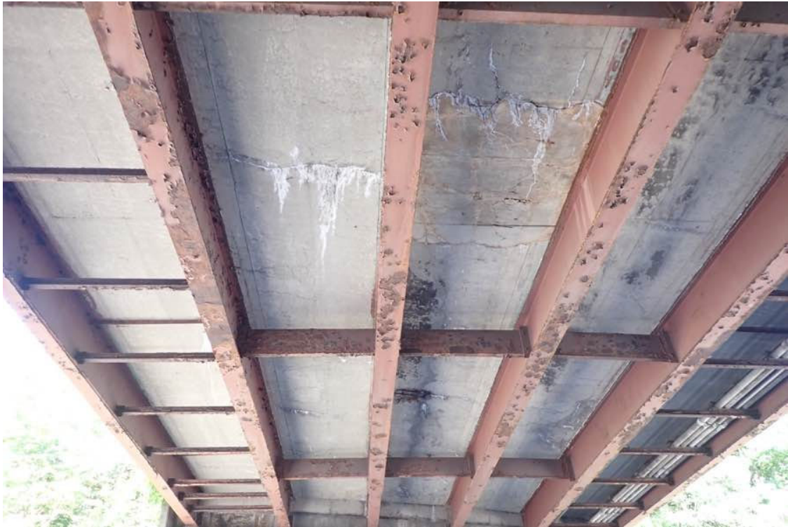
Photo 7: Deck underside in span 1.
