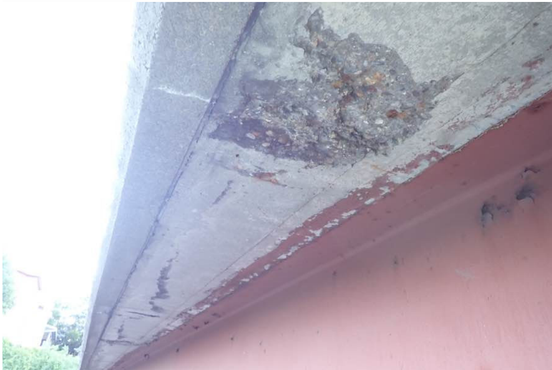
Photo 13: North deck fascia looking east from the ramp lane.
