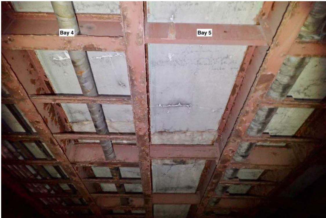
Photo 4: Deck underside in span 1 looking east.
