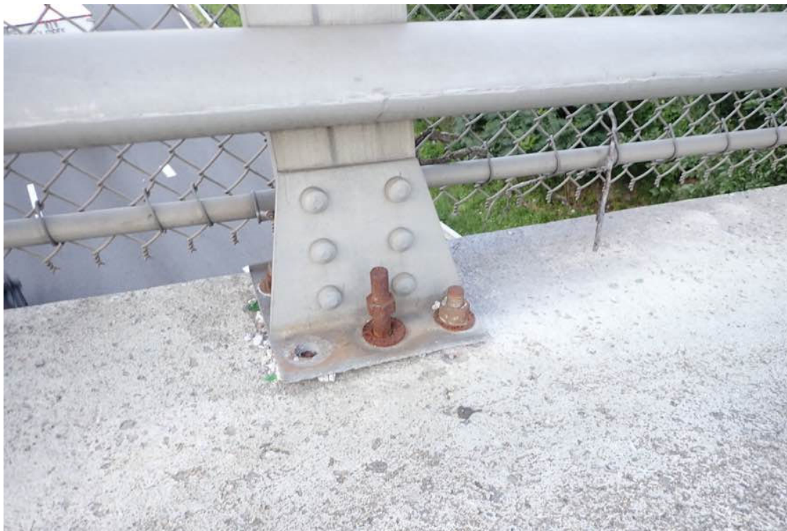
Photo 18: South railing at the 6th post from the west.
