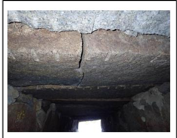
**Figure 3:** Crack in Granite Deck Slab (photo from MassDOT Routine & Member Inspection on May 13, 2021). 42.107038, -70.940290%
