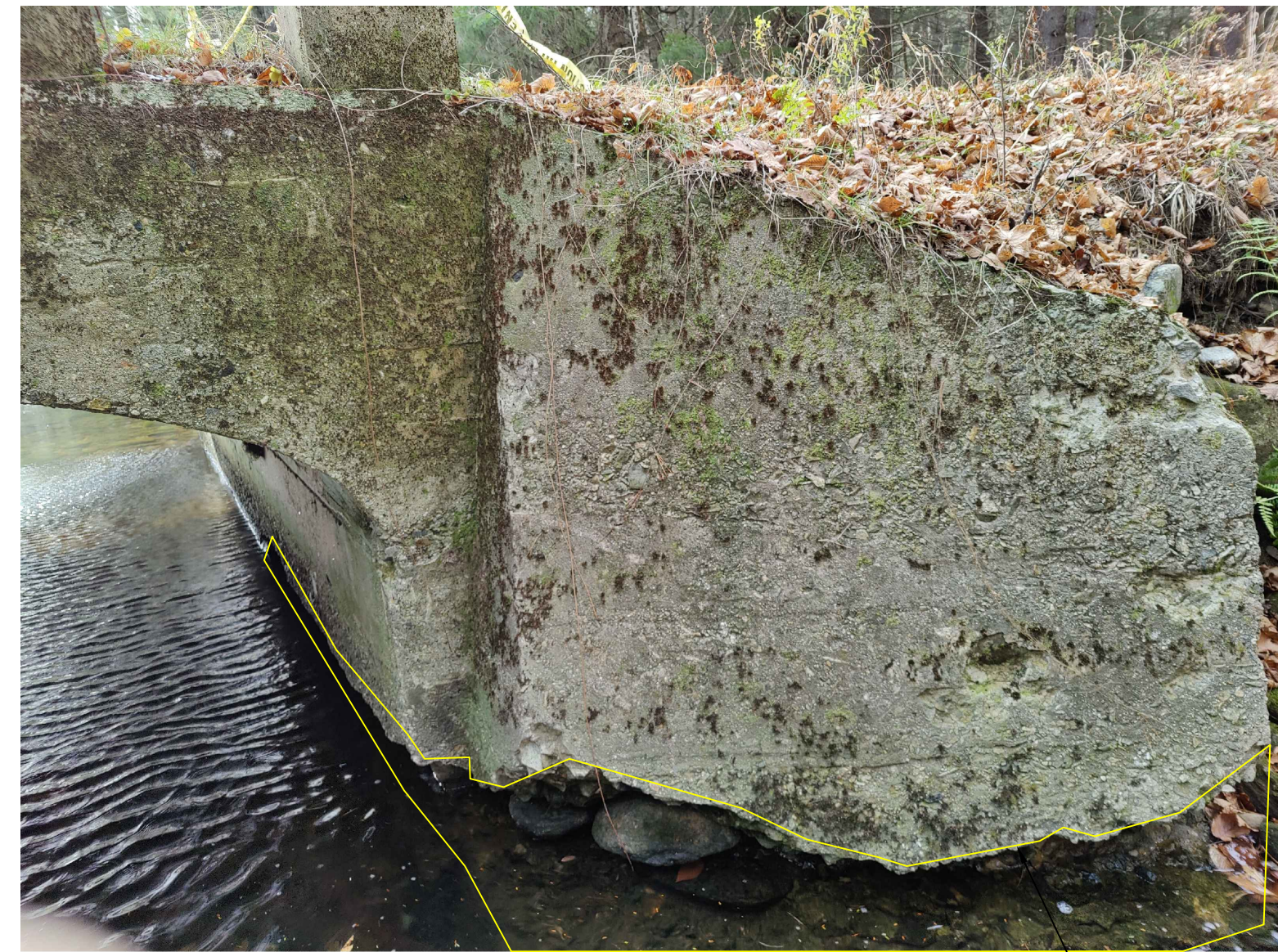
PHOTO 1 EXISTING NORTHWEST WINGWALL
