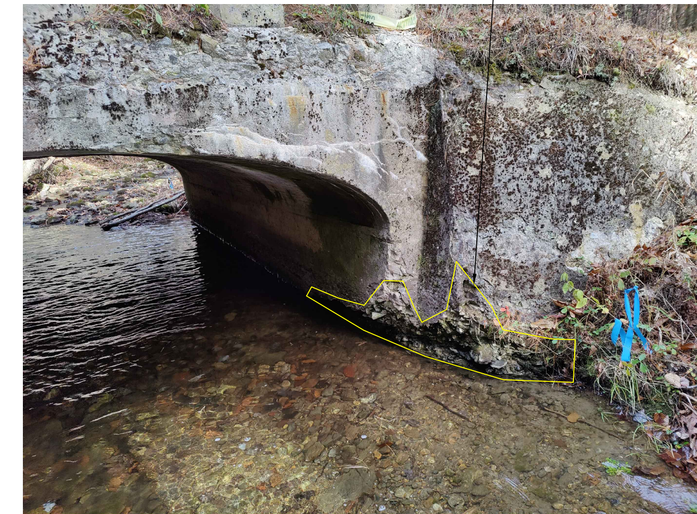
PHOTO 3 EXISTING SOUTHEAST WINGWALL
