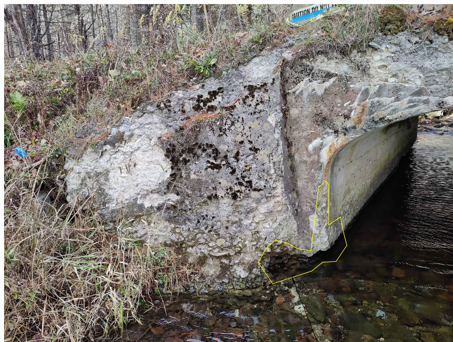
PHOTO 2 EXISTING SOUTHWEST WINGWALL
