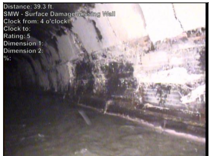
Photo: 797-796-20230503-083917-084514.JPG At: 39.33 ft. 4/. SMW - Surface Damage Missing Wall Joint: No
