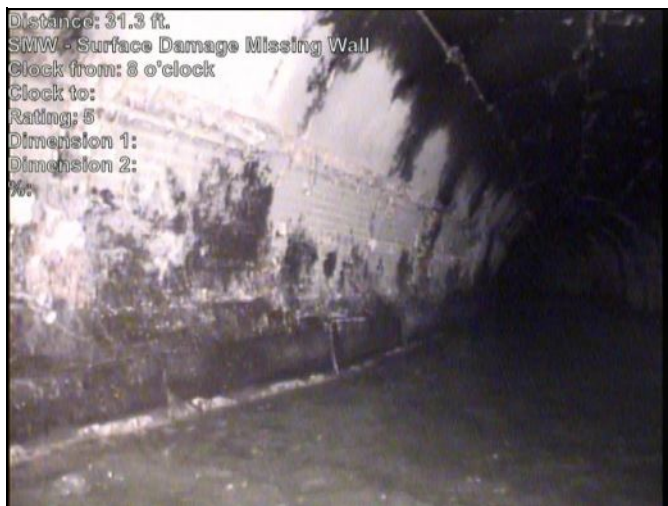
Photo: 797-796-20230503-083917-084450.JPG At: 31.324 ft. 8/. SMW - Surface Damage Missing Wall Joint: No
