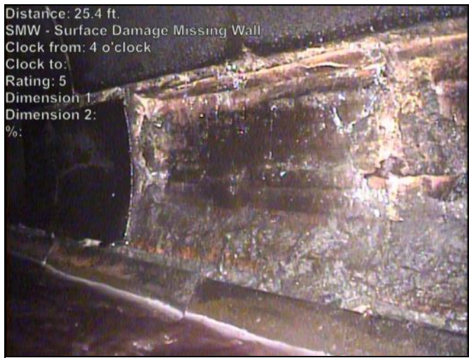
Photo: 791-J-8102-20230503-125257-125557.JPG At: 25.419 ft. 4/. SMW - Surface Damage Missing Wall Joint: No
