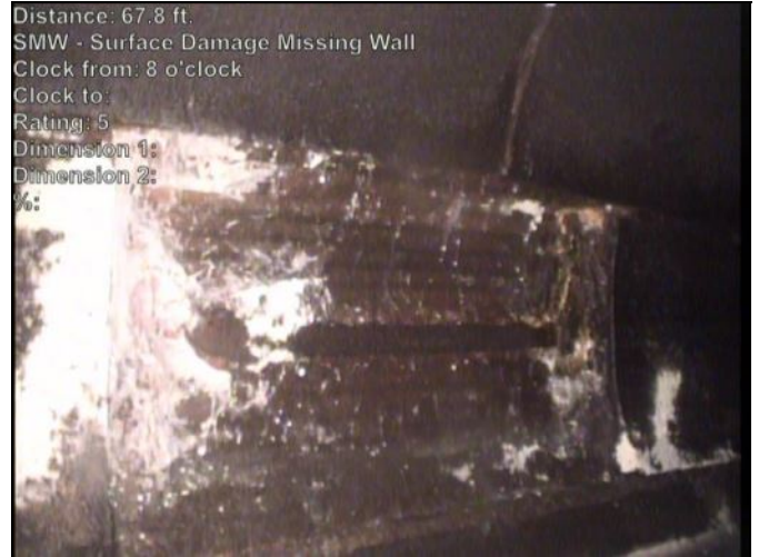
Photo: 796-795-20230503-090644-091234.JPG At: 67.752 ft. 8/. SMW - Surface Damage Missing Wall Joint: No
