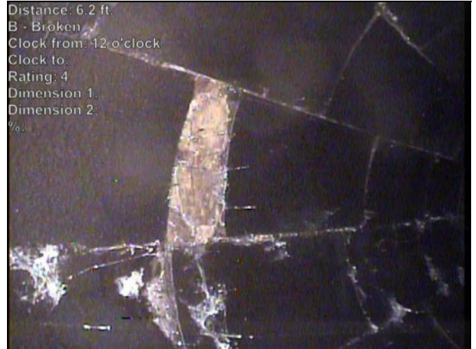
Photo: 7D8-7C1-20230503-133620-133708.JPG At: 6.205 ft. 12/. B - Broken Joint: No
