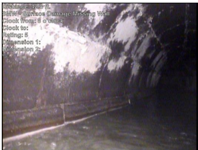
Photo: 797-796-20230503-083917-084530.JPG At: 42.833 ft. 8/. SMW - Surface Damage Missing Wall Joint: No
