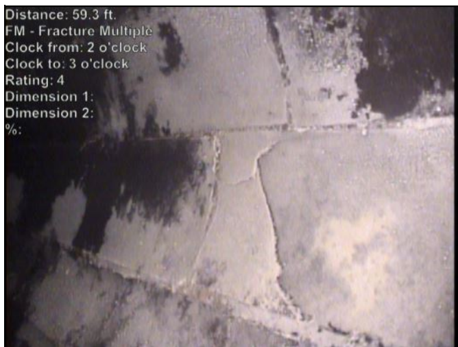
Photo: 797-796-20230503-083917-084644.JPG At: 59.345 ft. FM - Fracture Multiple 2/3 Joint: No
