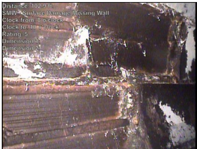
Photo: 791-J-8102-20230503-125257-130032.JPG At: 102.879 ft. SMW - Surface Damage Missing Wall 8/10 Joint: No
