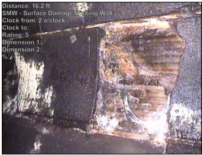
Photo: 791-J-8102-20230503-125257-125507.JPG At: 16.212 ft. 2/. SMW - Surface Damage Missing Wall Joint: No
