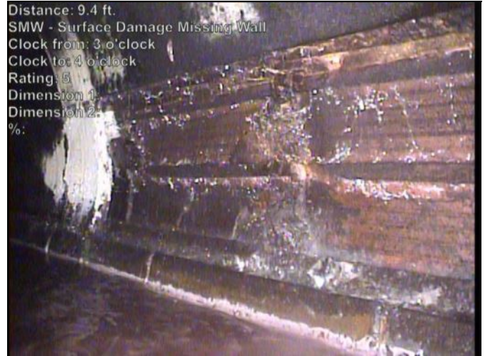
Photo: 791-J-8102-20230503-125257-125417.JPG At: 9.407 ft. 3/4 SMW - Surface Damage Missing Wall Joint: No
