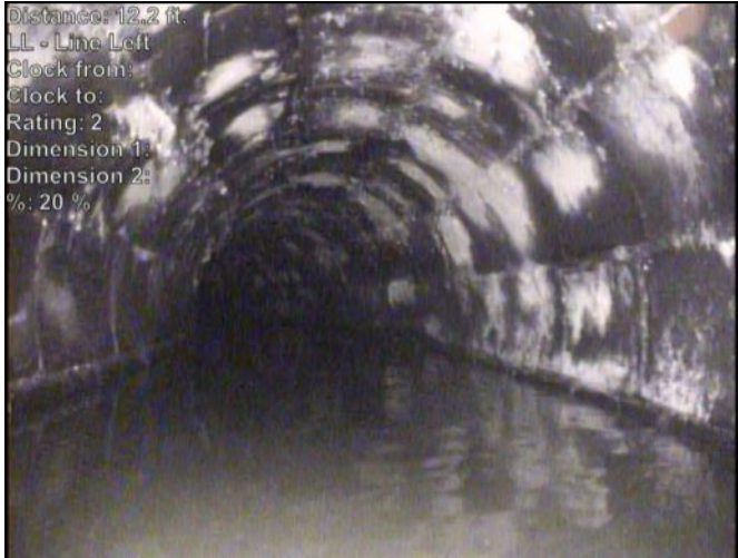
Photo: 798-797-20230503-081307-082744.JPG At: 12.209 ft. LL - Line Left Joint: No 20 %
