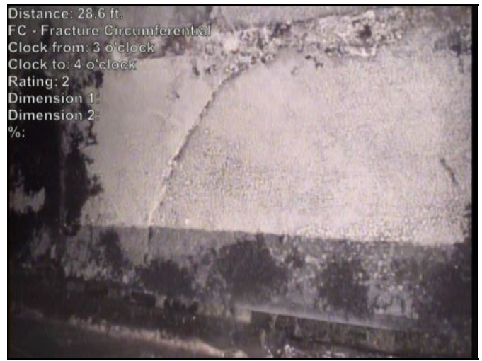
Photo: 797-796-20230503-083917-084429.JPG At: 28.622 ft. FC - Fracture Circumferential 3/4 Joint: No
