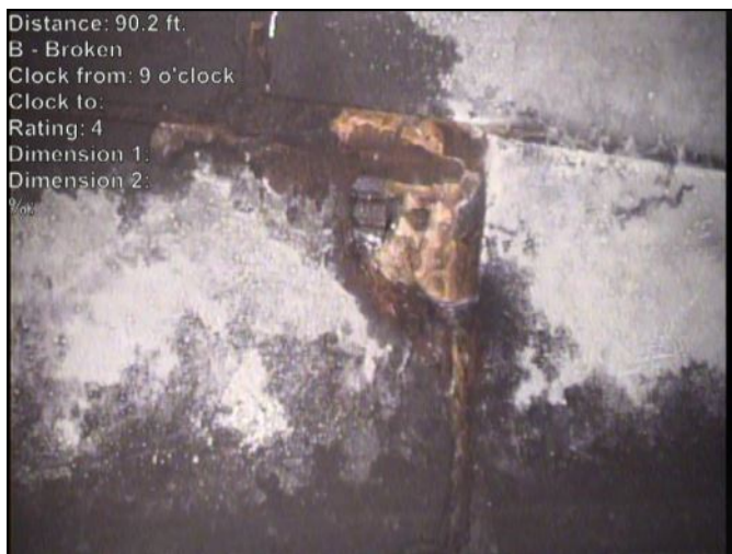
Photo: 797-796-20230503-083917-084937.JPG At: 90.169 ft. 9/. B - Broken Joint: No
