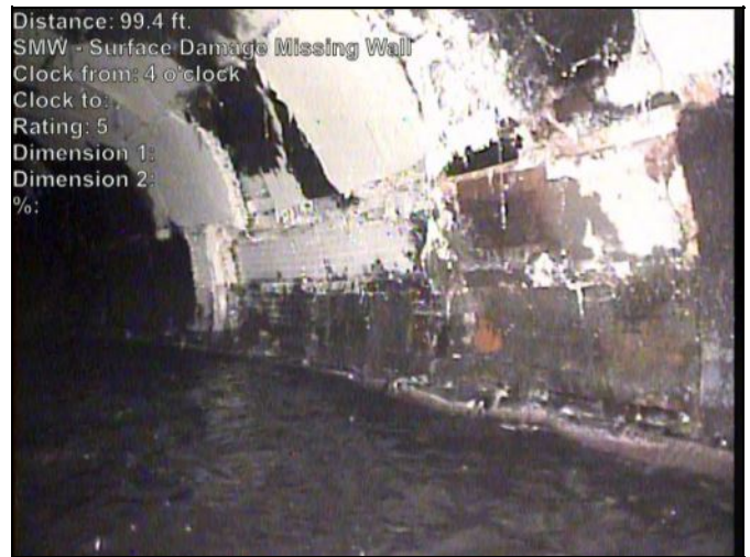
Photo: 791-J-8102-20230503-125257-130015.JPG At: 99.376 ft. 4/. SMW - Surface Damage Missing Wall Joint: No
