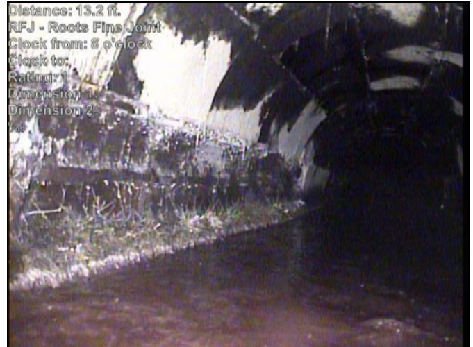
Photo: 791-J-8102-20230503-125257-125451.JPG At: 13.21 ft. 8/. RFJ - Roots Fine Joint Joint: Yes
