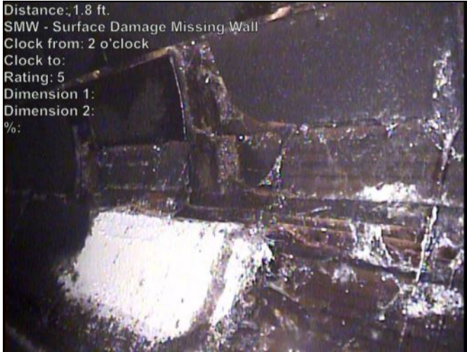
Photo: 791-J-8102-20230503-125257-125347.JPG At: 1.801 ft. 2/. SMW - Surface Damage Missing Wall Joint: No
