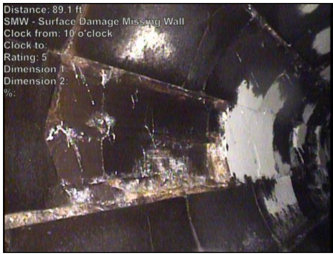
Photo: 791-J-8102-20230503-125257-125929.JPG At: 89.068 ft. SMW - Surface Damage Missing Wall 10/. Joint: No
