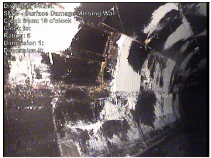
Photo: 791-J-8102-20230503-125257-125949.JPG At: 94.673 ft. SMW - Surface Damage Missing Wall 10/. Joint: No
