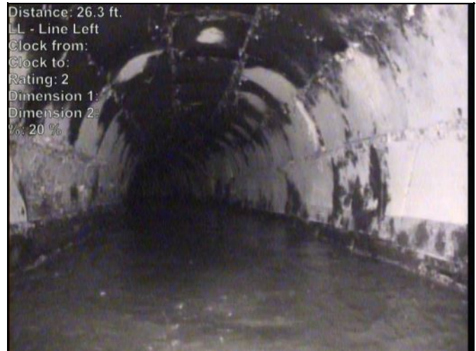
Photo: 797-796-20230503-083917-084409.JPG At: 26.32 ft. LL - Line Left Joint: No 20 %
