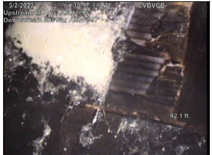
Photo: 798-797-20230502-103631-104706.JPG At: 87.367 ft. FM - Fracture Multiple 10/11 Joint: No
