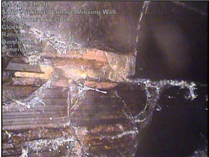
Photo: 7D8-7C1-20230503-133620-133648.JPG At: 4.503 ft. 12/. SMW - Surface Damage Missing Wall Joint: No
