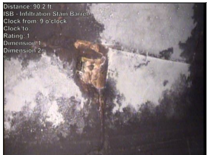
Photo: 797-796-20230503-083917-084916.JPG At: 90.169 ft. 9/. ISB - Infiltration Stain Barrel Joint: No
