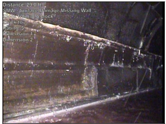
Photo: 791-J-8102-20230503-125257-125613.JPG At: 29.022 ft. 8/. SMW - Surface Damage Missing Wall Joint: No
