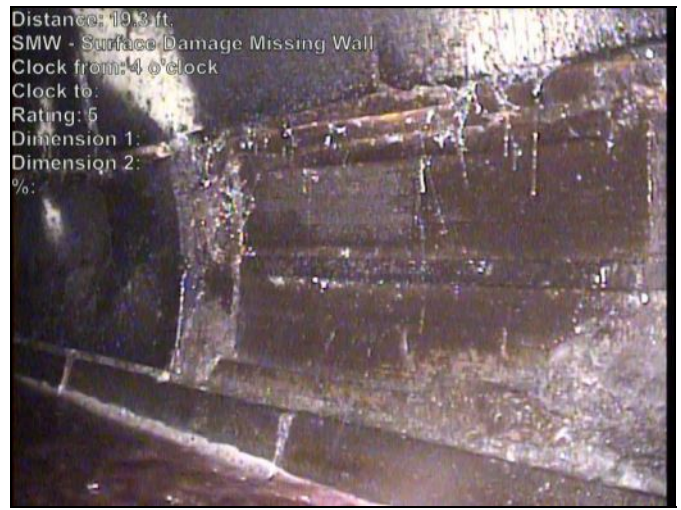
Photo: 791-J-8102-20230503-125257-125530.JPG At: 19.315 ft. 4/. SMW - Surface Damage Missing Wall Joint: No
