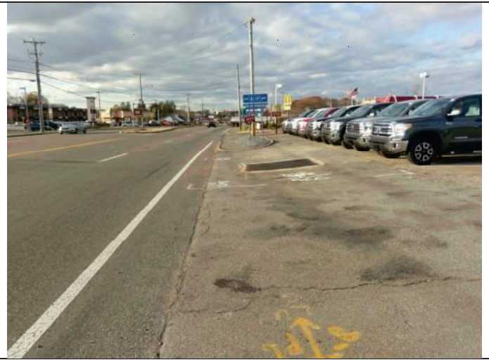
U.S. Route 6 looking westbound towards the intersection at Route 136
