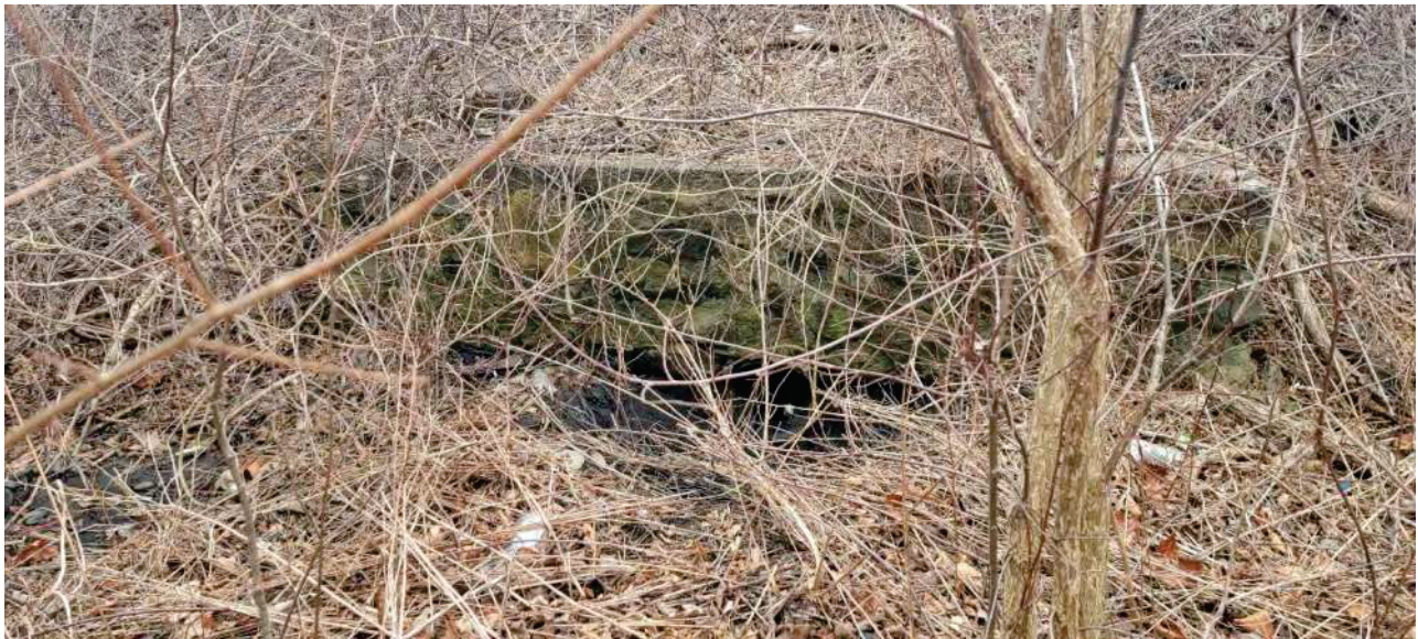
Photograph 4: Southeast view of culvert discharging stormwater towards the E-series BVW.
