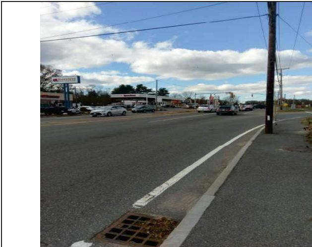
U.S. Route 6 looking eastbound towards the intersection at Route 118
