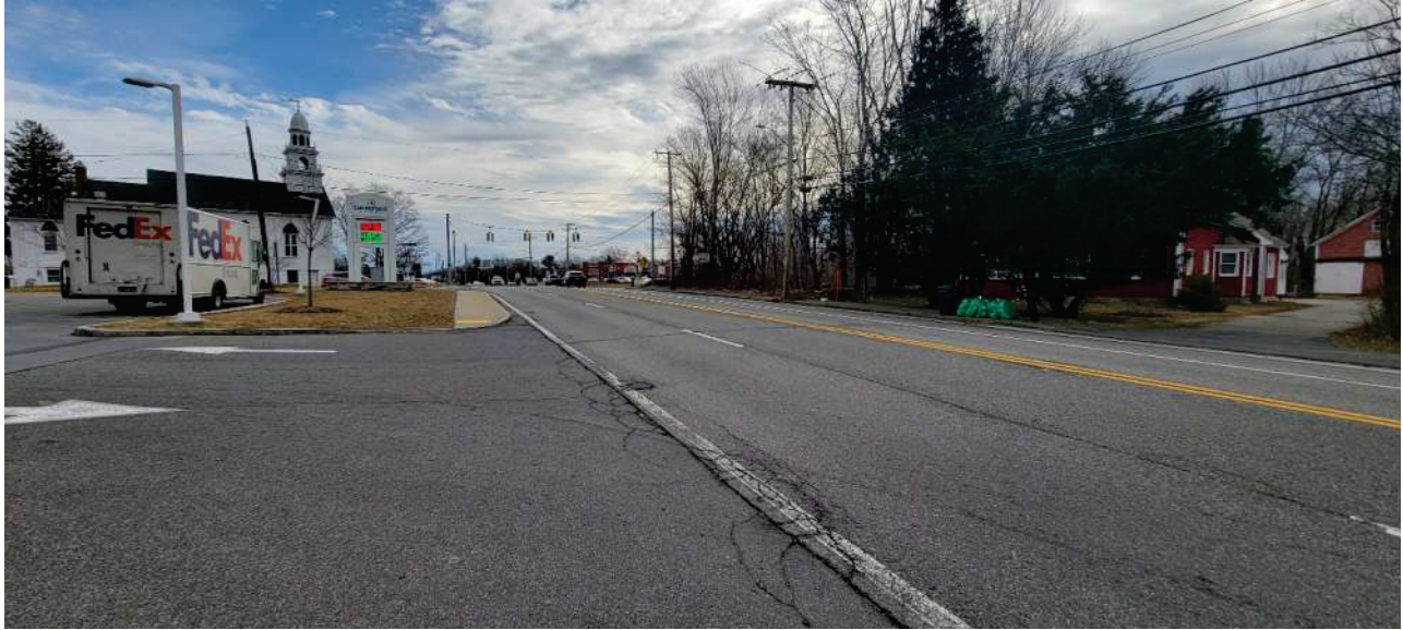
Photograph 1: East view of the Route 6 with Route 6/Maple Avenue intersection in background.
