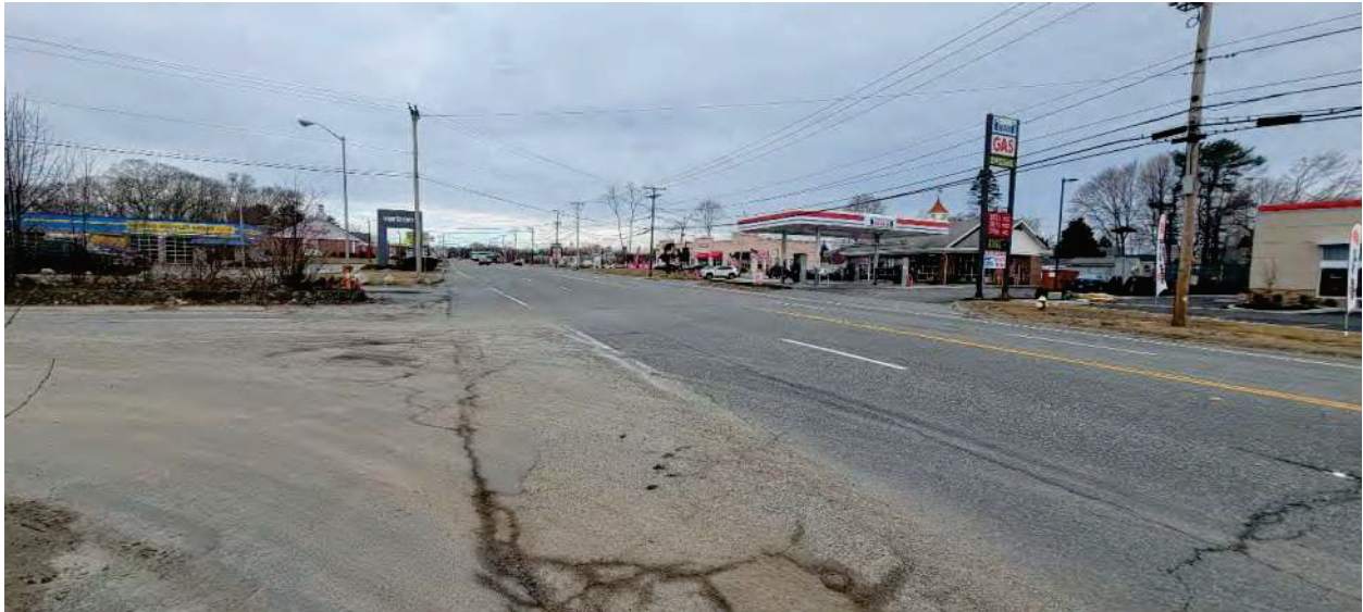
Photo 3: Northwest view of Route 6 from #711 Route 6 (eastern site limit).
