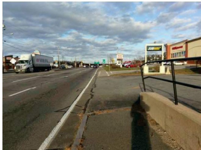
Route 136 looking northbound towards intersection at U.S. Route 6
