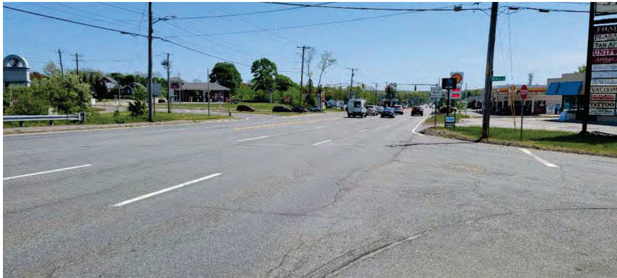
Photograph 1: East view of Route 6/Route 118 intersection (Route 118 to the left). Taken May 10, 2023.
