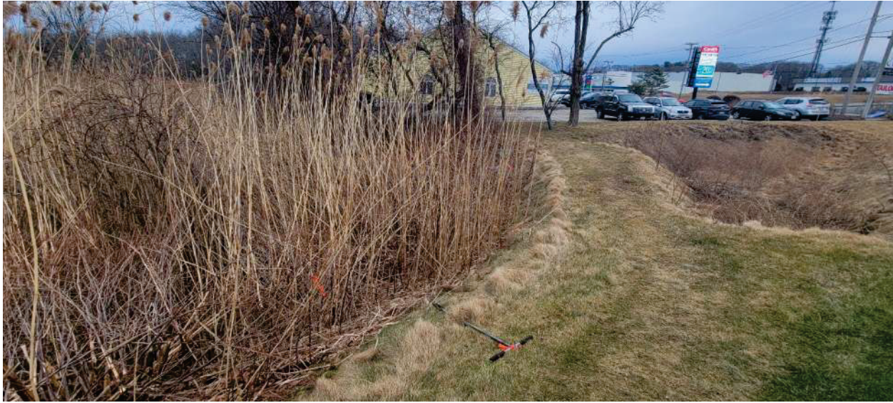
Photograph 7: Northwest view of D-series BVW (left), upland lawn area (center) and adjacent stormwater basin (right).
